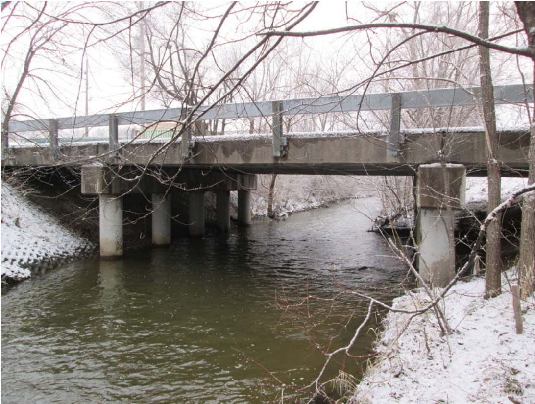
Photo No. 1 South Elevation of Structure, looking North
