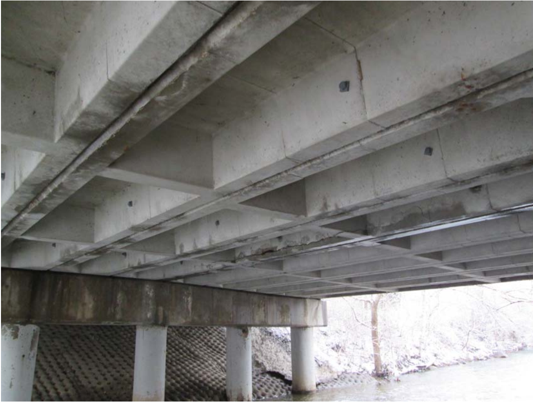
Photo No. 9 Underside of Center Span, looking Northwest
