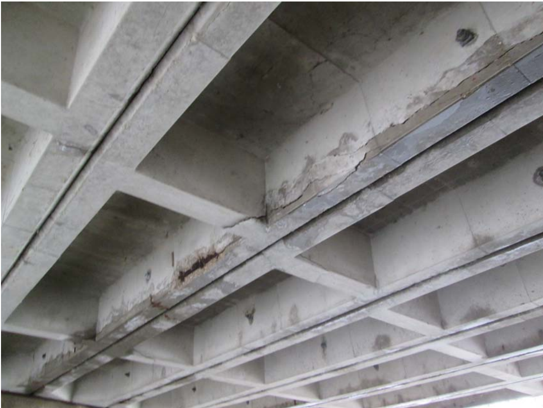
Photo No. 12 Joint Between Beams 5 and 6 in Center Span, looking Southeast
