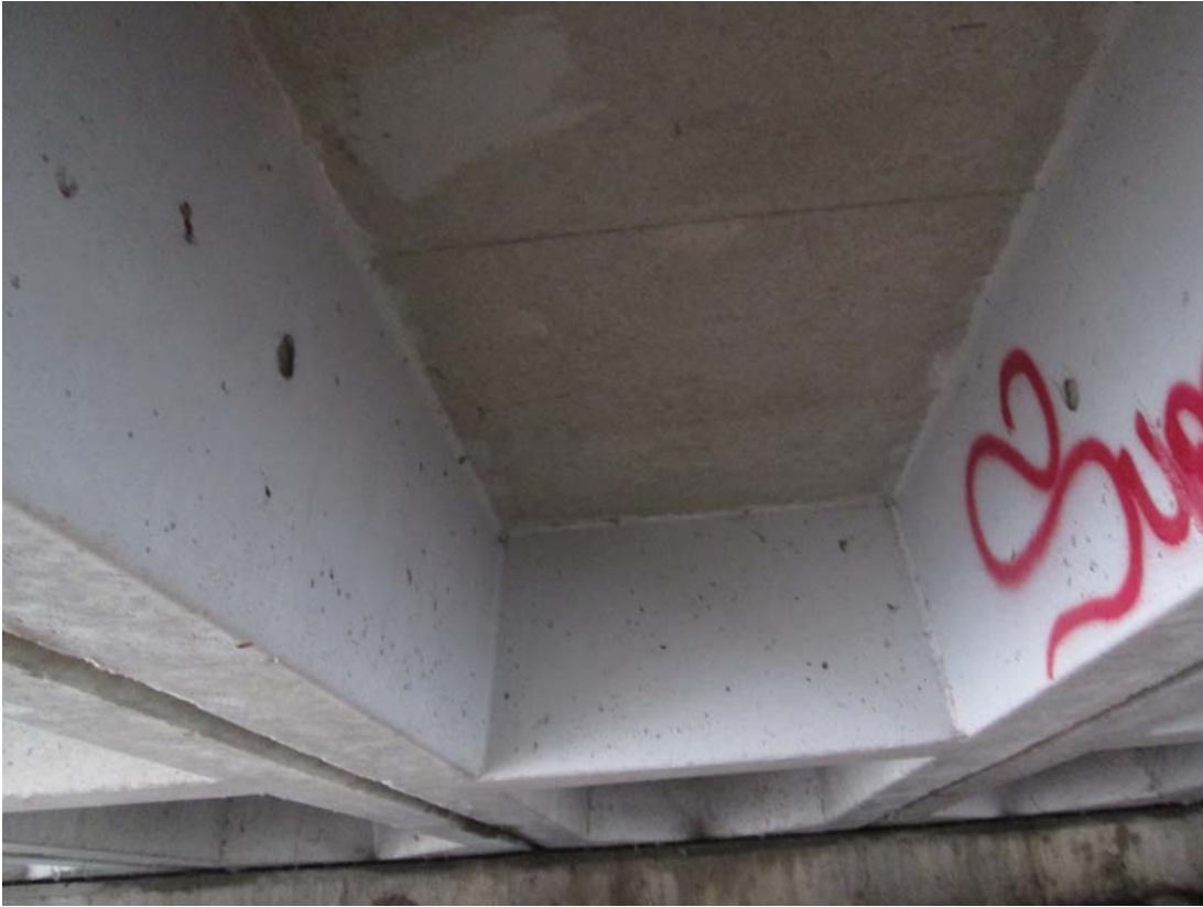
Photo No. 11 Typical Condition of Channel Beams in East Span, looking East
