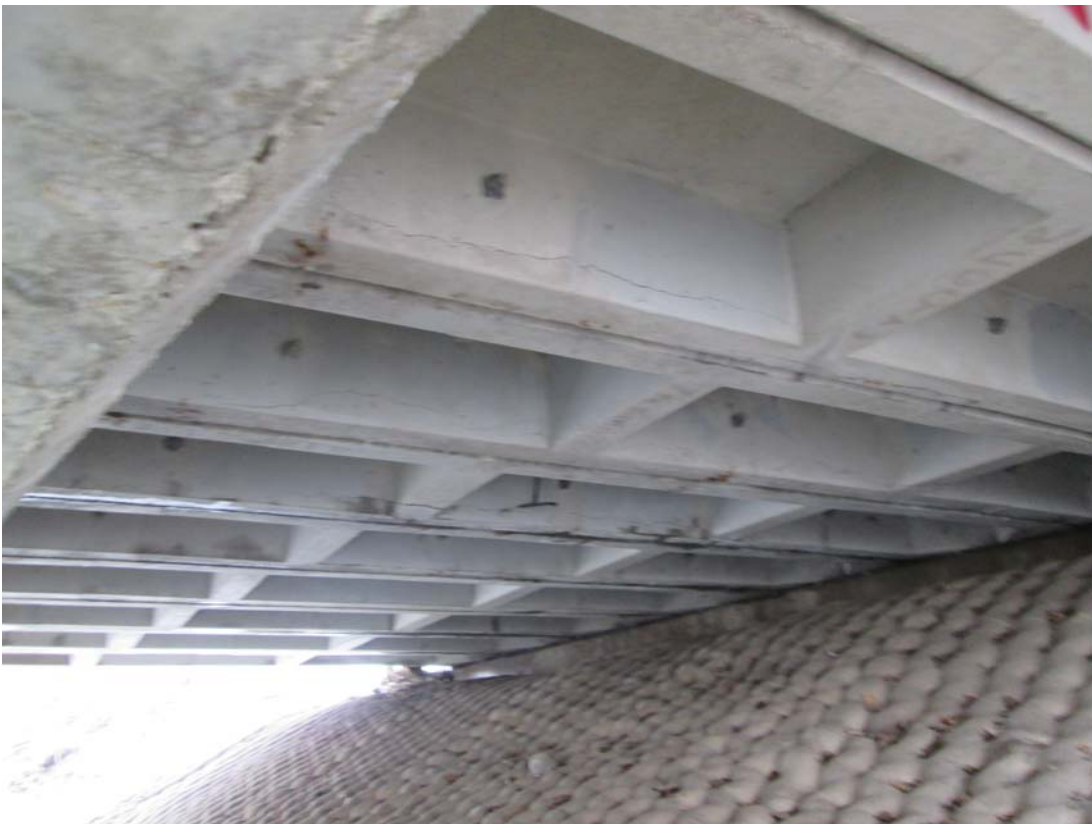
Photo No. 10 Underside of West Span, looking Southwest
