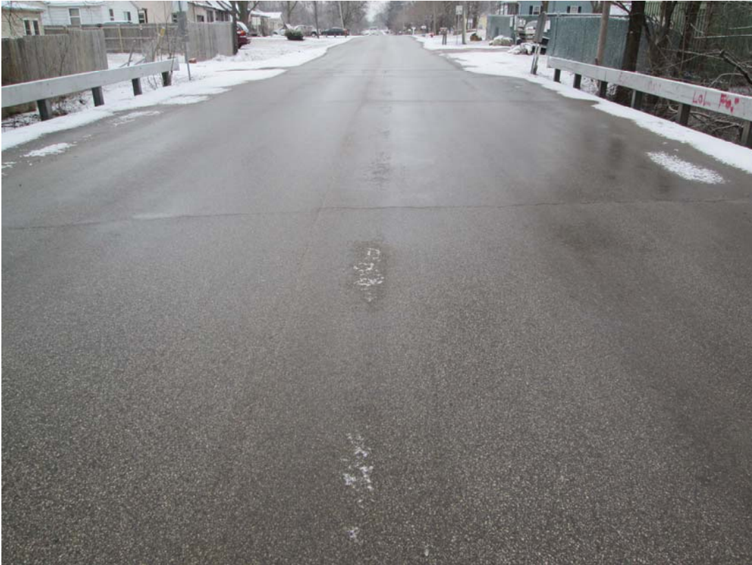
Photo No. 7 Typical Deck Condition, looking West
