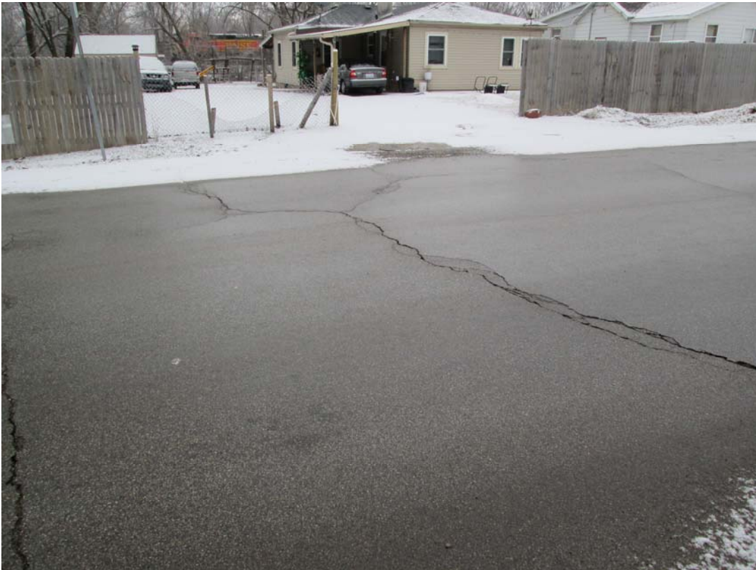
Photo No. 5 West Approach Roadway, looking Southwest
