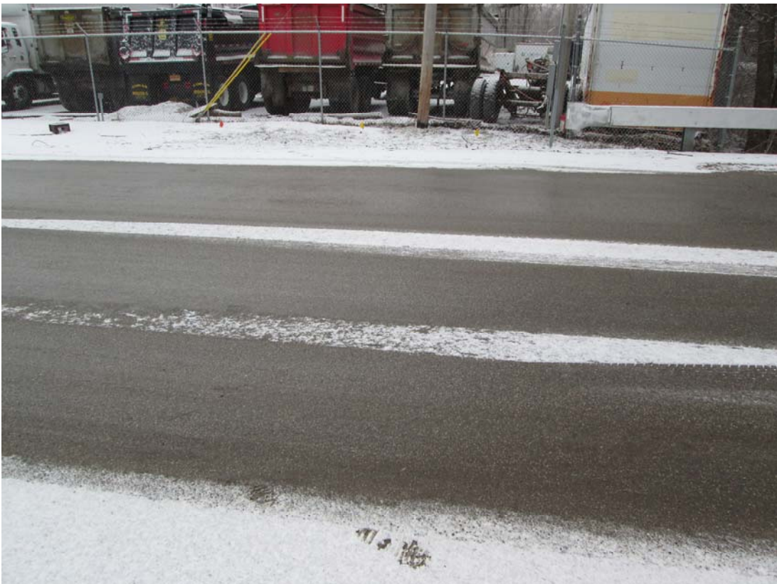
Photo No. 4 East Approach Roadway, looking South
