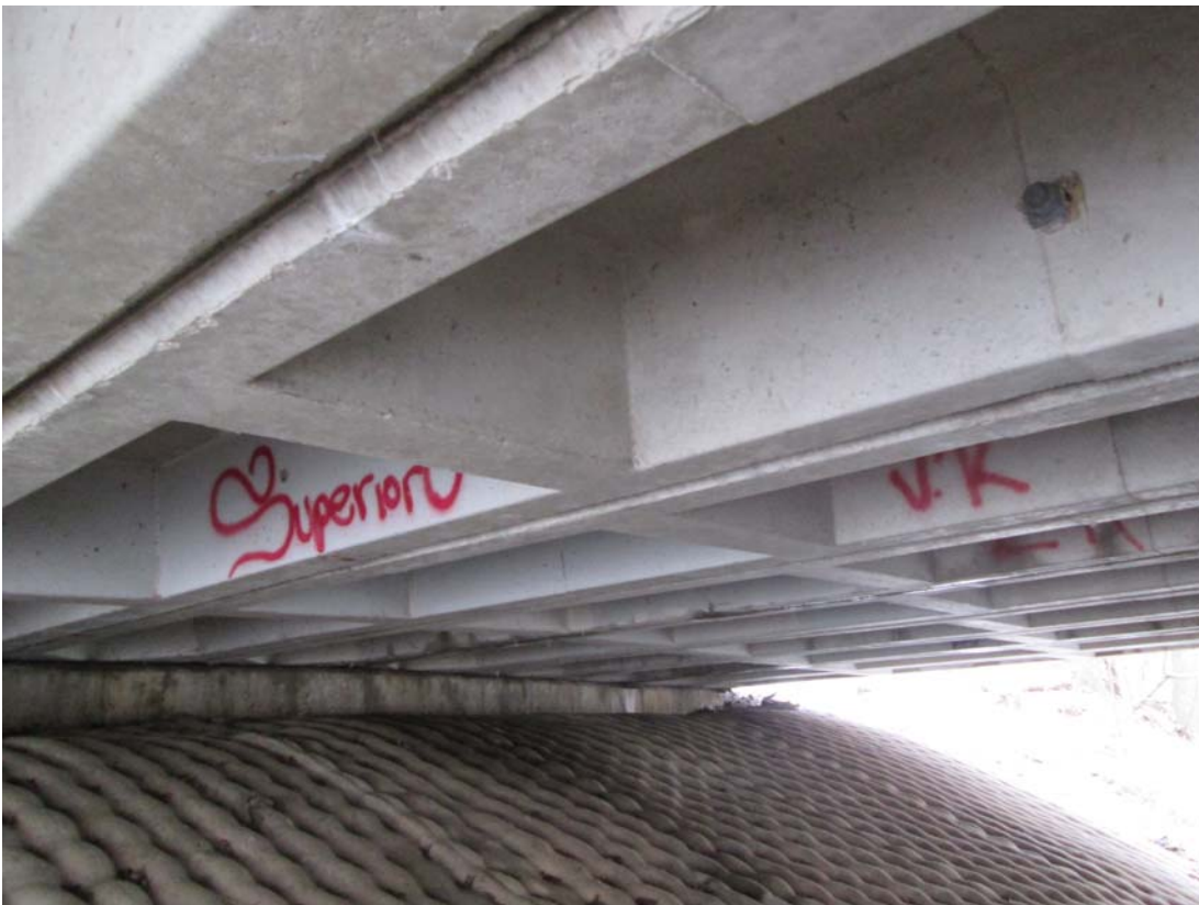
Photo No. 8 Underside of East Span, looking Southeast
