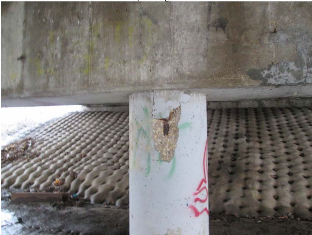
Photo No. 18 Typical Spall on Pier Pile Encasement (East Pier Middle Column Shown), looking East
