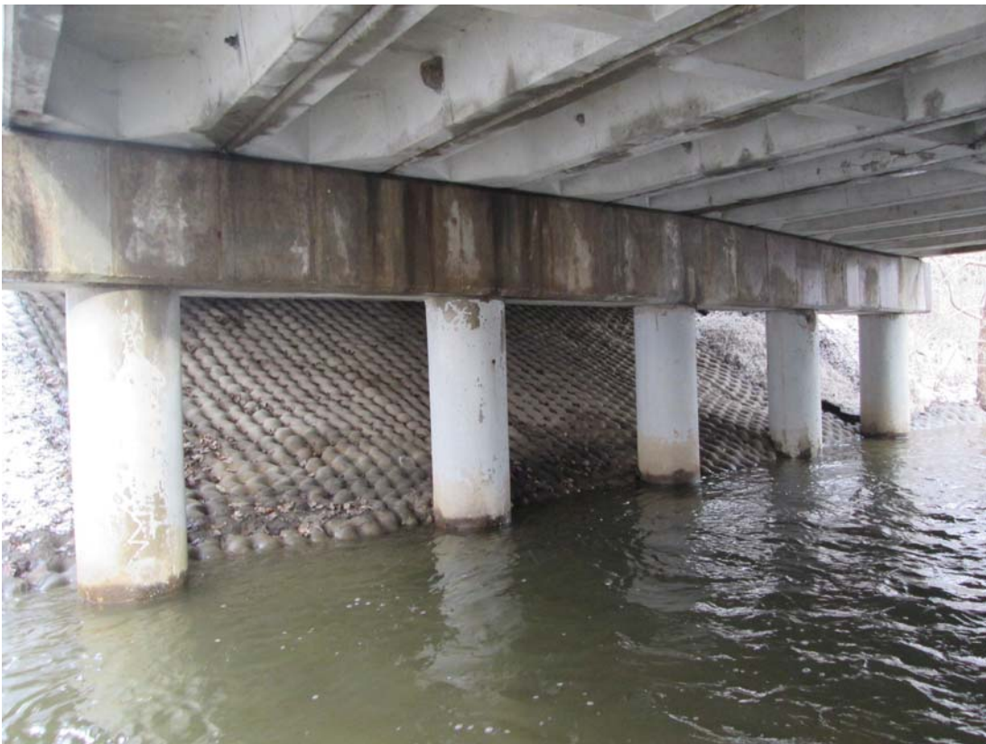
Photo No. 16 West Pier, looking Northwest
