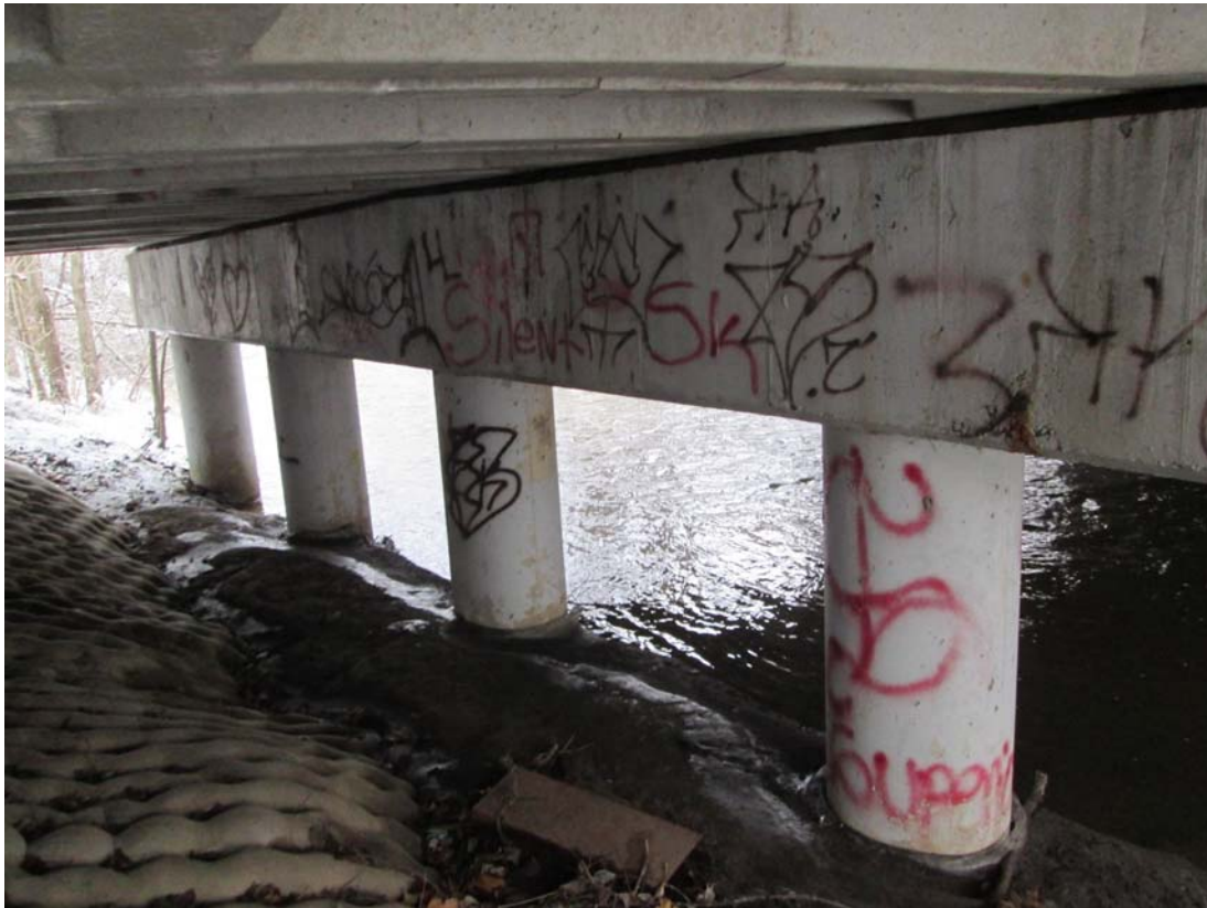
Photo No. 17 East Pier, looking Southwest
