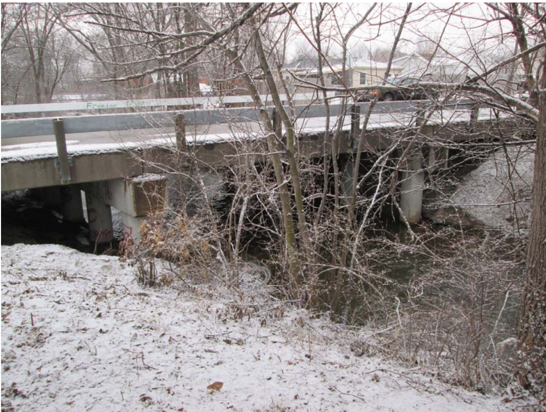
Photo No. 2 North Elevation of Structure, looking South
