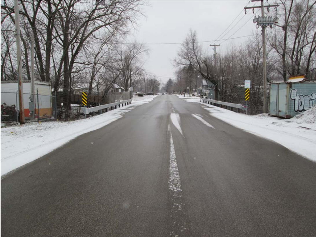
Photo No. 3 Approach Roadway and Structure, looking West
