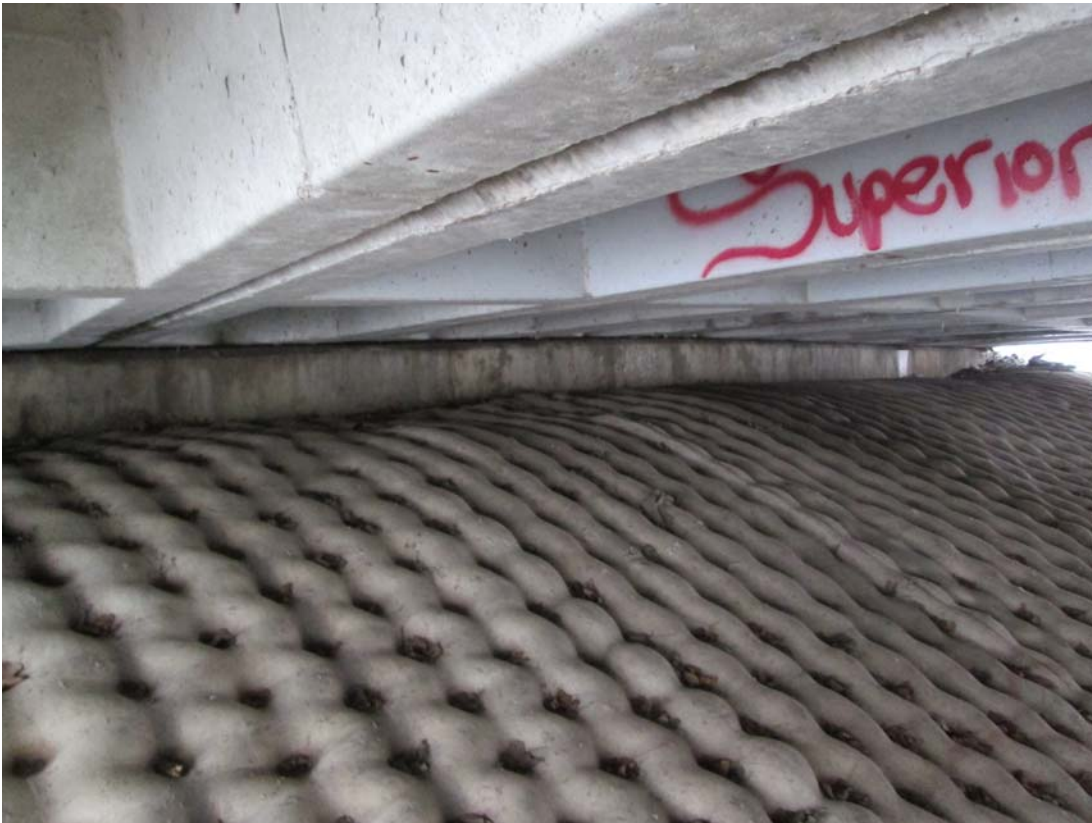
Photo No. 15 East Abutment Elevation, looking Southeast
