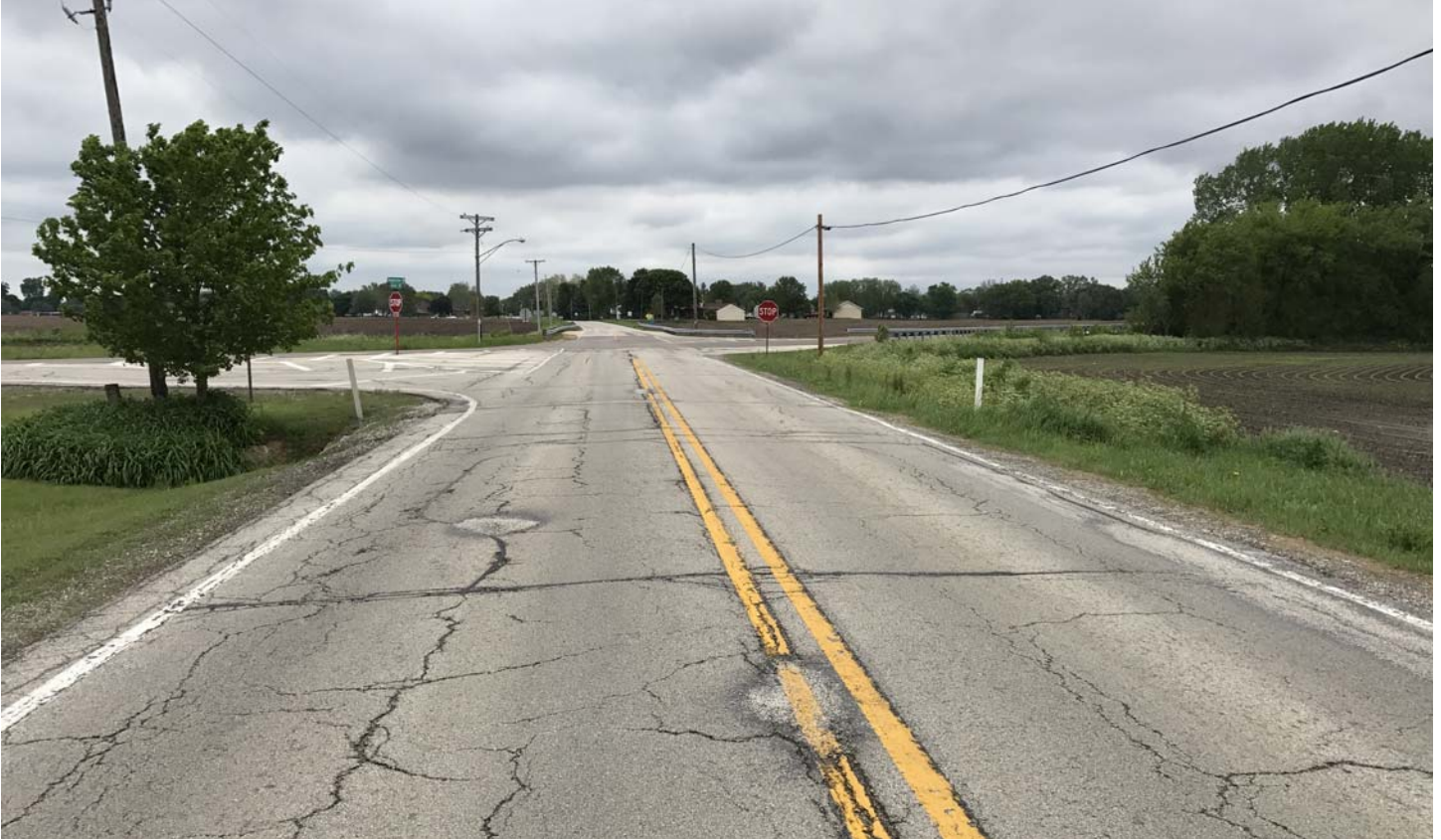
Photo 5 - Looking East along Harter Rd
