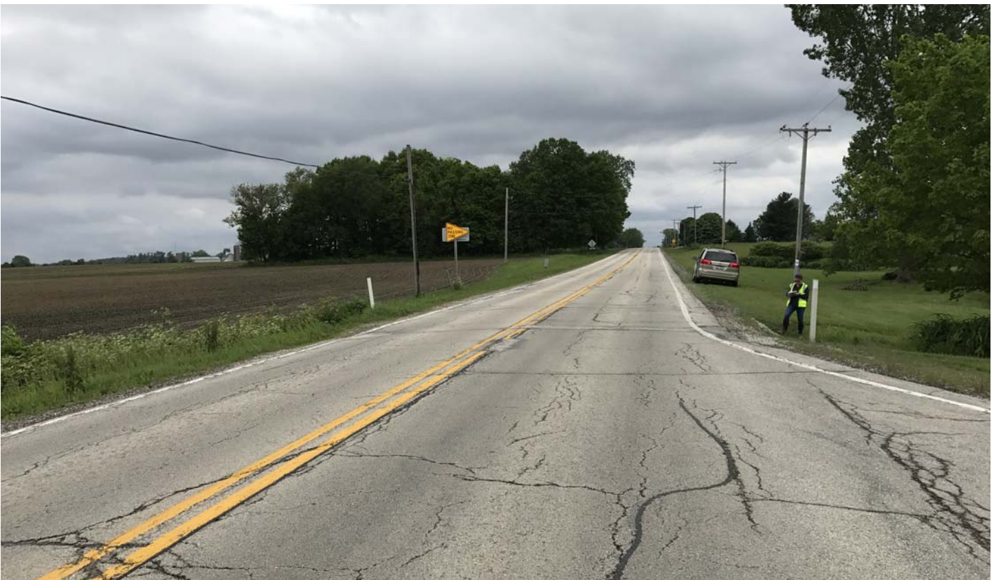
Photo 6 - Looking West along Harter Rd
