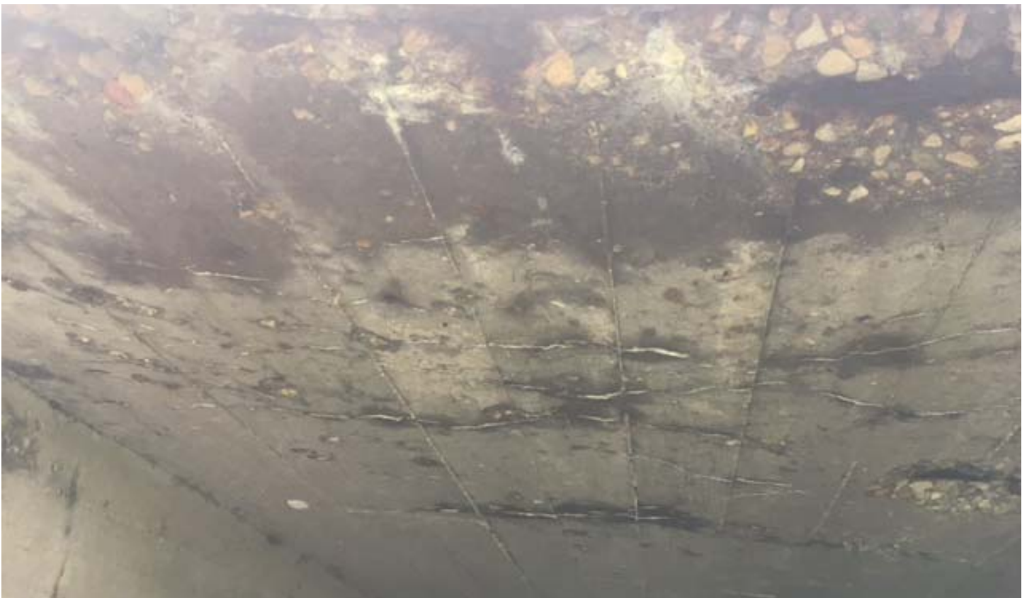
Photo 14 - Top Slab Map Cracking at North End
