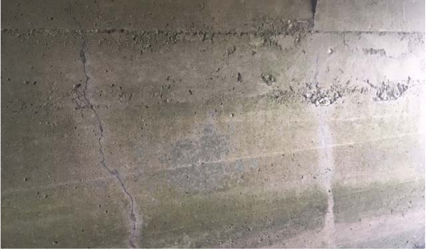
Photo 11 - West Wall North End Cracks
