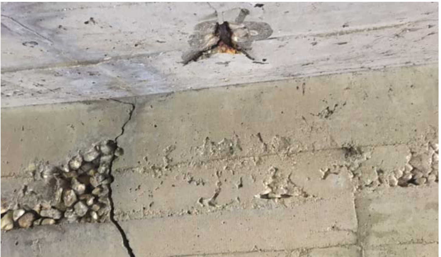
Photo 10 - Top Slab Spall near Mid Span Crack
