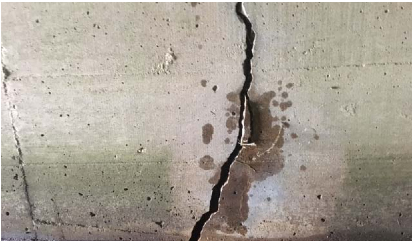
Photo 8 - East Wall Mid Span Crack
