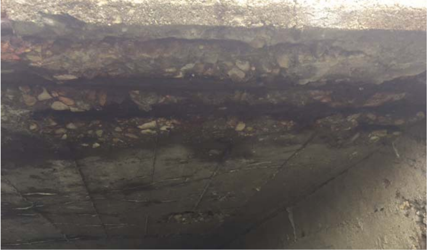
Photo 15 - North Headwall Spalls with Reinforcement
