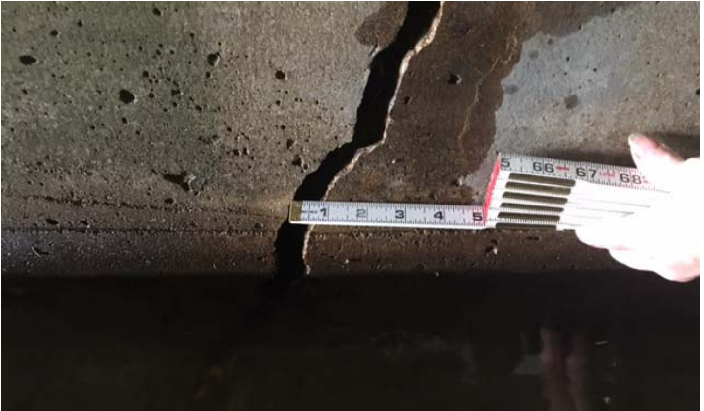
Photo 9 - East Wall Crack Closeup
