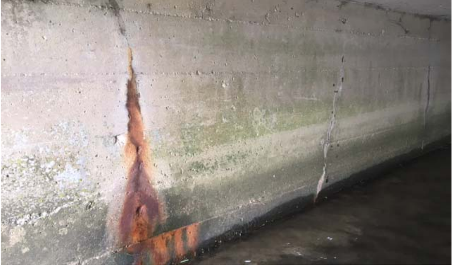
Photo 13 - East Wall North End Cracks
