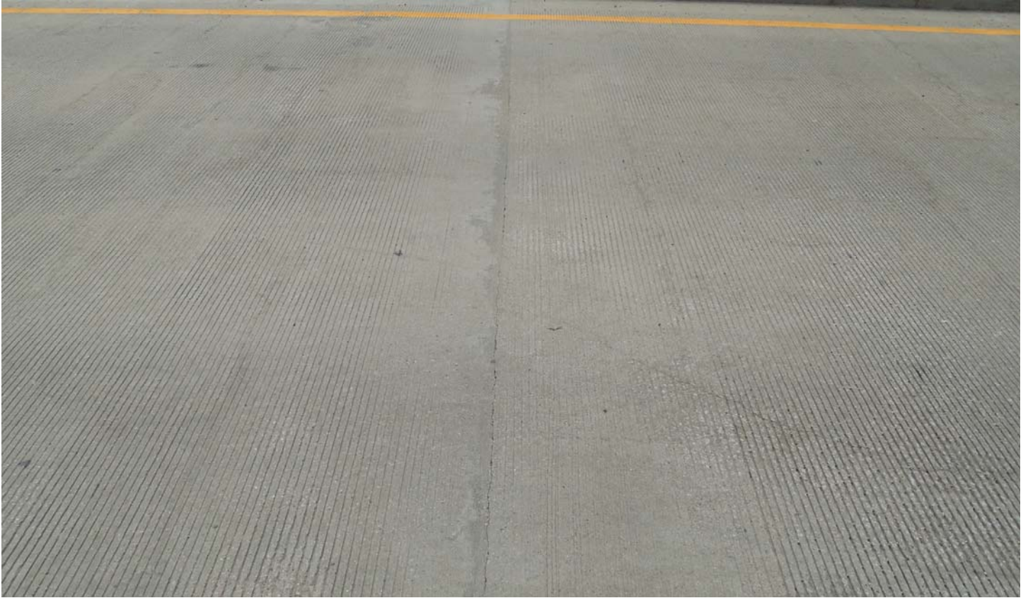
Photo 61 - Top of Deck in Span 4 - Cold Joint
