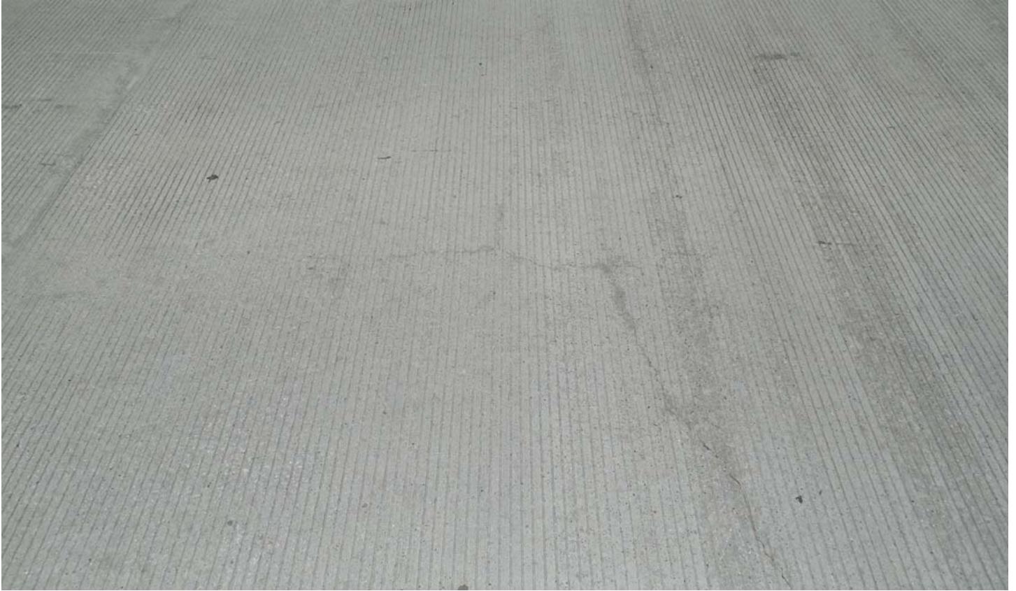
Photo 59 - Top of Deck - Typical Cracking in Span 2
