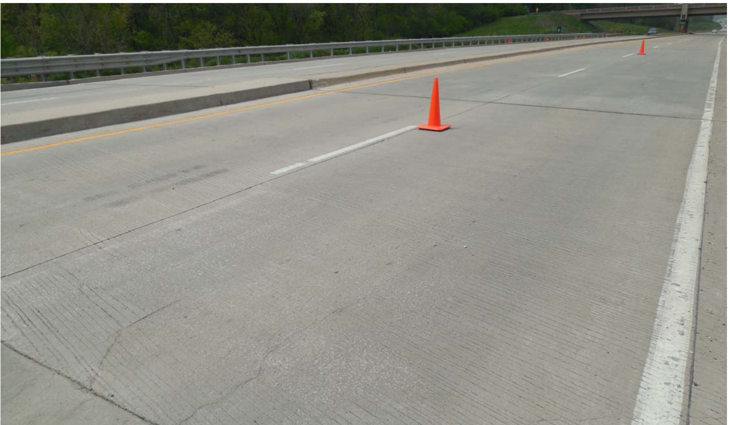
Photo 50 - West Approach - Westbound Lanes
