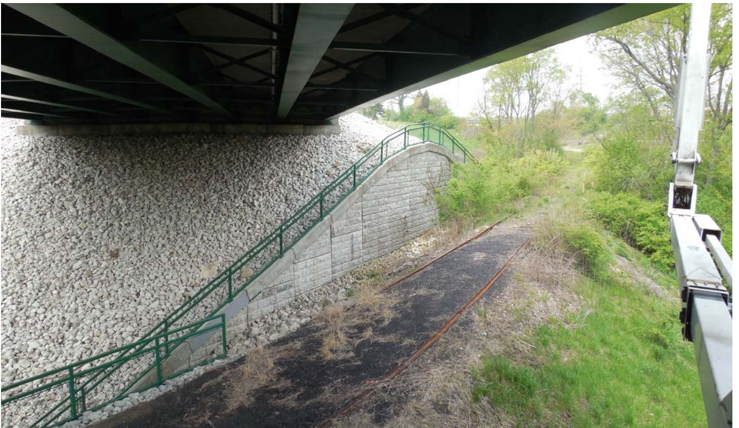
Photo 42 - Slopewall and Retaining Wall of the West Abutment
