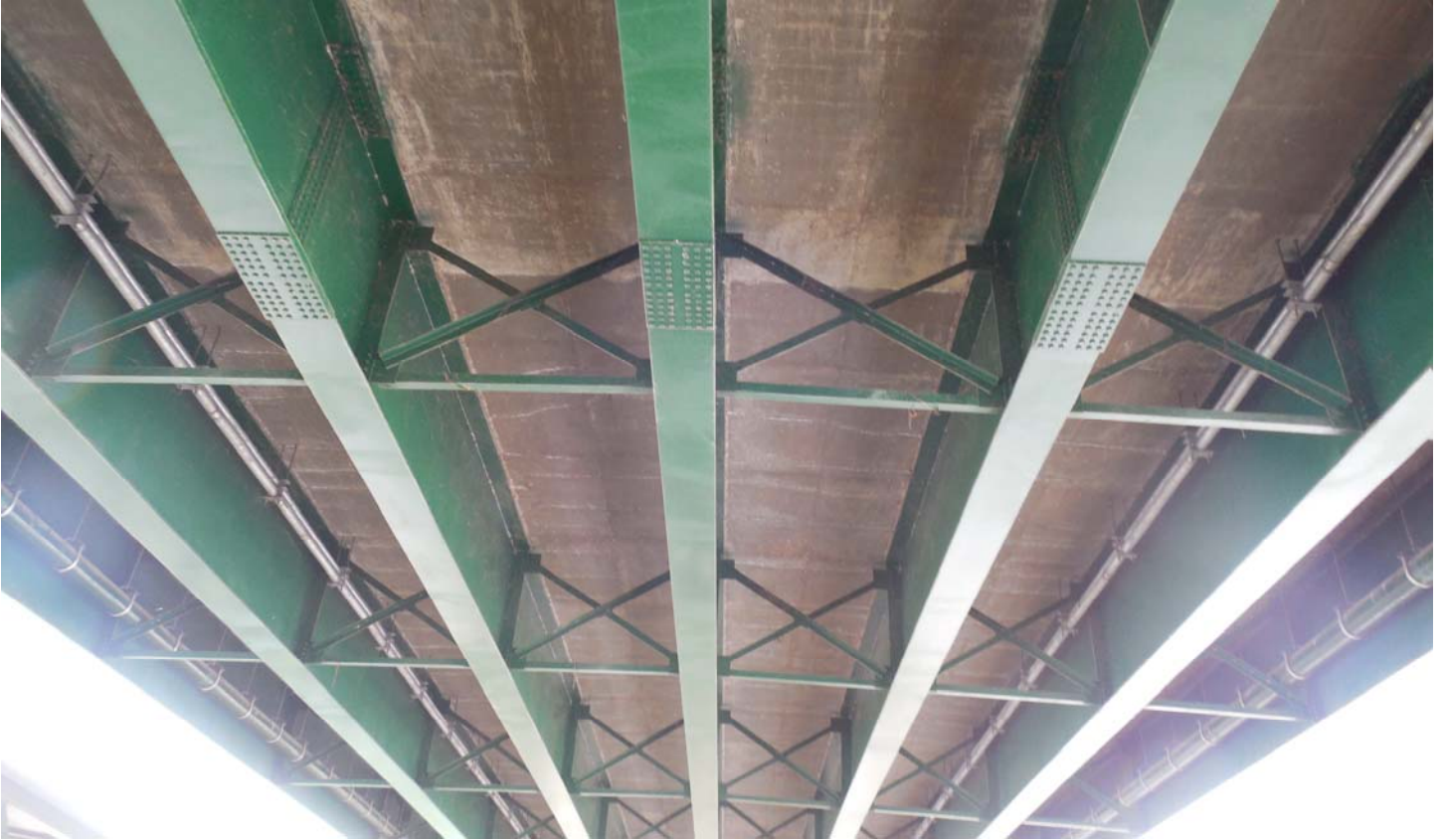
Photo 17 - Underside of Deck in Span 3 Looking West
