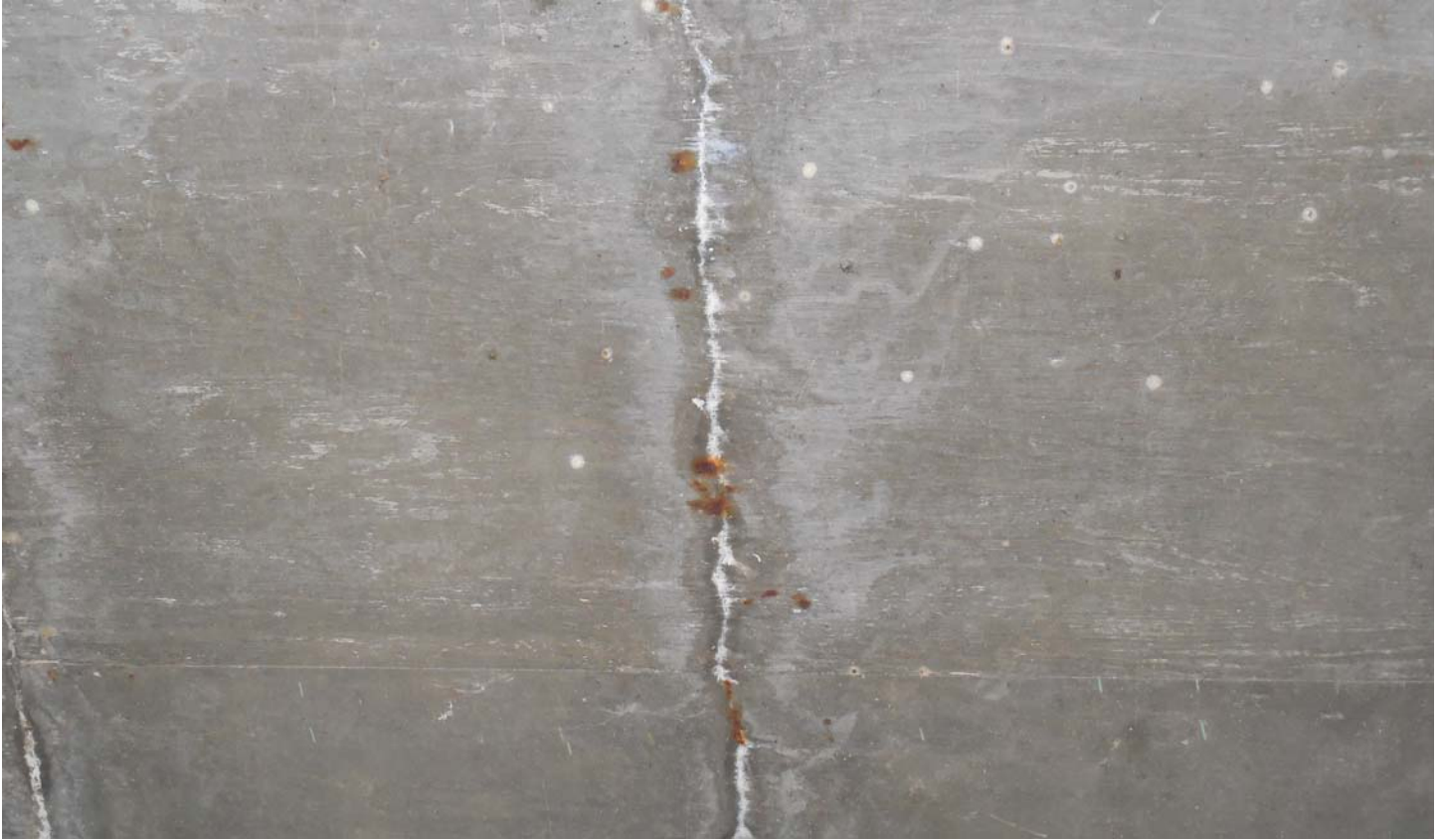
Photo 19 - Underside of Deck - Span 3 Bay 3 Rust Staining
