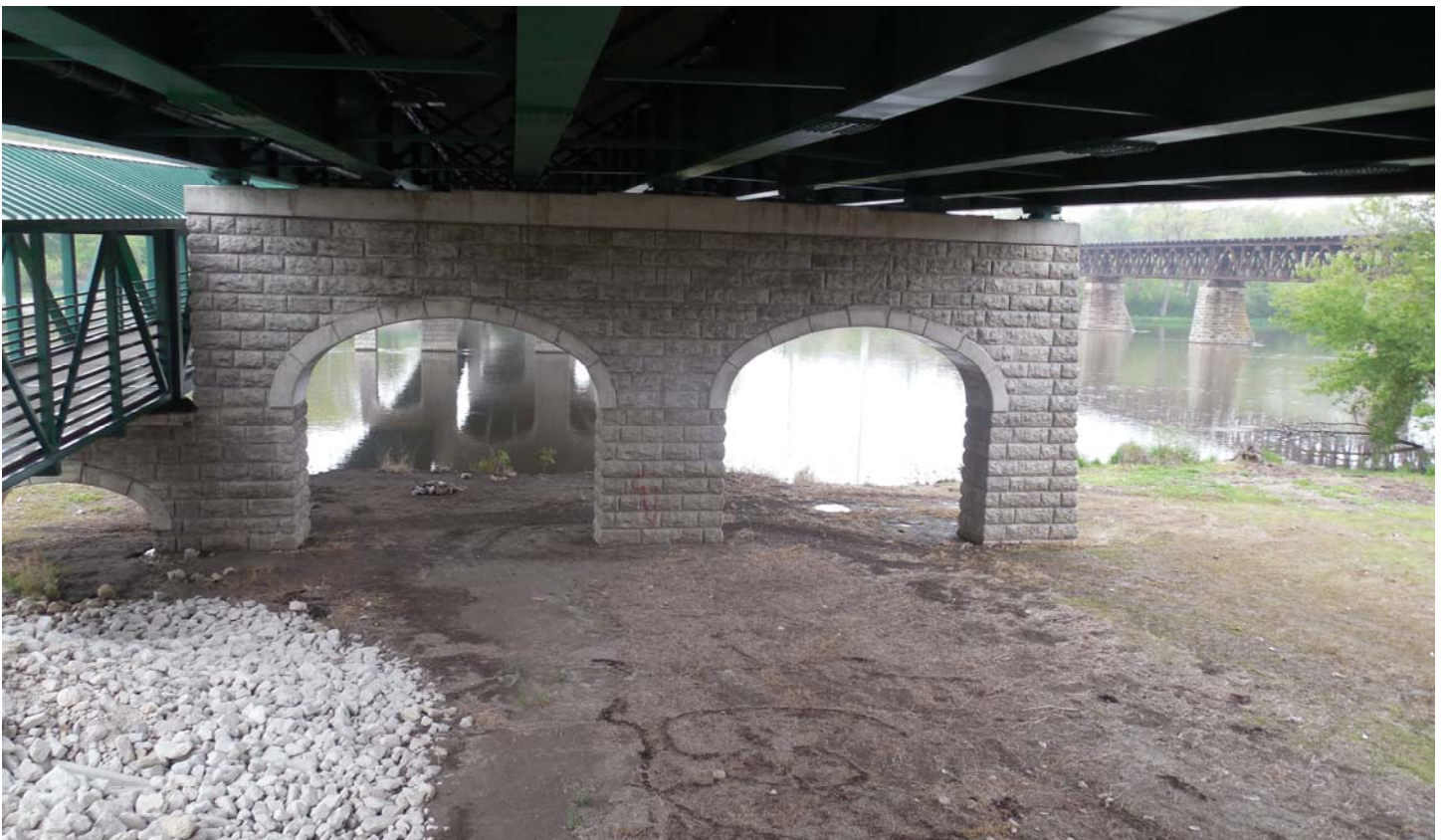
Photo 4 - East Face of Pier 4
