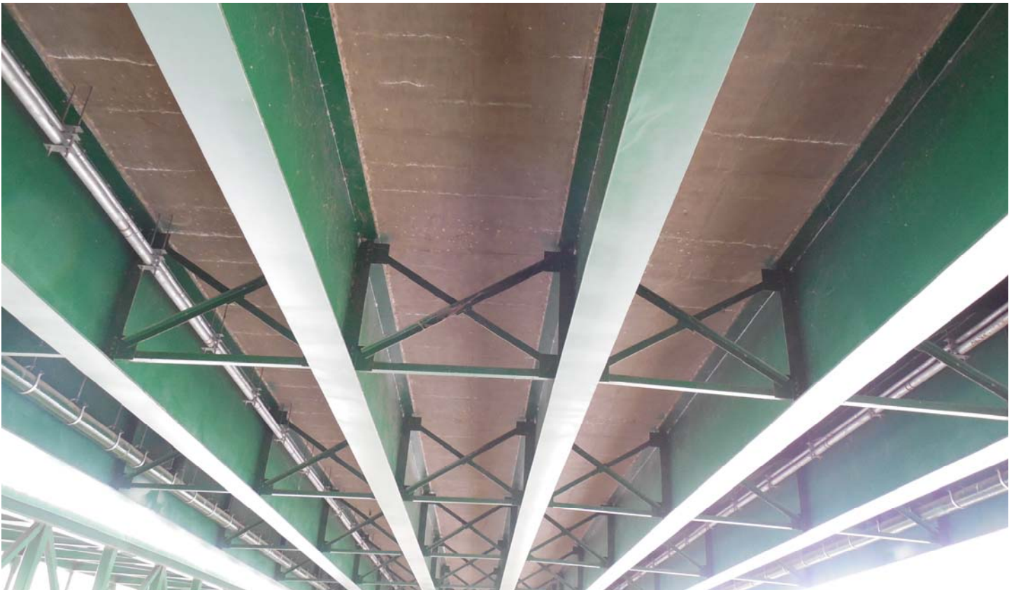
Photo 8 - Underside of Deck in Span 4
