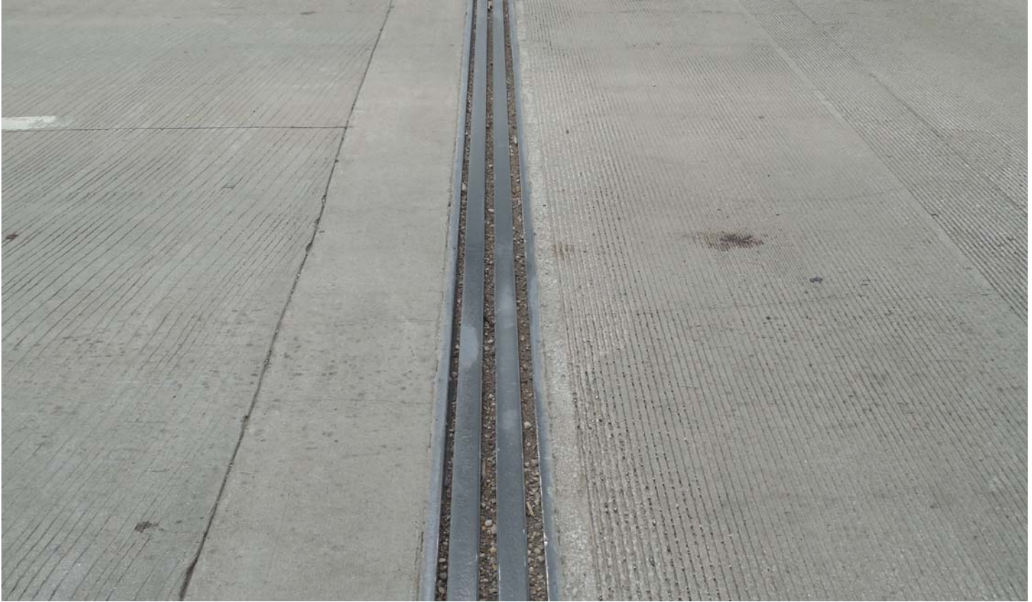
Photo 65 - Deck Joint at East Abutment in the Westbound Lane Looking South
