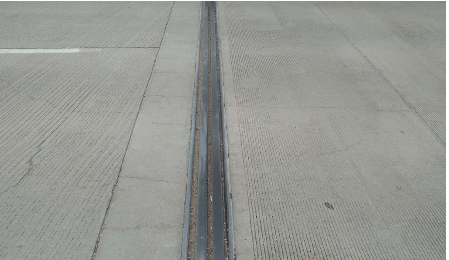
Photo 64 - Deck Joint at East Abutment in the Eastbound Lane Looking South
