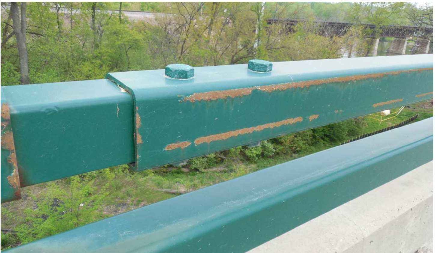
Photo 56 - Light Pole - North Rail near West Abutment Looking North
