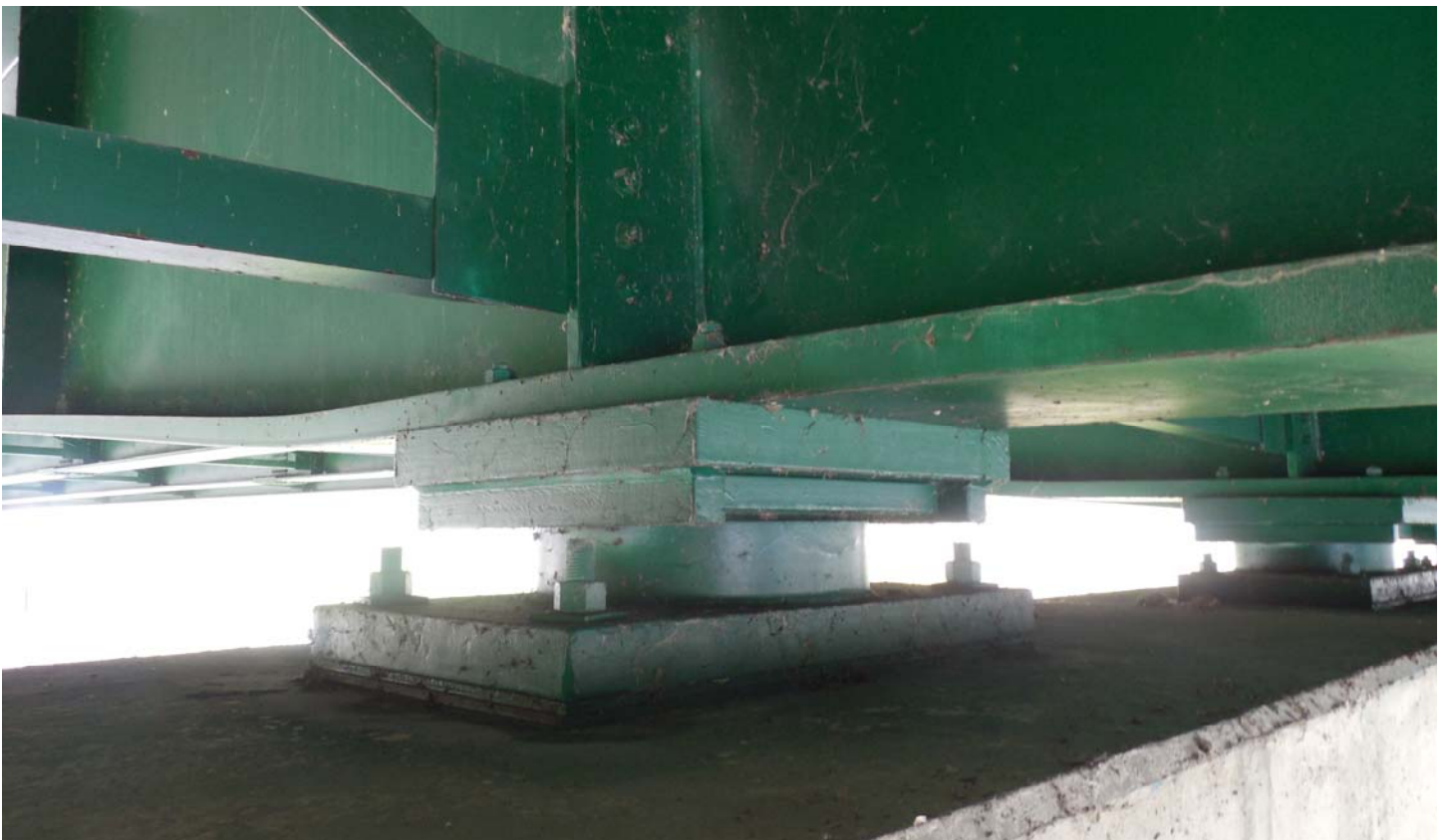
Photo 34 - Bearing at Pier 1
