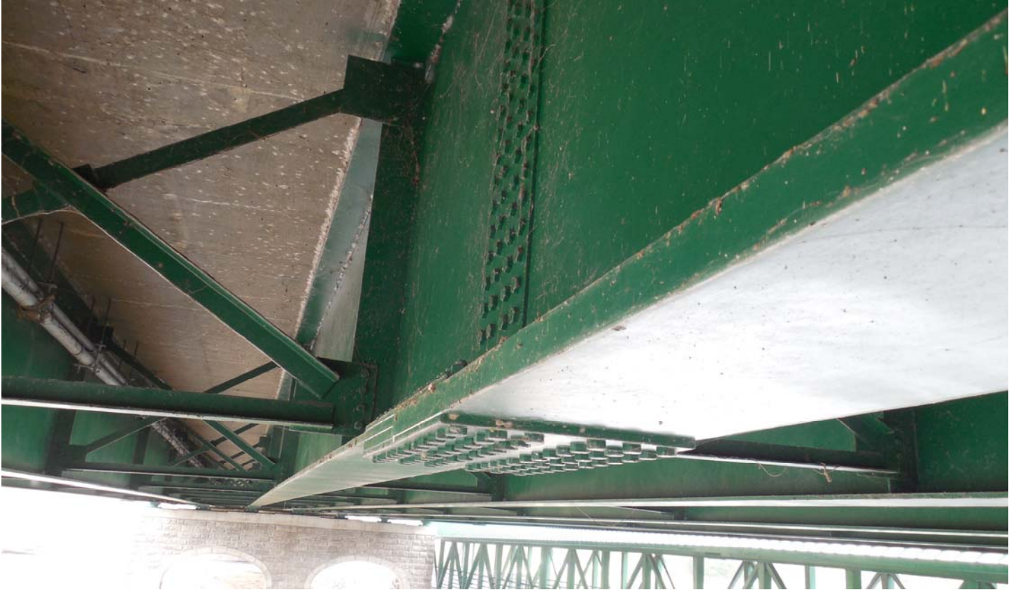
Photo 13 - Typical Beam Span 4
