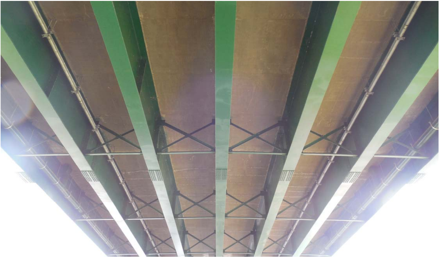
Photo 35 - Underside Deck in Span 2 from Pier 1
