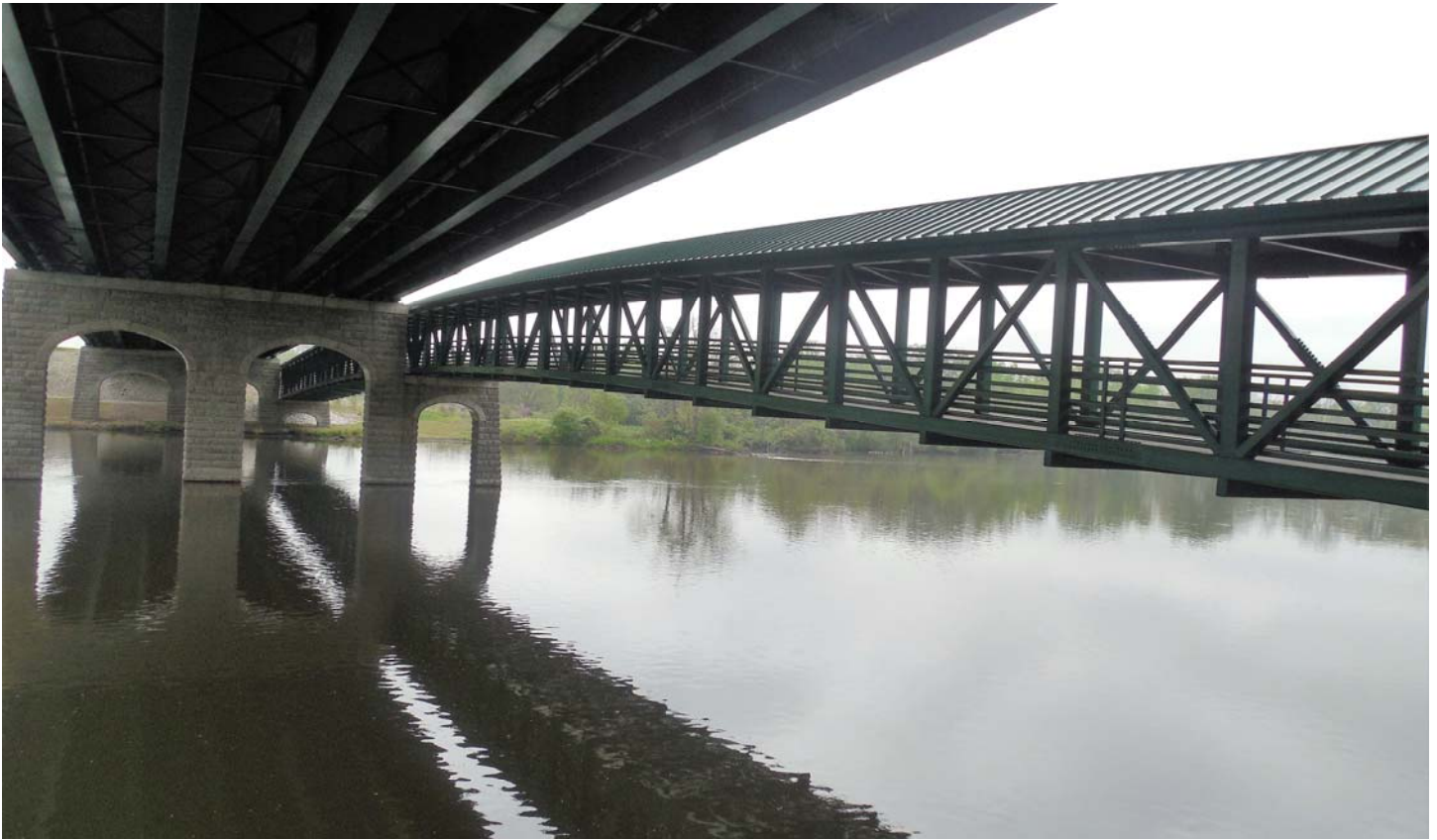
Photo 21 - Pedestrian Bridge Looking East From Pier 2
