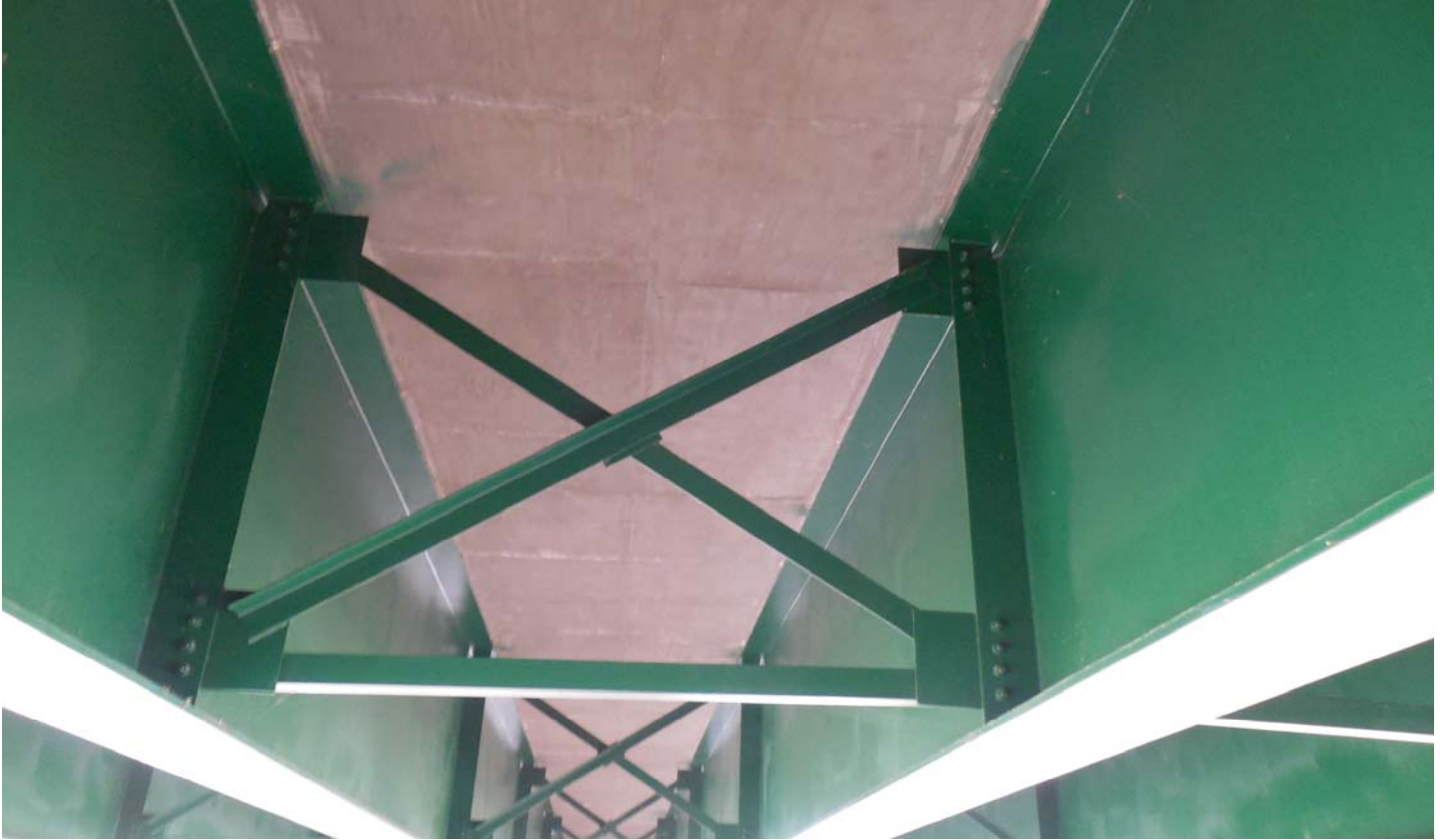
Photo 3 - Span 5 - Typical Diaphragm
