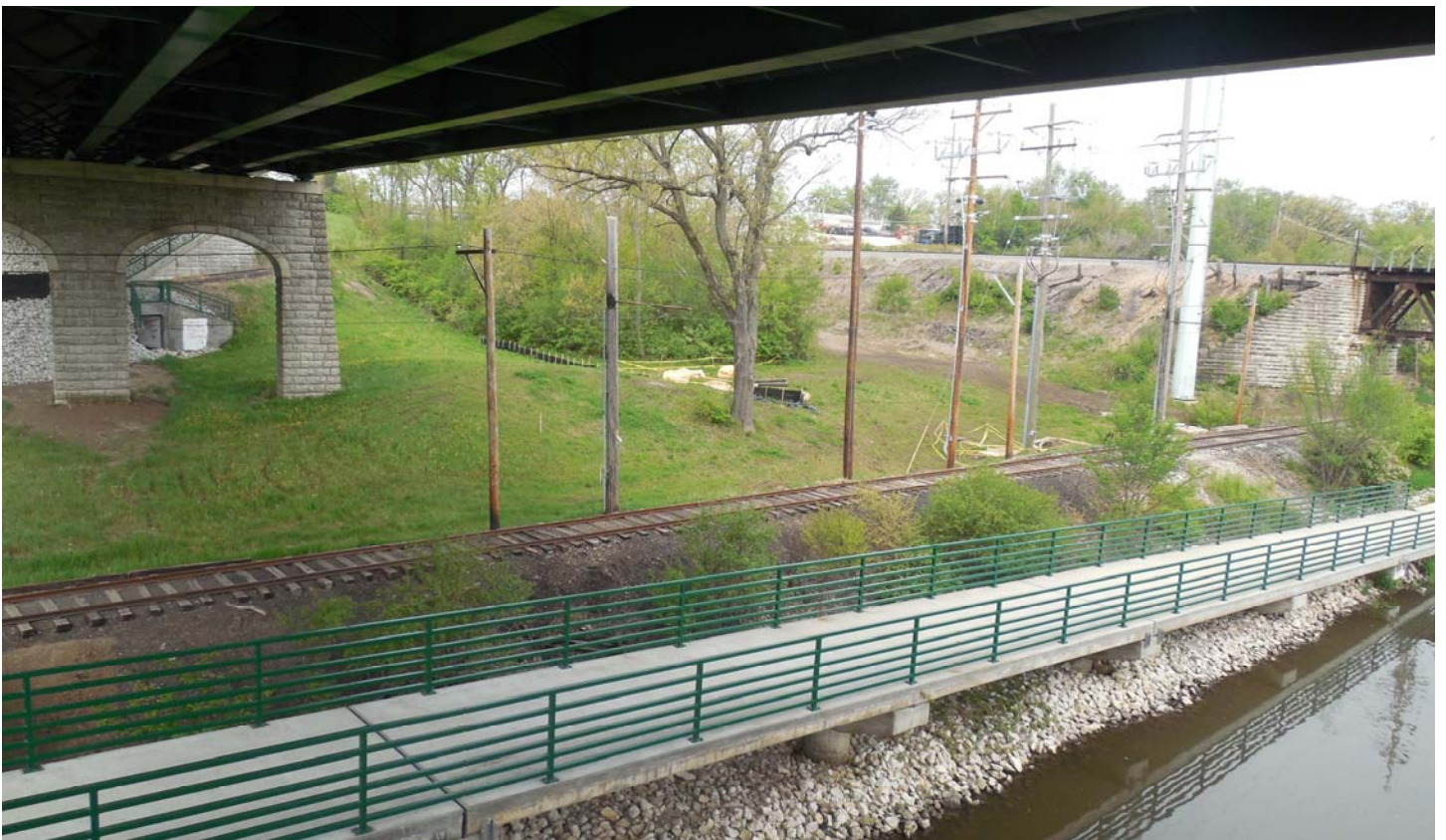
Photo 28 - Track and Power Lines in Span 2
