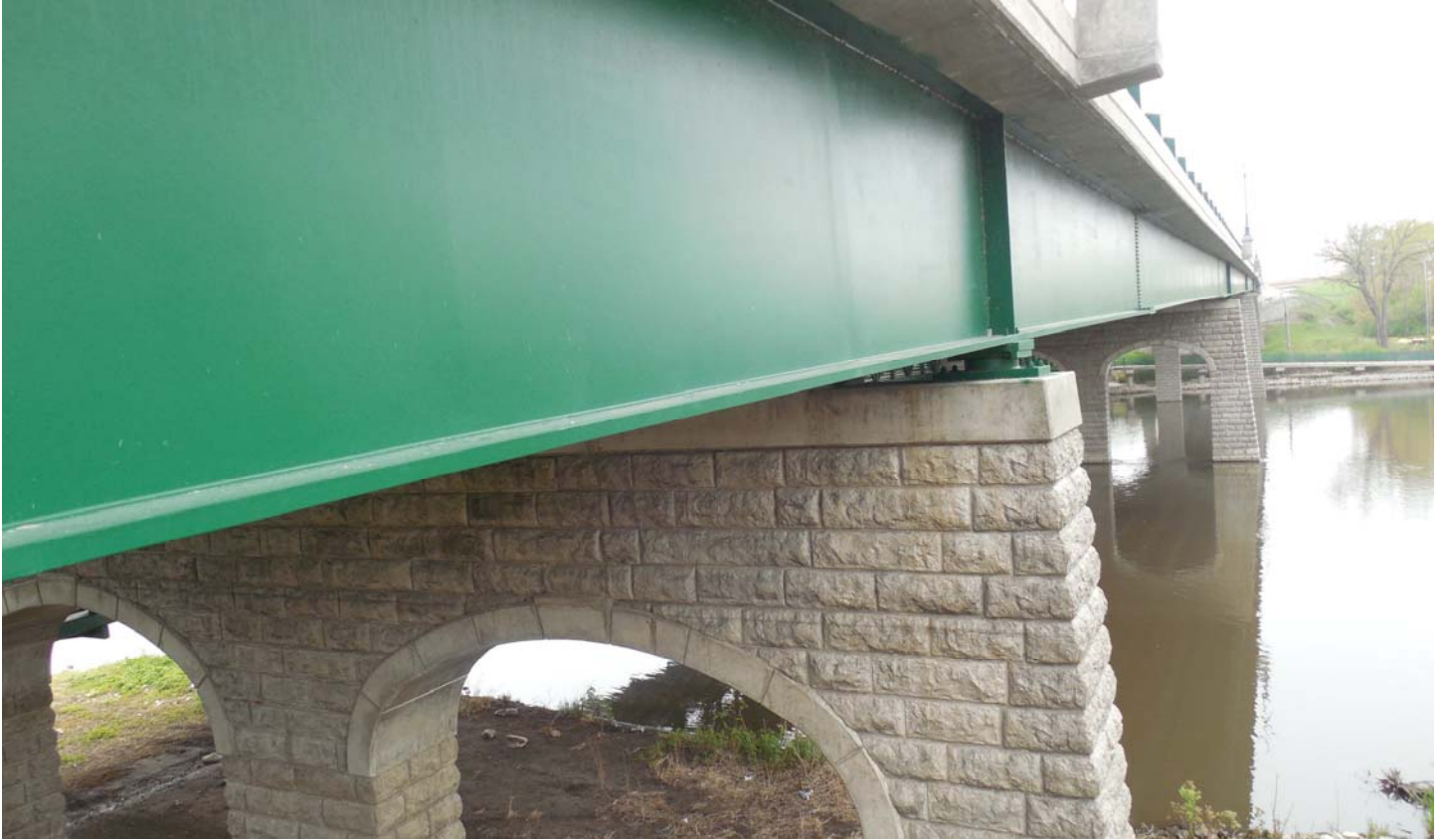
Photo 7 - North Fascia Looking Southwest
