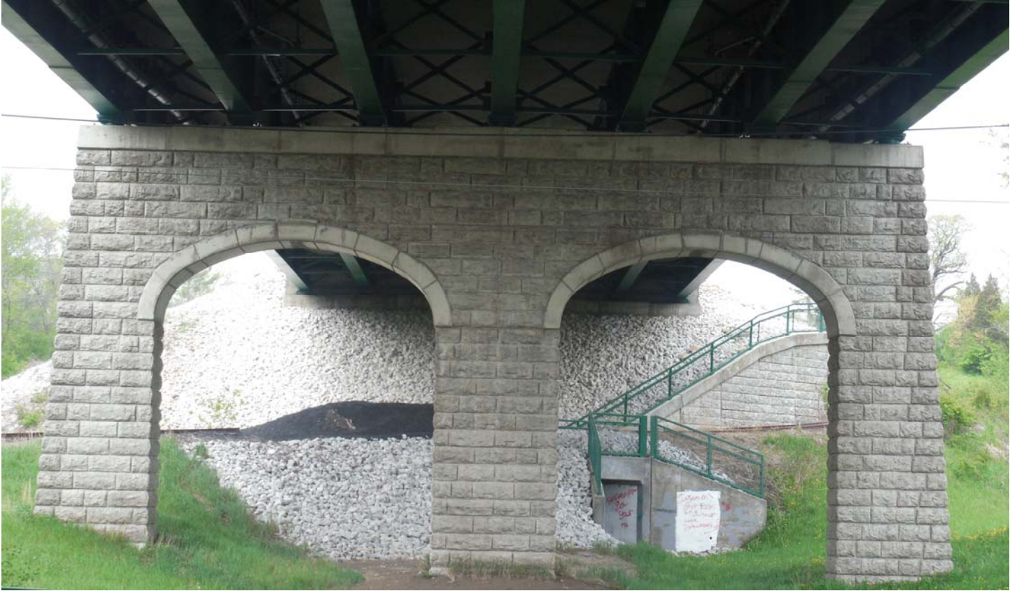
Photo 27 - East Face of Pier 1
