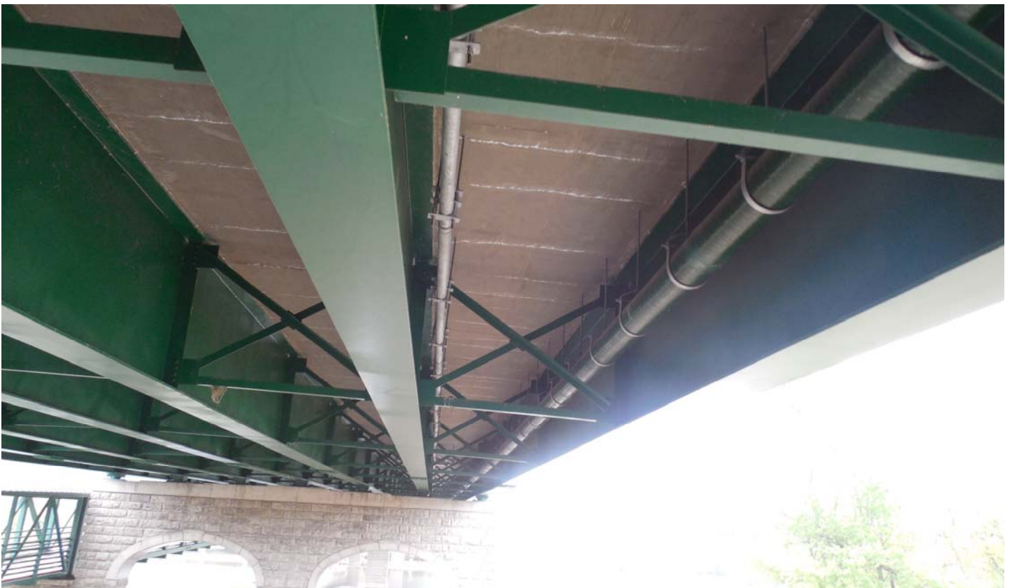
Photo 2 - Underside of Deck - North Bay of Span 5
