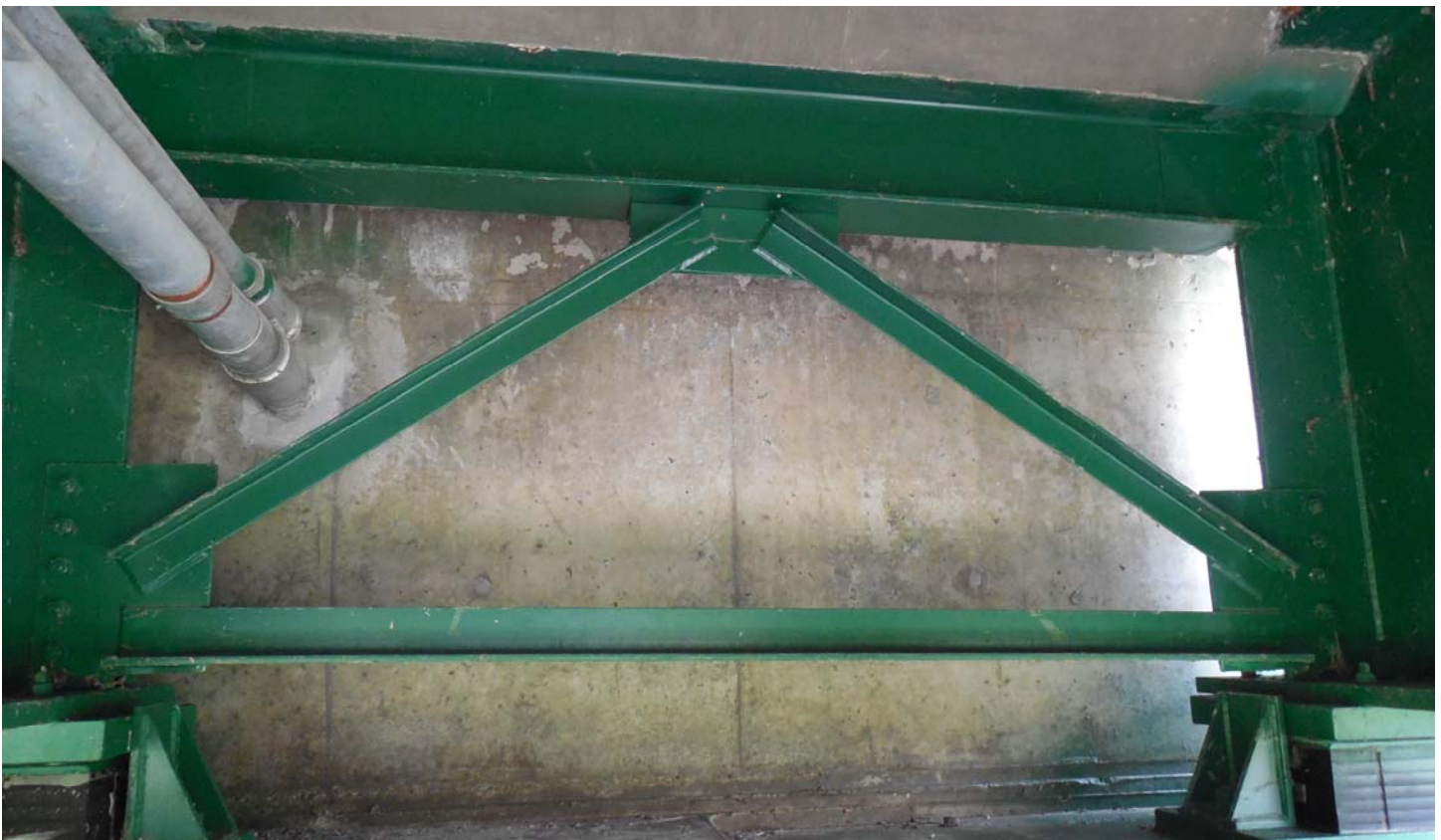
Photo 44 - Diaphragm and West Abutment Backwall - Bay 1
