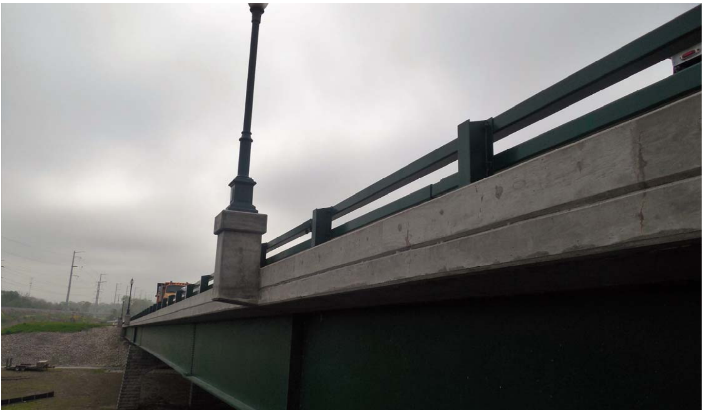
Photo 16 - Outside of North Parapet and Lightpole Looking Southeast
