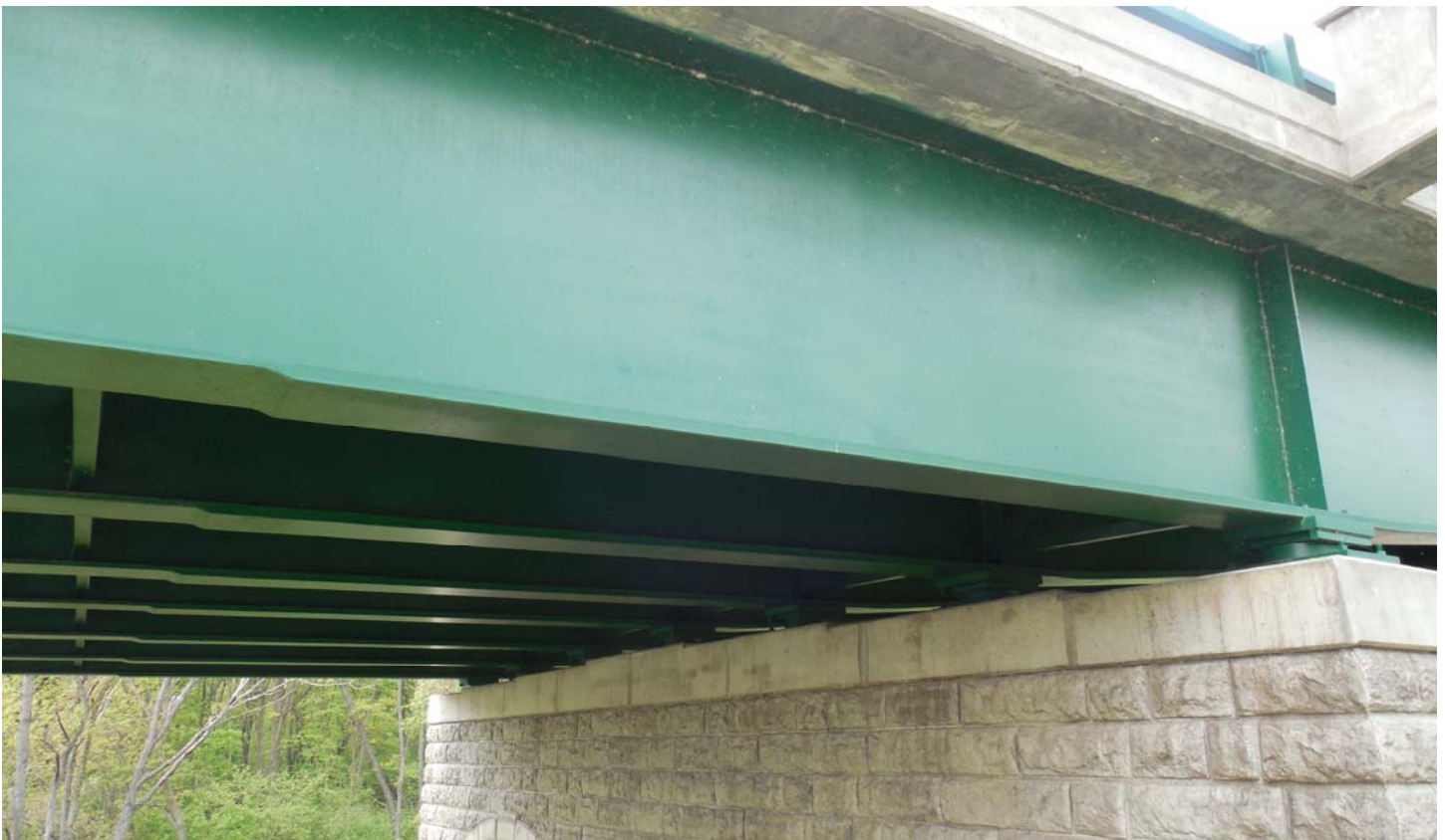
Photo 32 - Span 2 - Change in Flange near Pier 1
