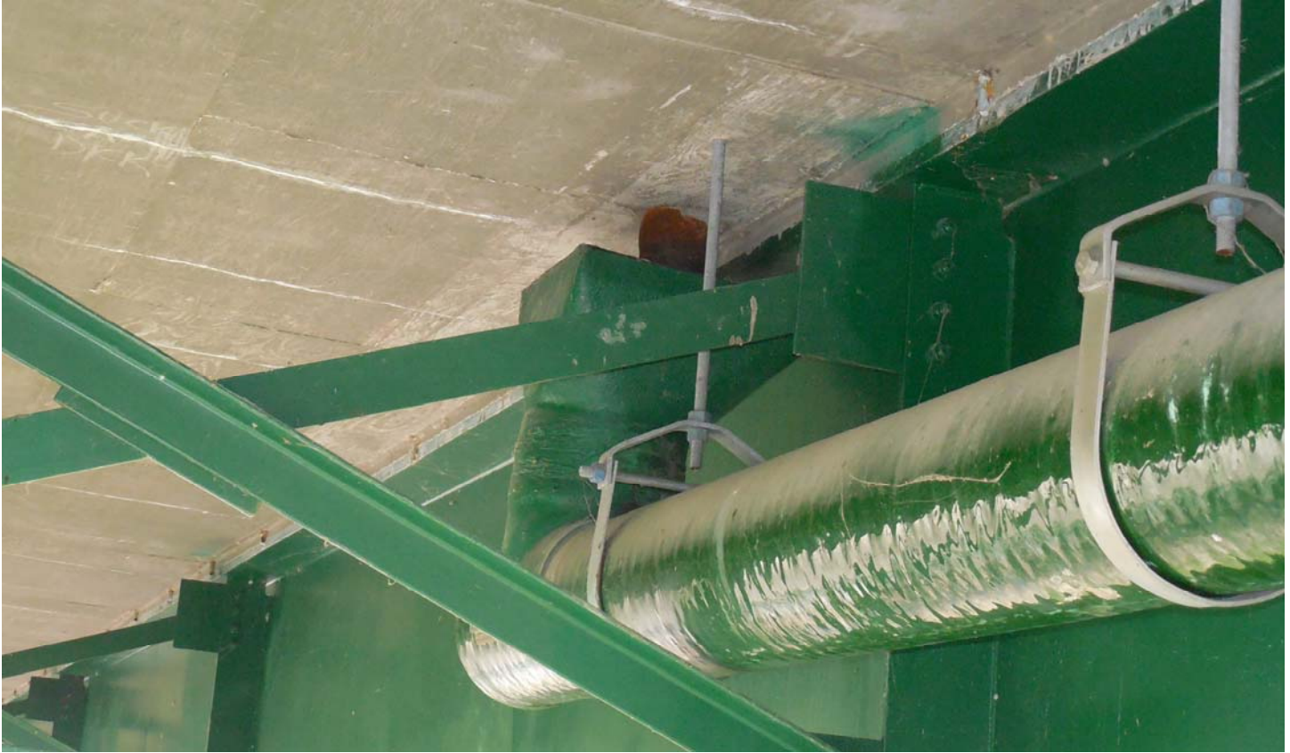
Photo 43 - Drain Detail Underside Bay 1 - Span 1
