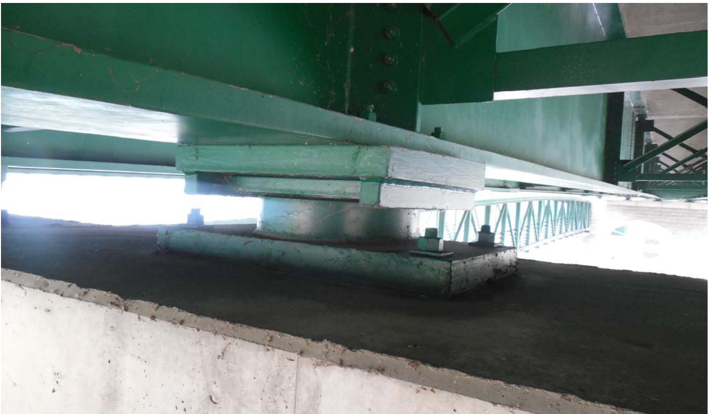
Photo 6 - Typical Bearing at Pier 4
