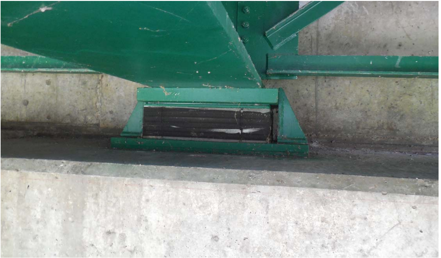
Photo 45 - Bearing at the West Abutment
