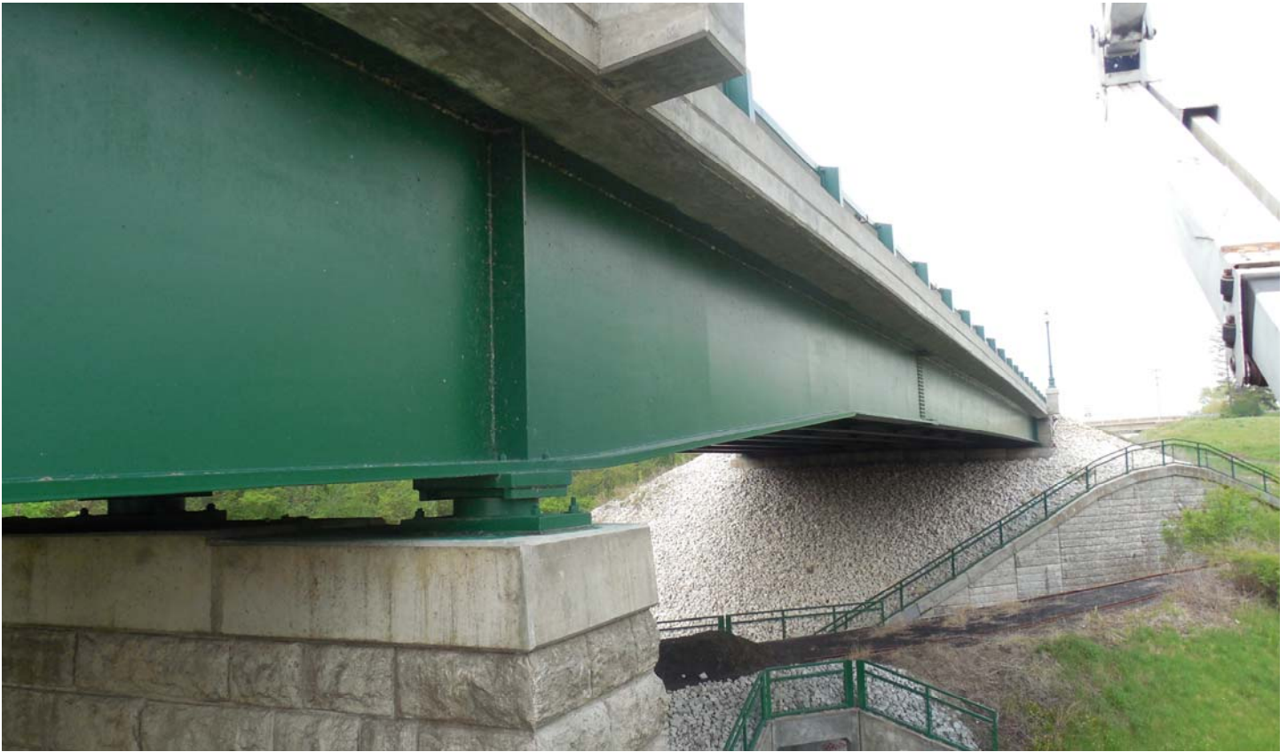
Photo 31 - Span 1 - Change in Beam Section
