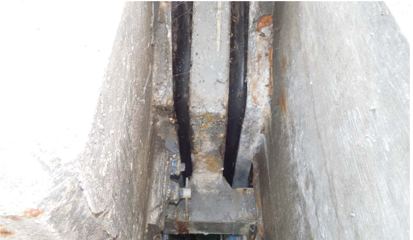
Photo 48 - Underside Joint at West Abutment Looking South
