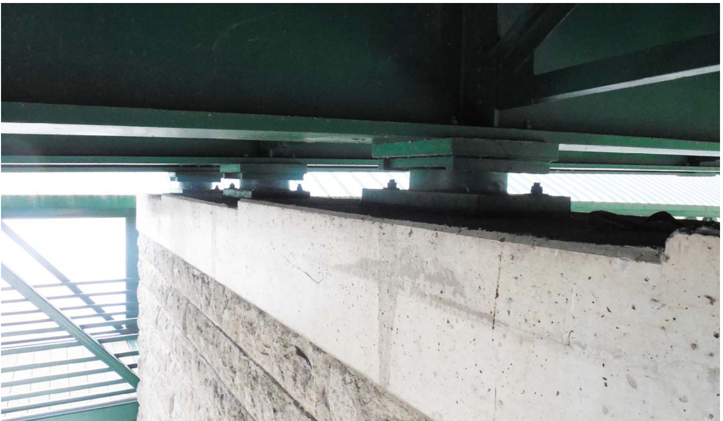
Photo 12 - Bearings at Pier 3
