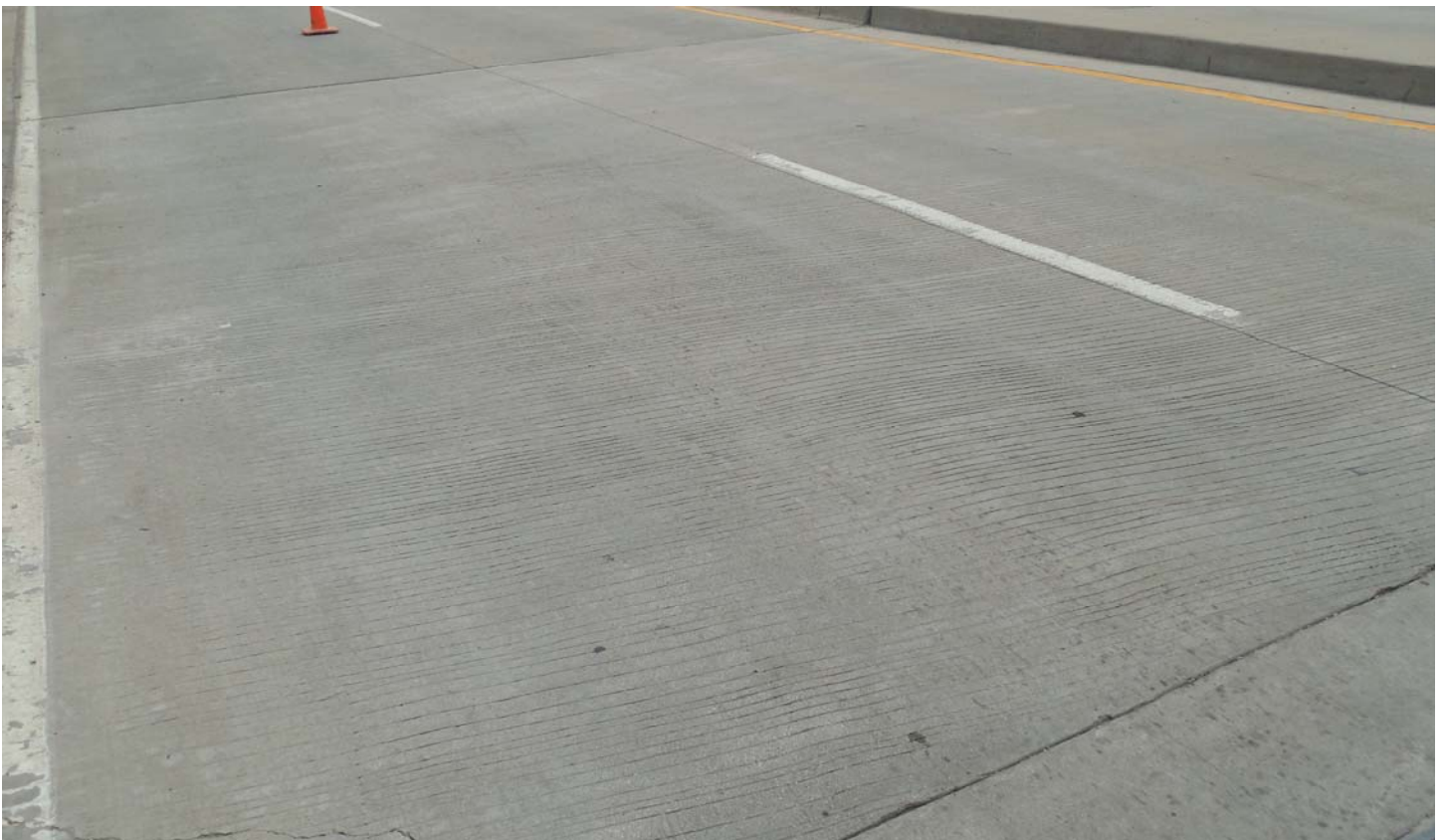
Photo 62 - East Approach - Westbound Lanes
