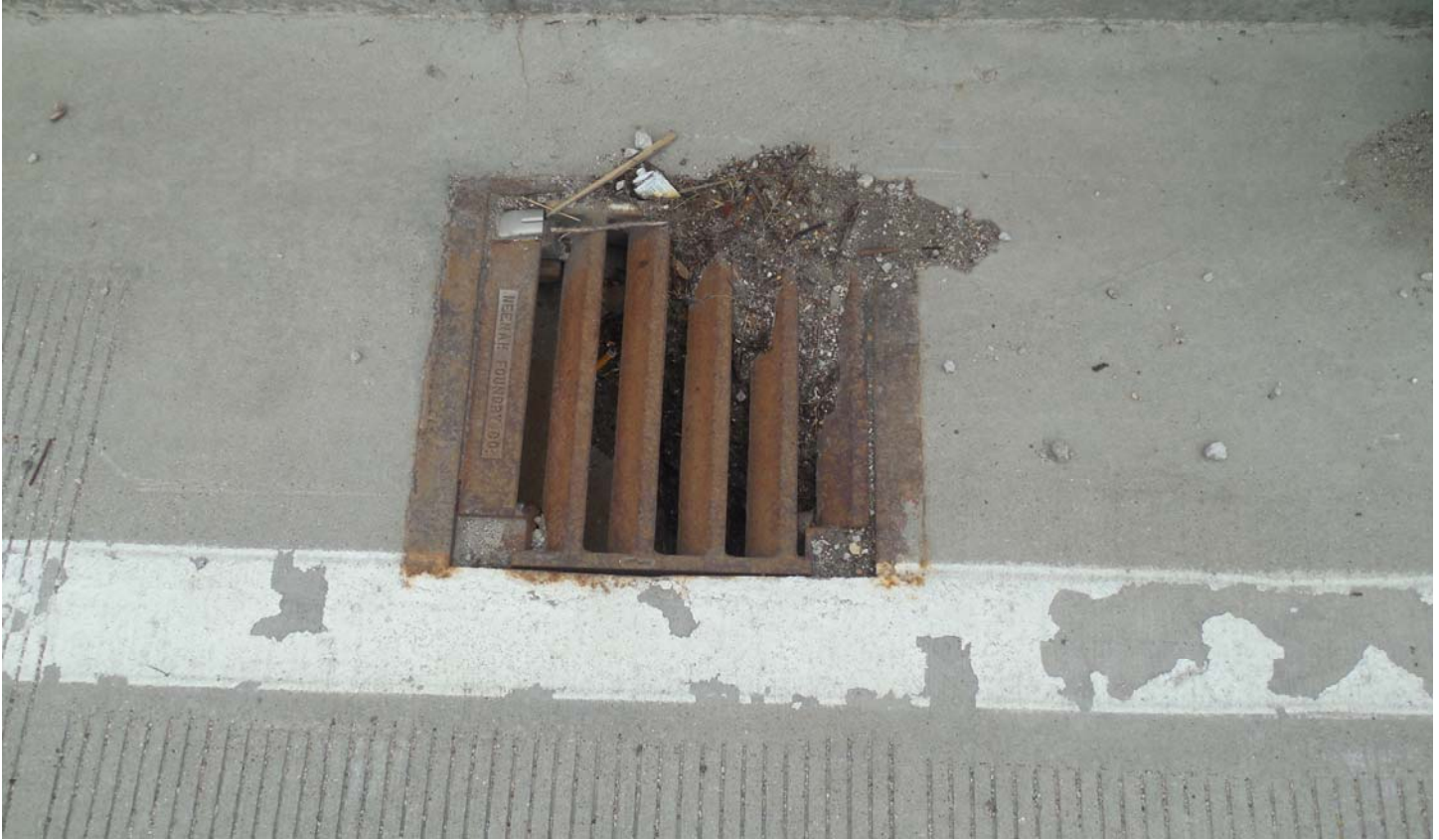
Photo 57 - Top of Deck Drain - Span 1
