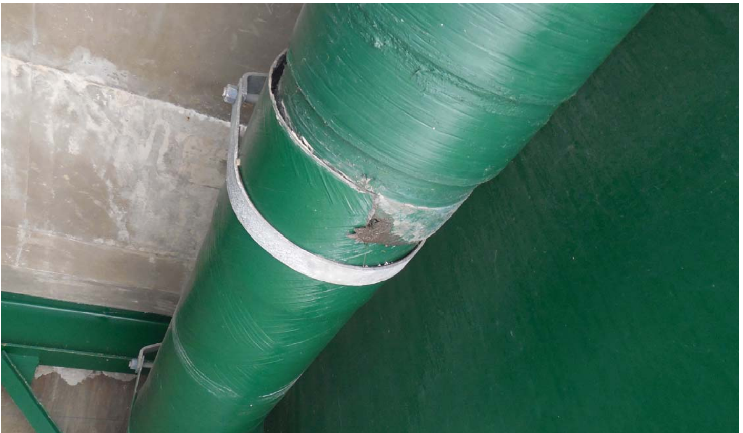
Photo 72 - Drainage Pipe in Bay 6 near the East Abutment
