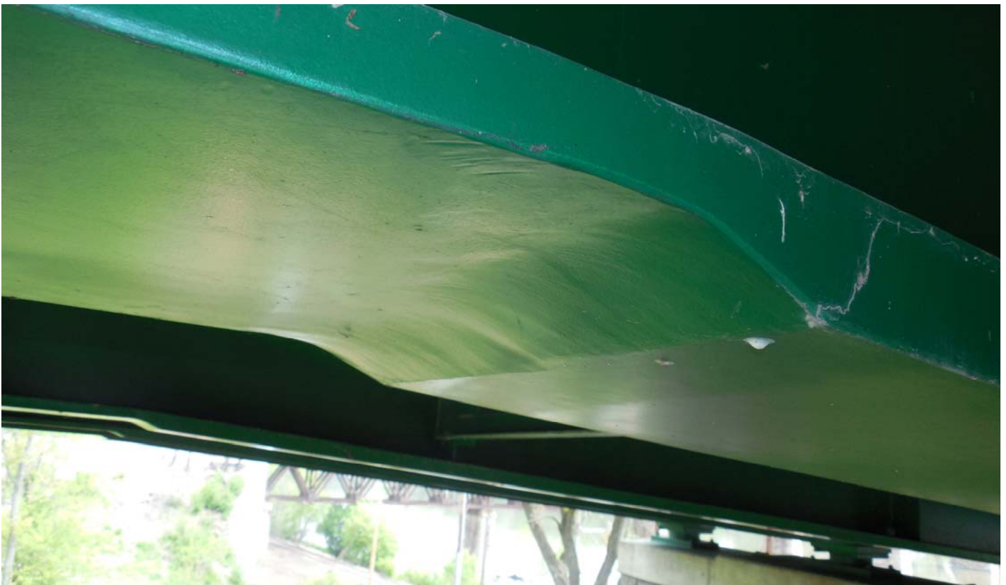
Photo 38 - Span 1 - Beam 4 at Change of Section
