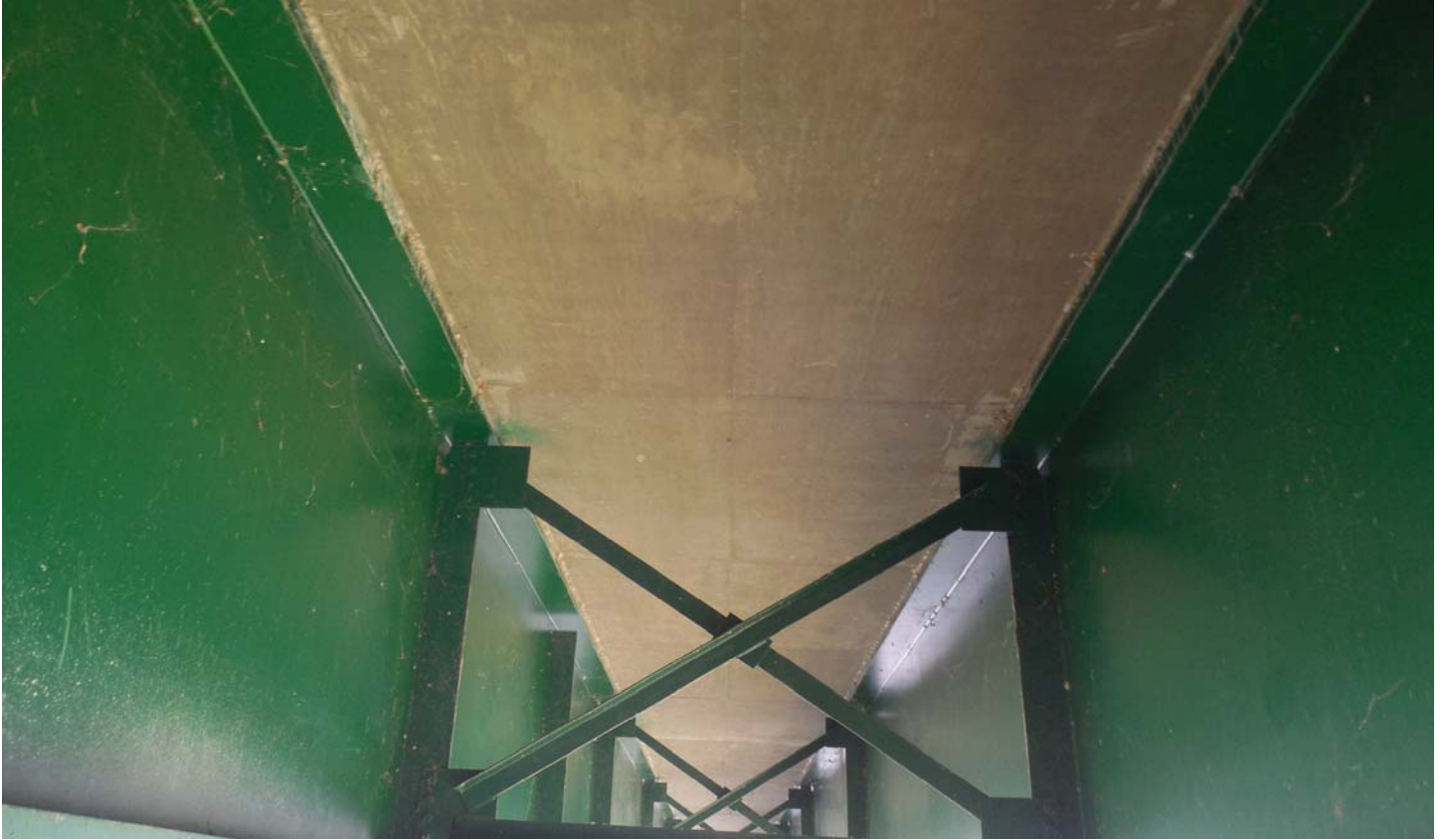
Photo 33 - Span 2 From Pier 1
