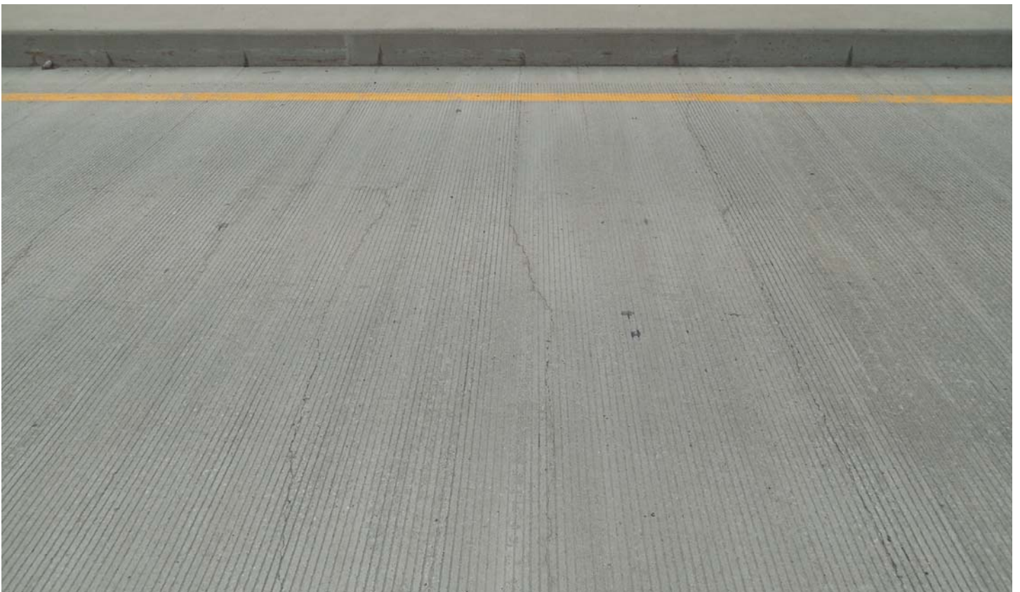
Photo 60 - Top of Deck - Typical Cracking in Span 3
