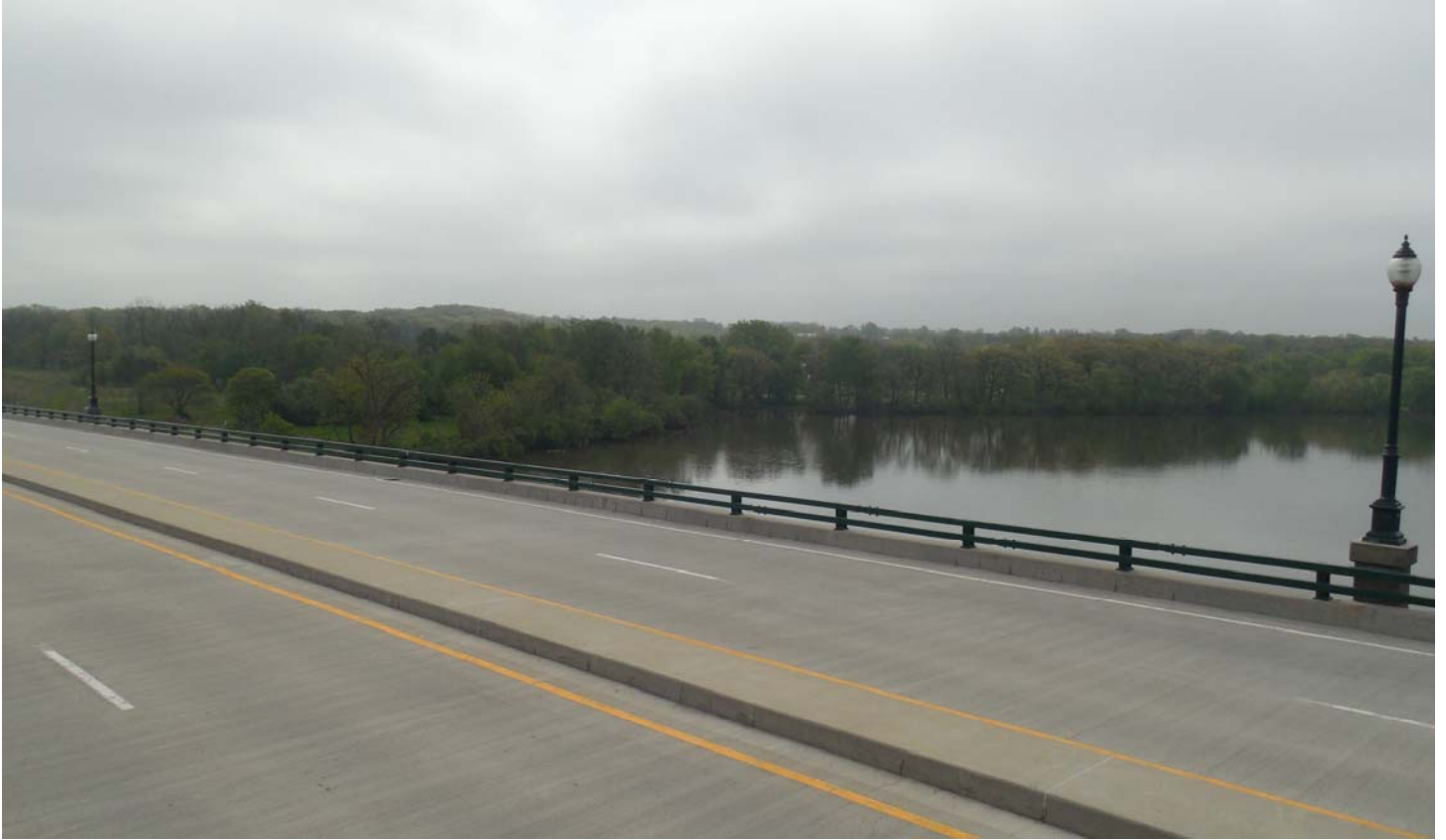
Photo 25 - Looking Southeast Across Bridge
