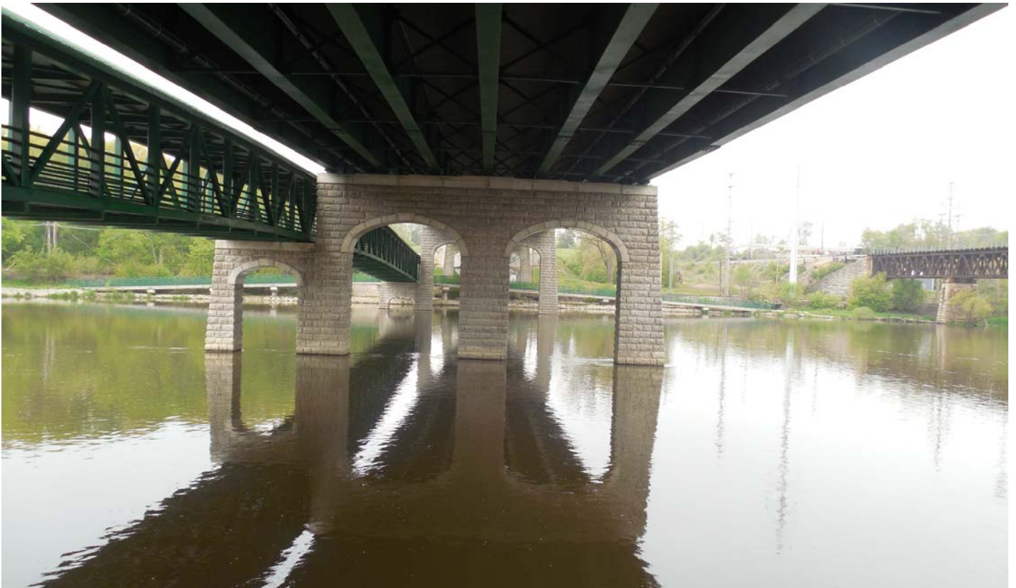
Photo 10 - East Face of Pier 3
