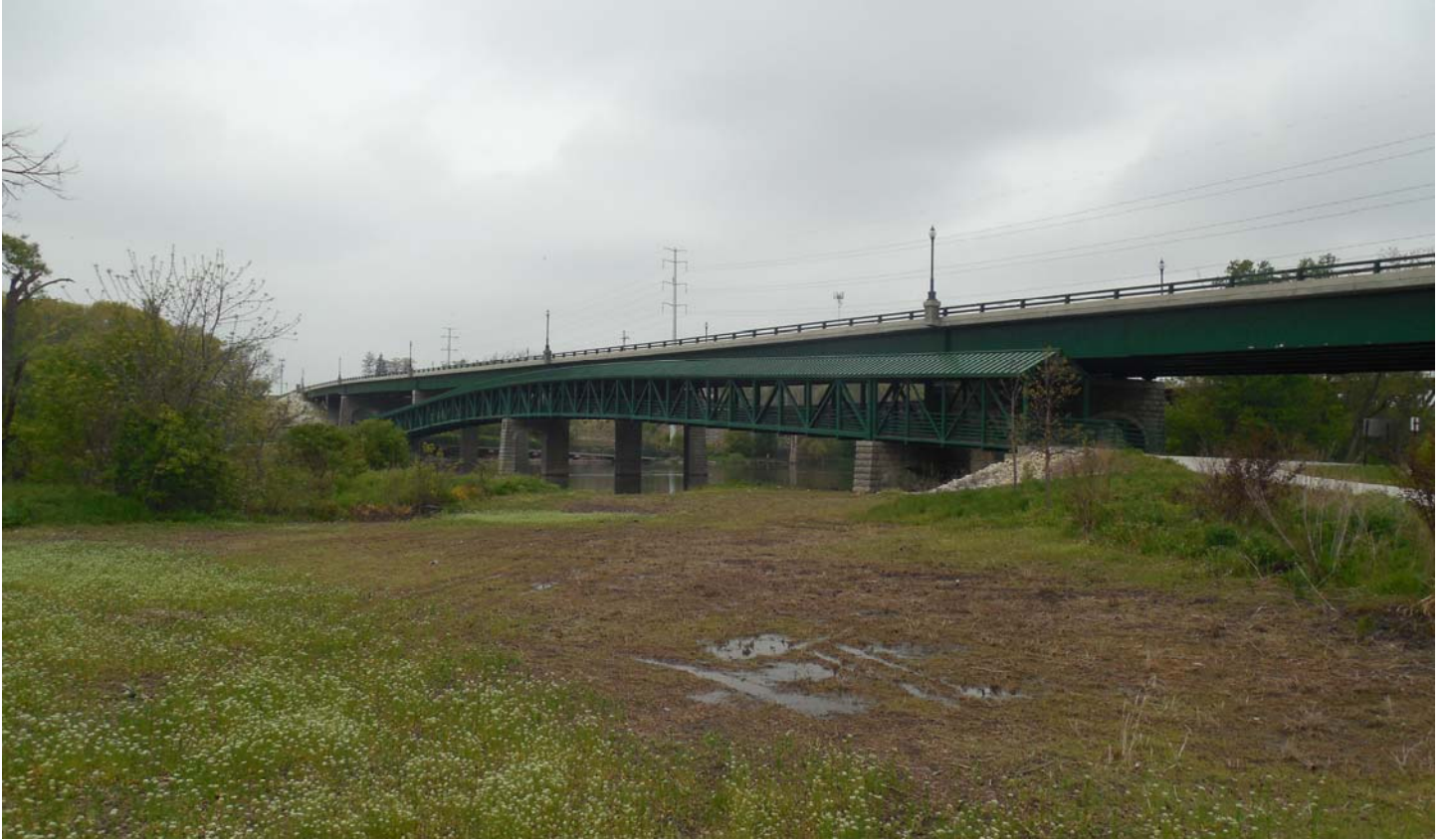
Photo 73 - South Elevation Looking Northwest
