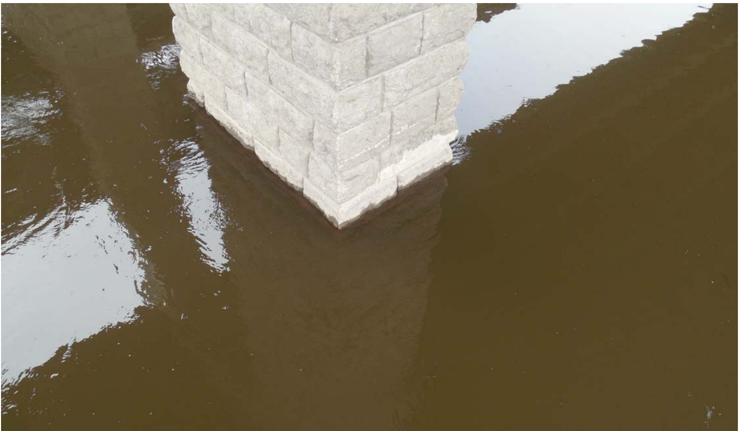
Photo 22 - Pier 2 Column at the Waterline
