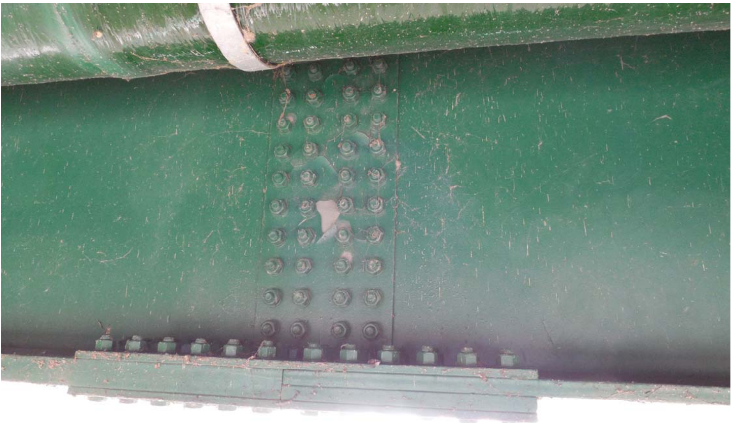
Photo 14 - Span 4 - Paint Failure on Splice Plate
