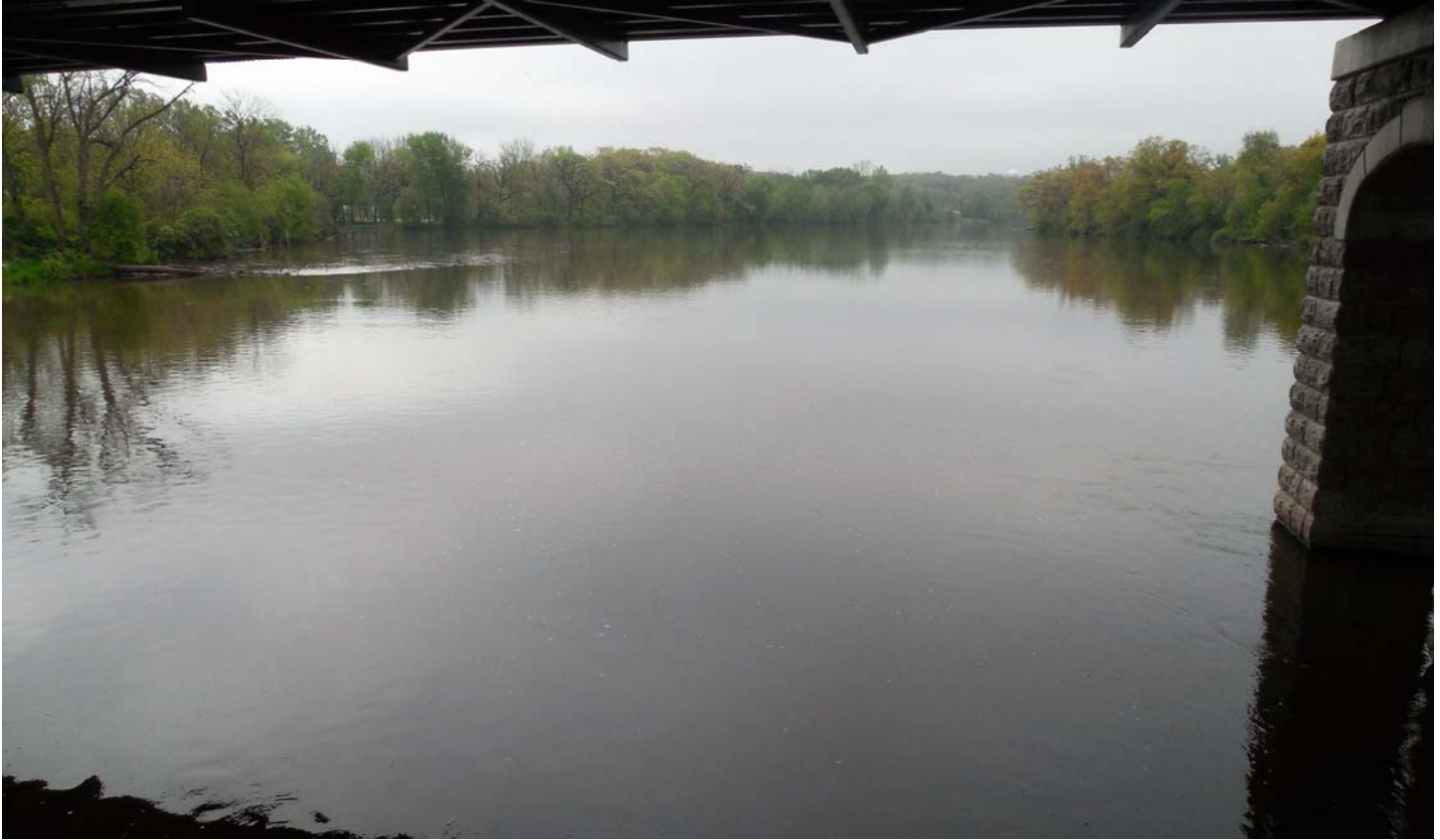
Photo 11 - Looking South Downstream from Bridge
