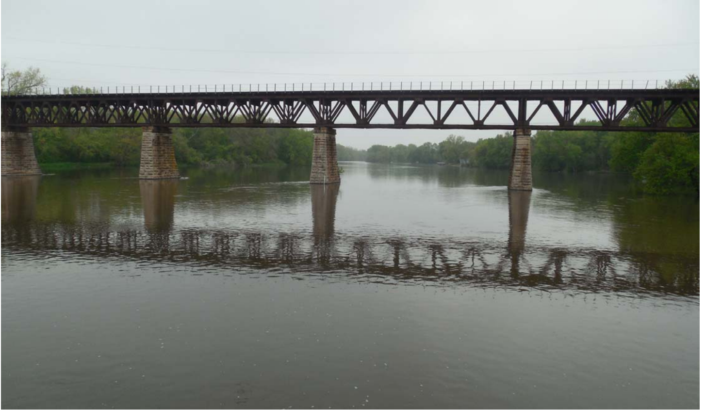
Photo 15 - Looking North Upstream from Bridge
