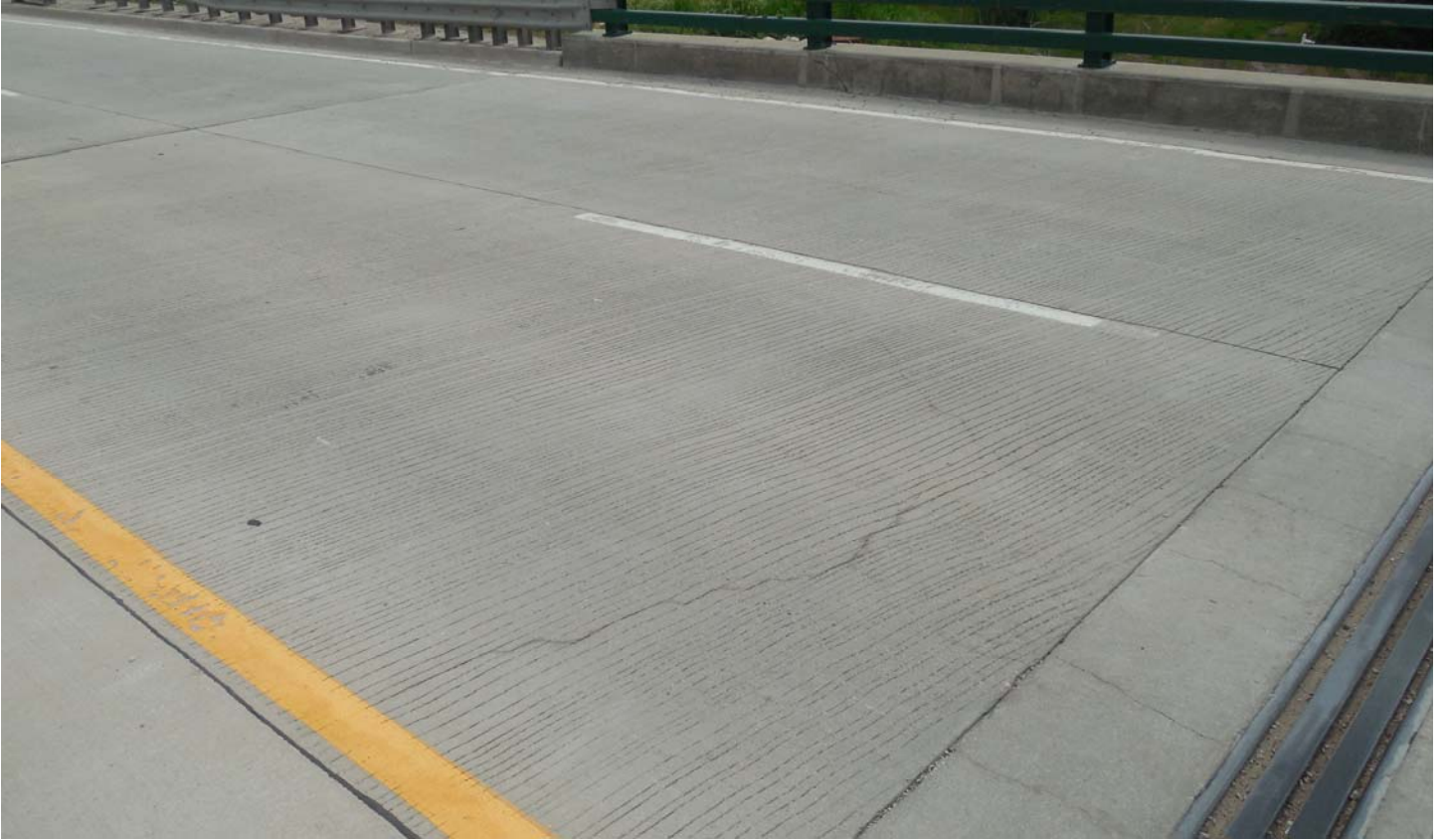
Photo 63 - East Approach - Eastbound Lanes
