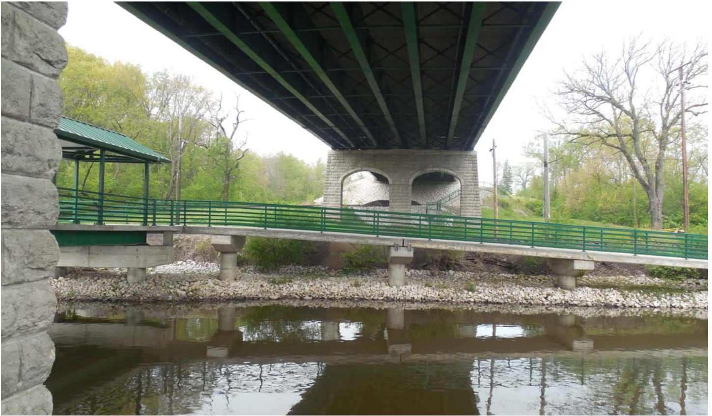
Photo 23 - Span 2 Looking West
