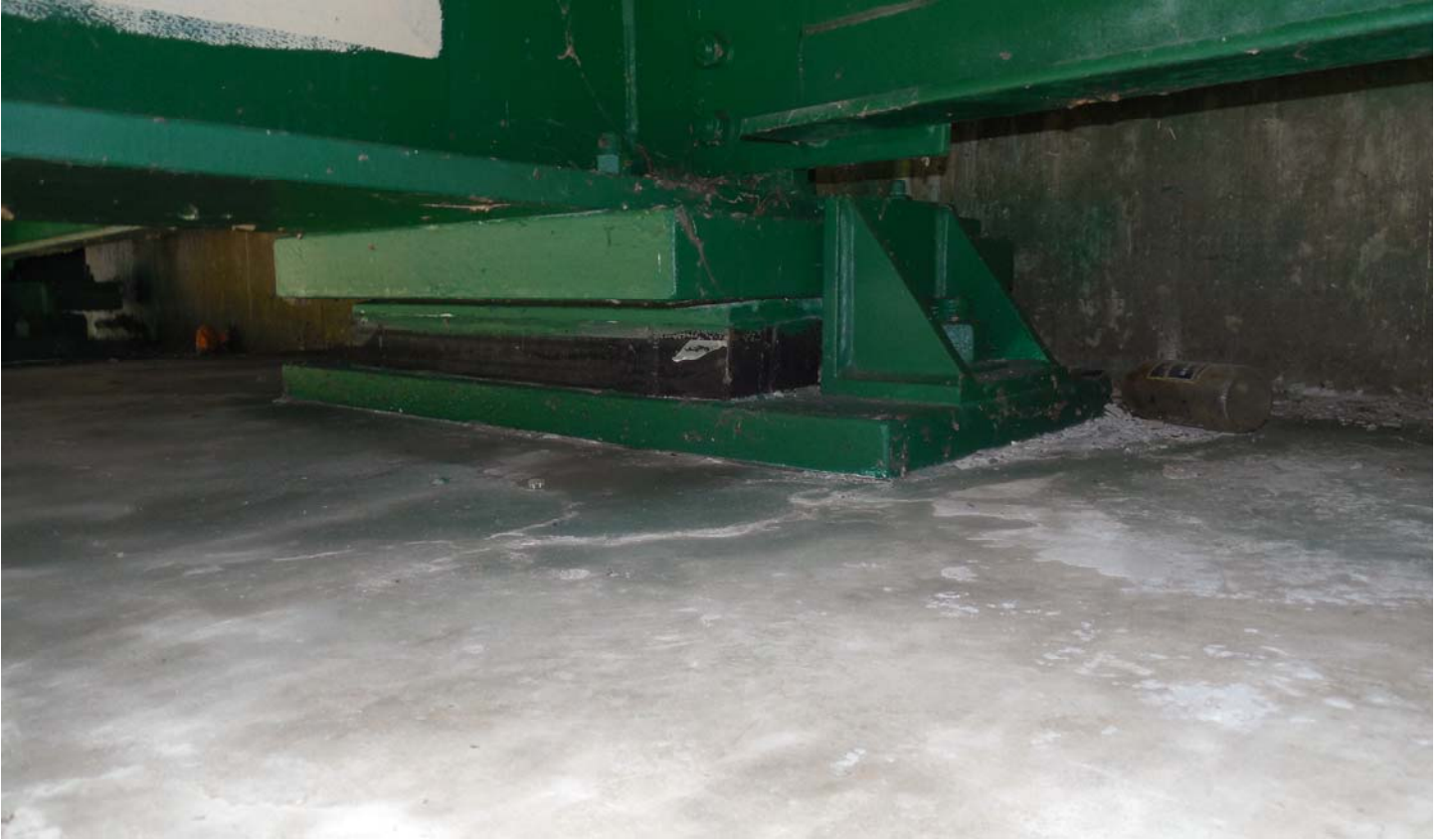
Photo 69 - Bearing at East Abutment
