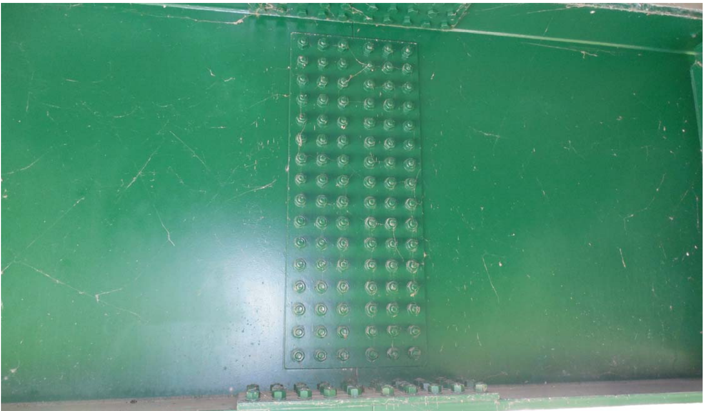
Photo 40 - Splice Plate of Beam 4
