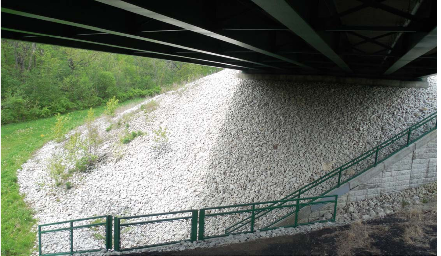
Photo 41 - Slopewall and Retaining Wall of the West Abutment
