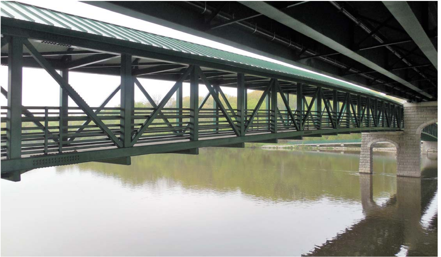
Photo 9 - Pedestrian Bridge Looking Southwest
