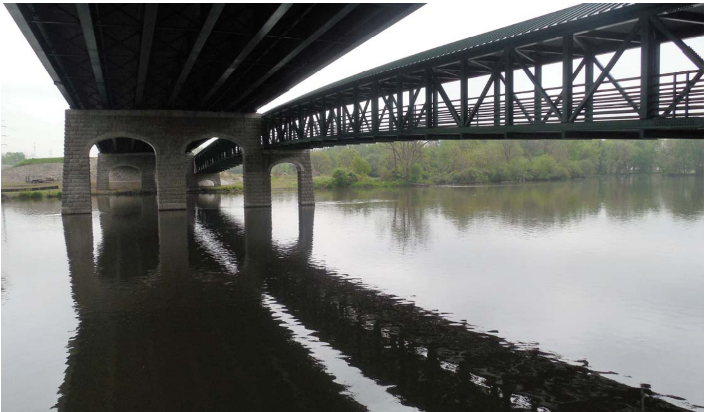
Photo 24 - Pedestrian Bridge Looking East From Pier 2
