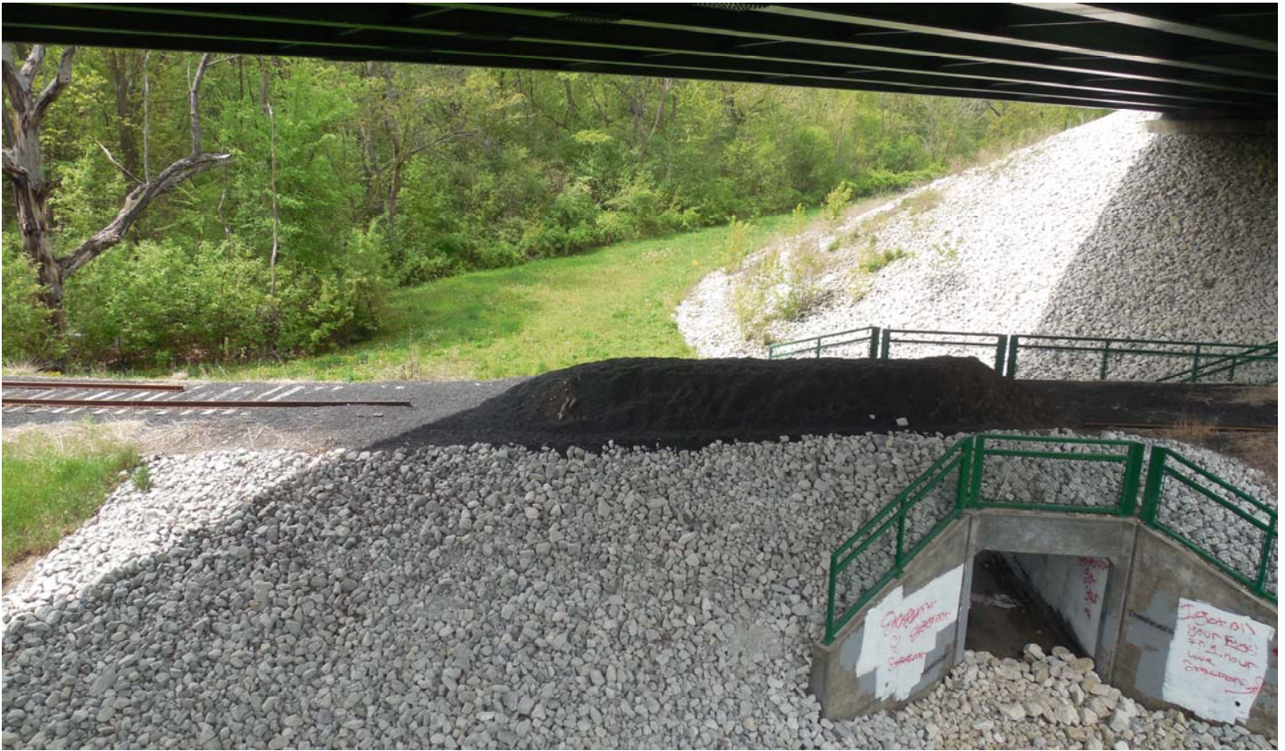
Photo 37 - Railroad Construction in Progress Under Span 1 Looking Southwest
