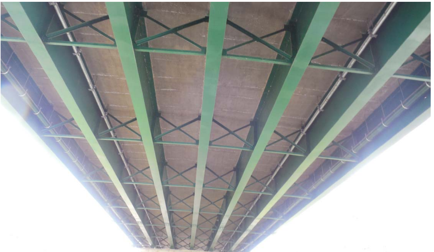
Photo 26 - Underside of Deck in Span 2
