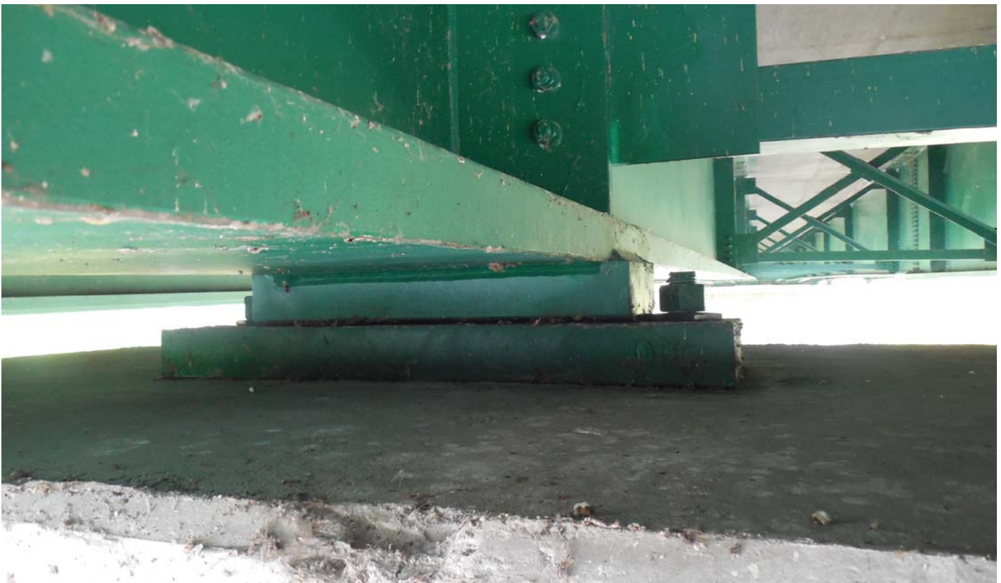
Photo 20 - Bearing at Pier 2 Beam 4
