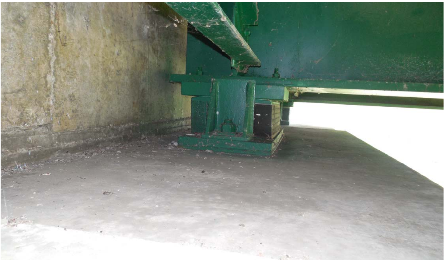
Photo 46 - Bearing at the West Abutment
