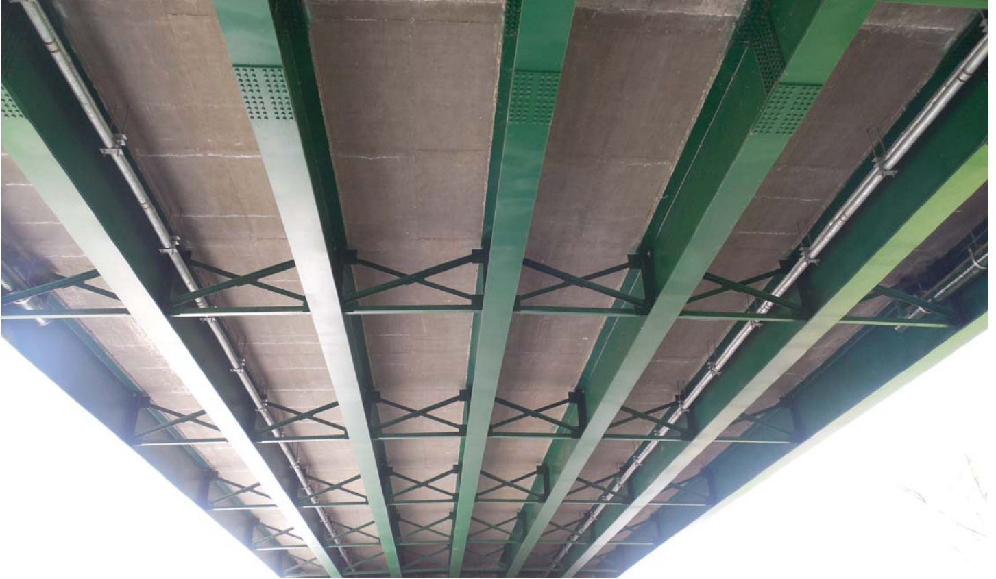
Photo 39 - Underside of Span 1 from Pier 1
