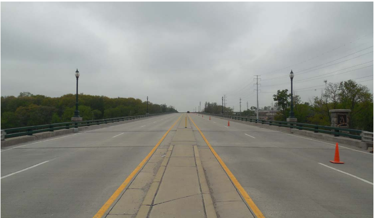
Photo 66 - Looking West Across Bridge From East Approach
