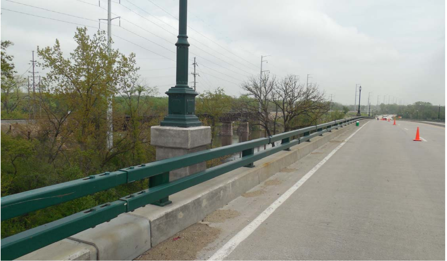
Photo 55 - Light Pole - North Rail near West Abutment Looking Northeast
