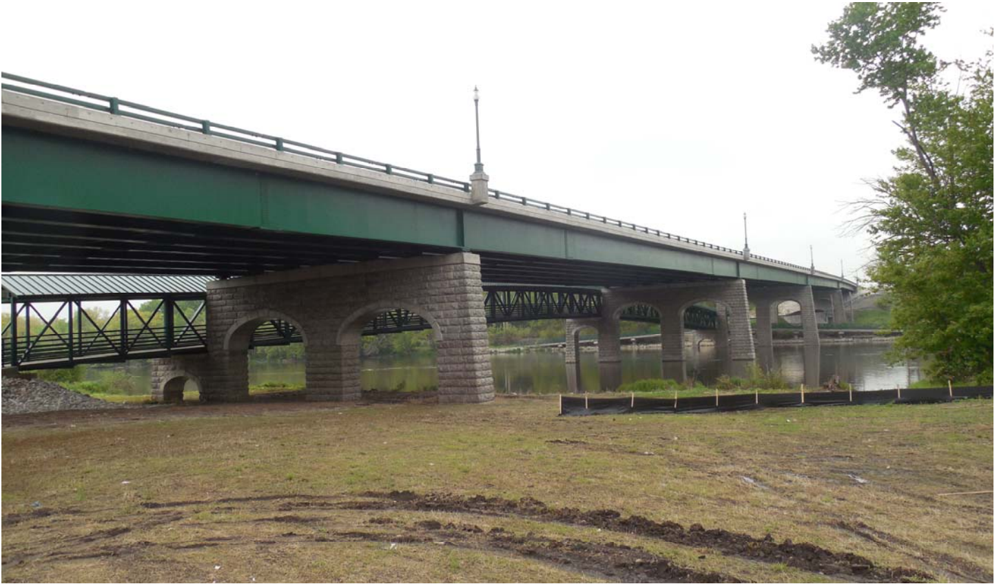
Photo 67 - North Elevation Looking Southwest
