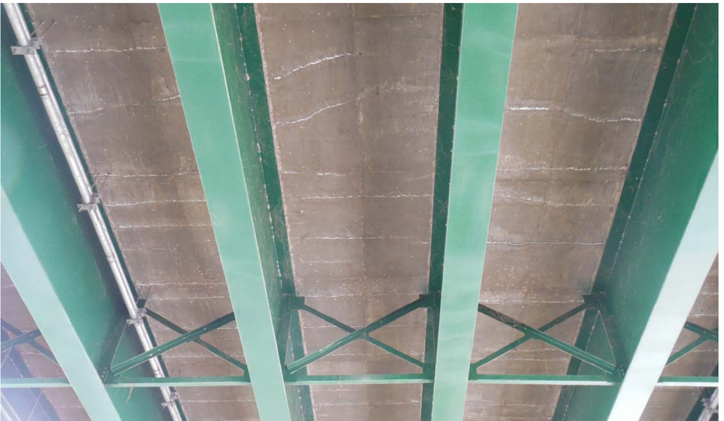
Photo 18 - Underside of Deck in Span 3
