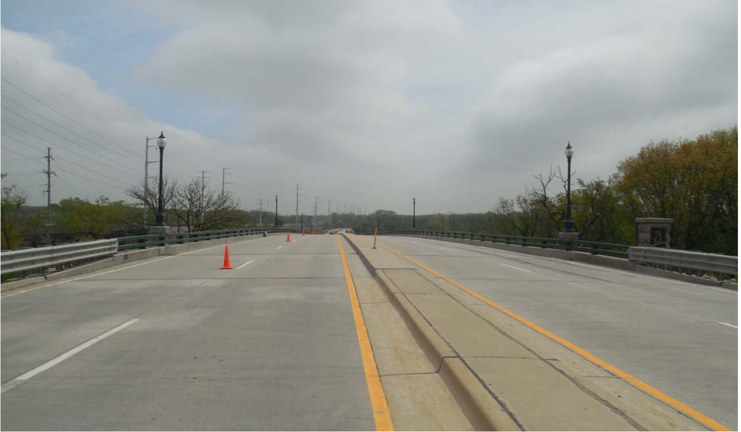
Photo 49 - Looking East Across Bridge
