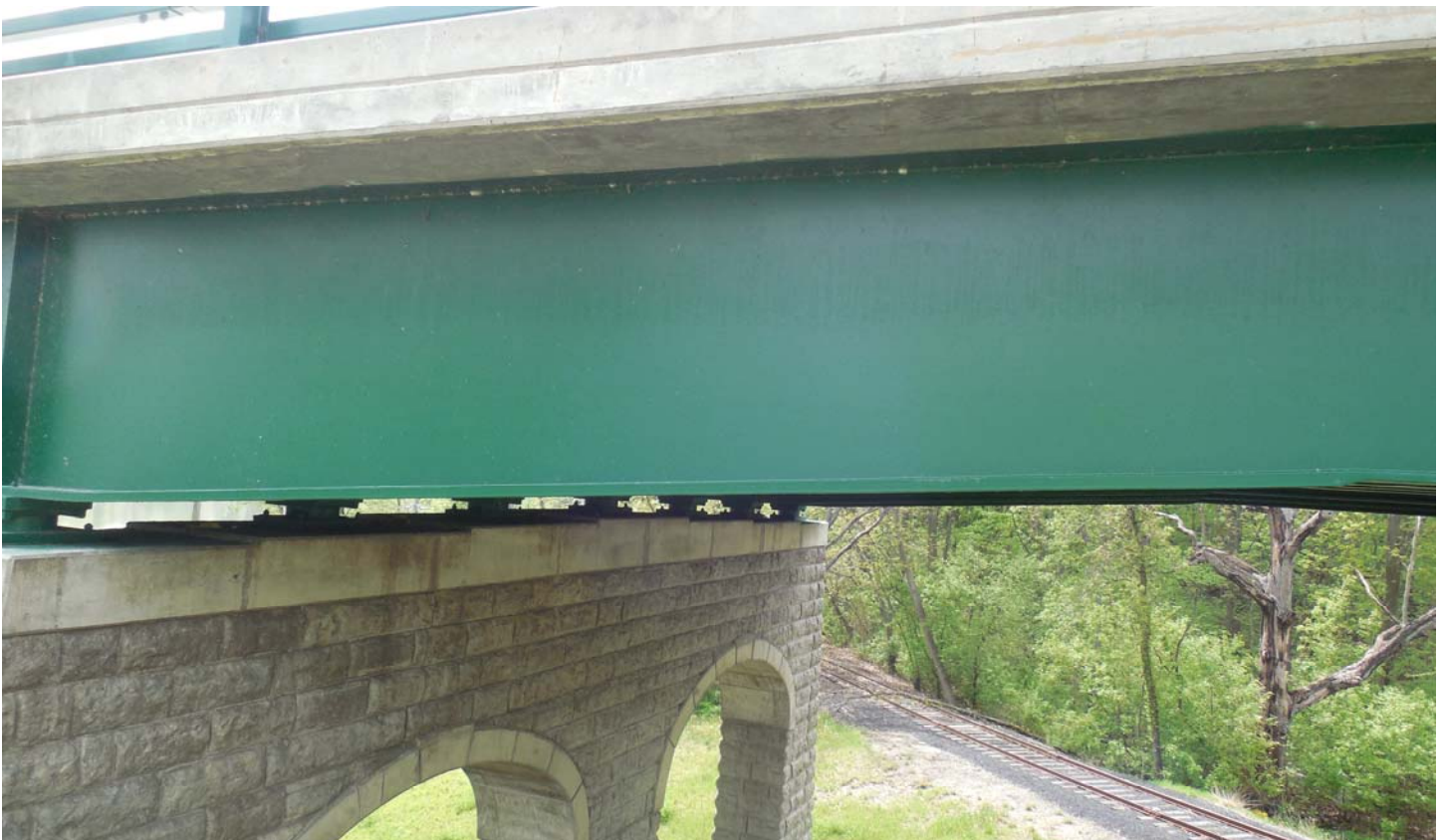
Photo 36 - North Fascia - Span 1
