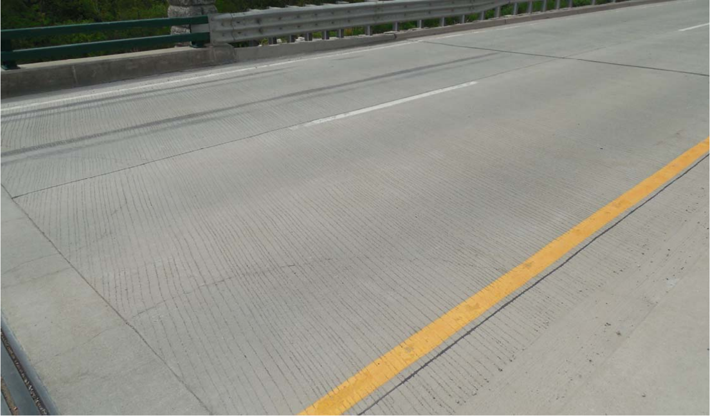
Photo 51 - West Approach - Eastbound Lanes
