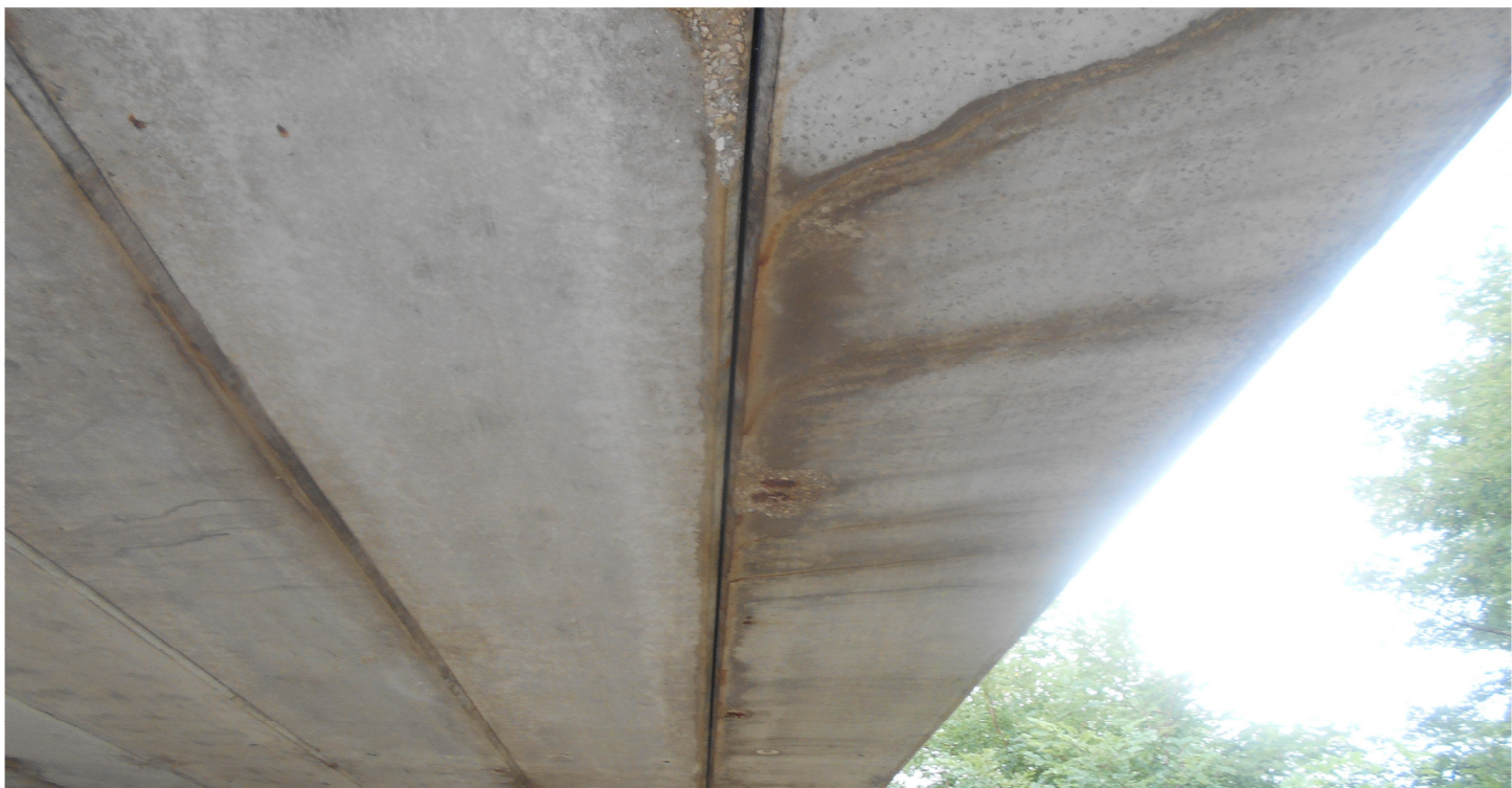
Photo 12 - Moderate Keyway Joint Leakage along Beams 10 & 11 - Span 3
