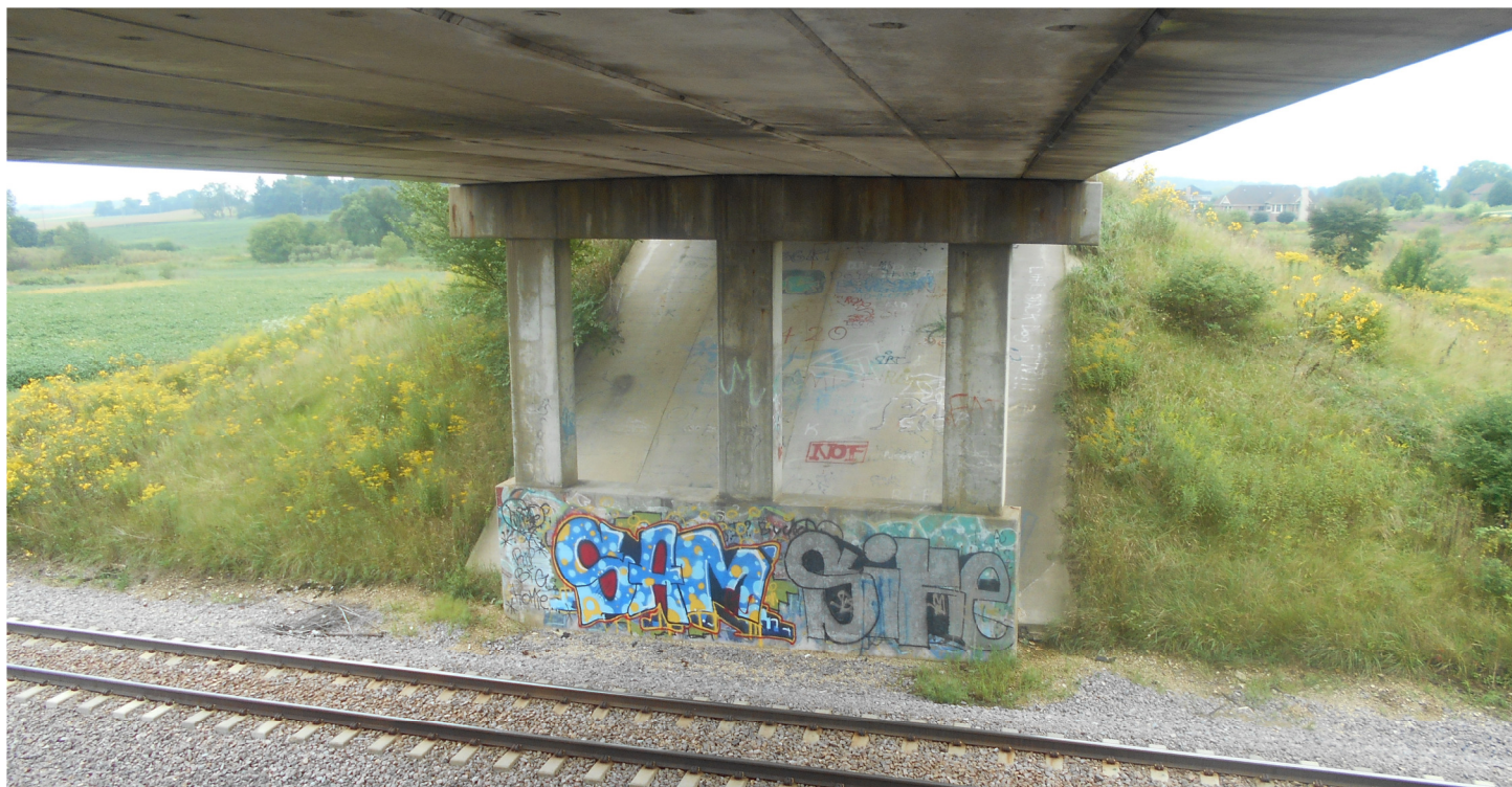
Photo 9 - North Face of the South Pier
