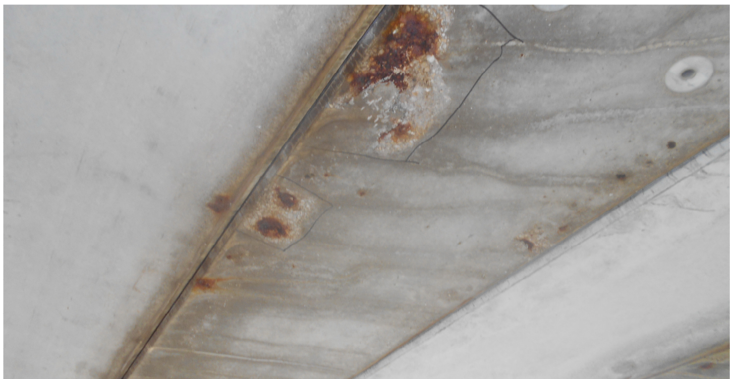
Photo 6 - 2' x 1' Spall with an Exposed Shear Stirrup near Midspan - Beam 9, Span 1
