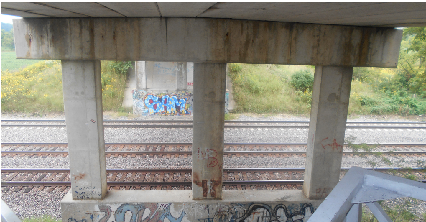
Photo 14 - North Face of the North Pier
