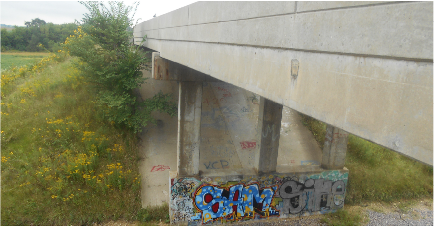
Photo 17 - Looking South down East Fascia
