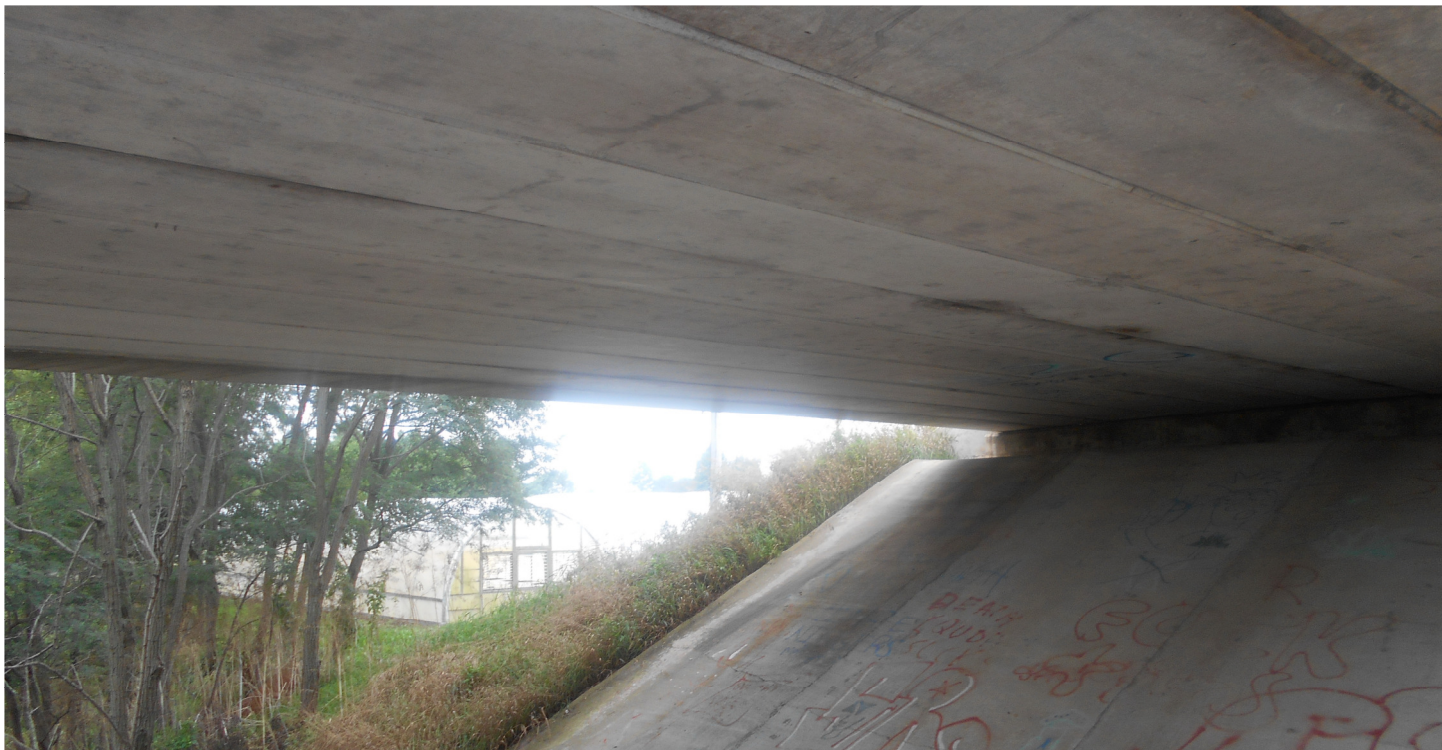
Photo 13 - Underside of Beams Looking Northwest - Span 3
