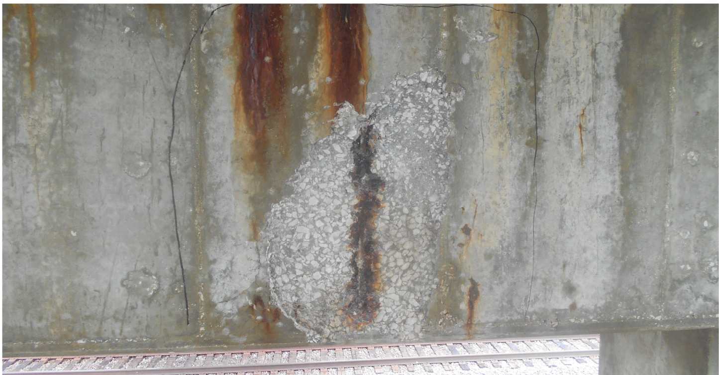
Photo 8 - 2.5' x 3' x 1.5' Deep Spall with an Exposed Shear Stirrup - South Face of South Pier
