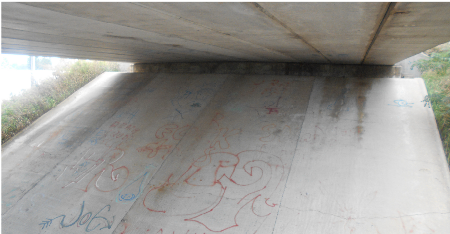
Photo 11 - North Span and Abutment
