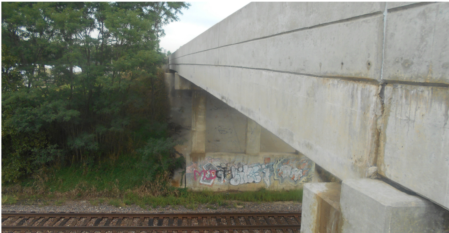
Photo 1 - Looking North down West Fascia
