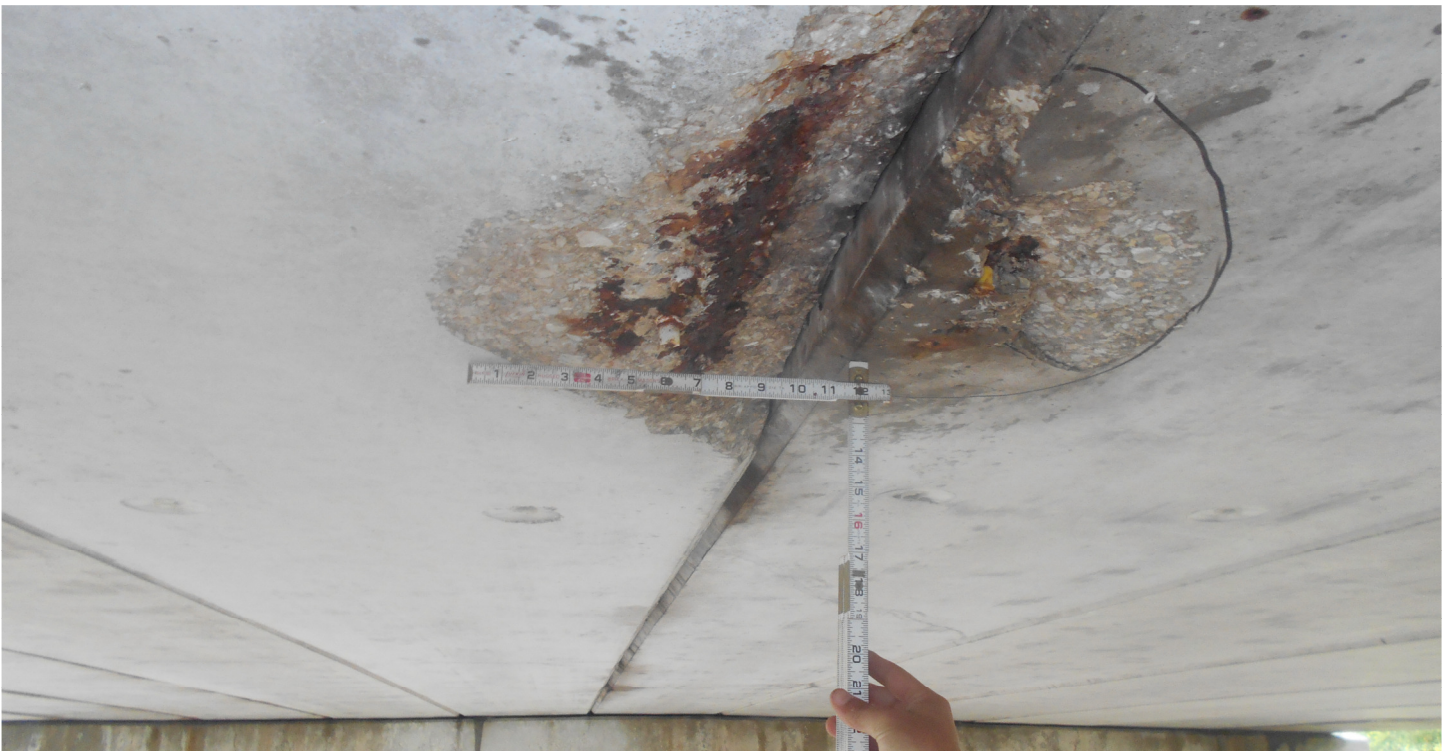
Photo 16 - Previously Mentioned Spall - Beam 7, Span 3
