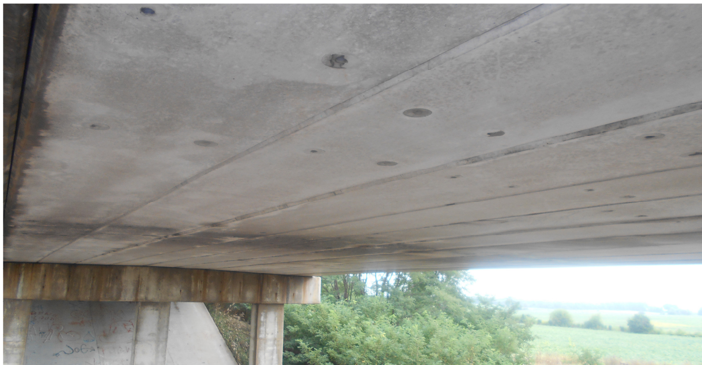
Photo 5 - Underside of Beams Looking Northeast - Span 2
