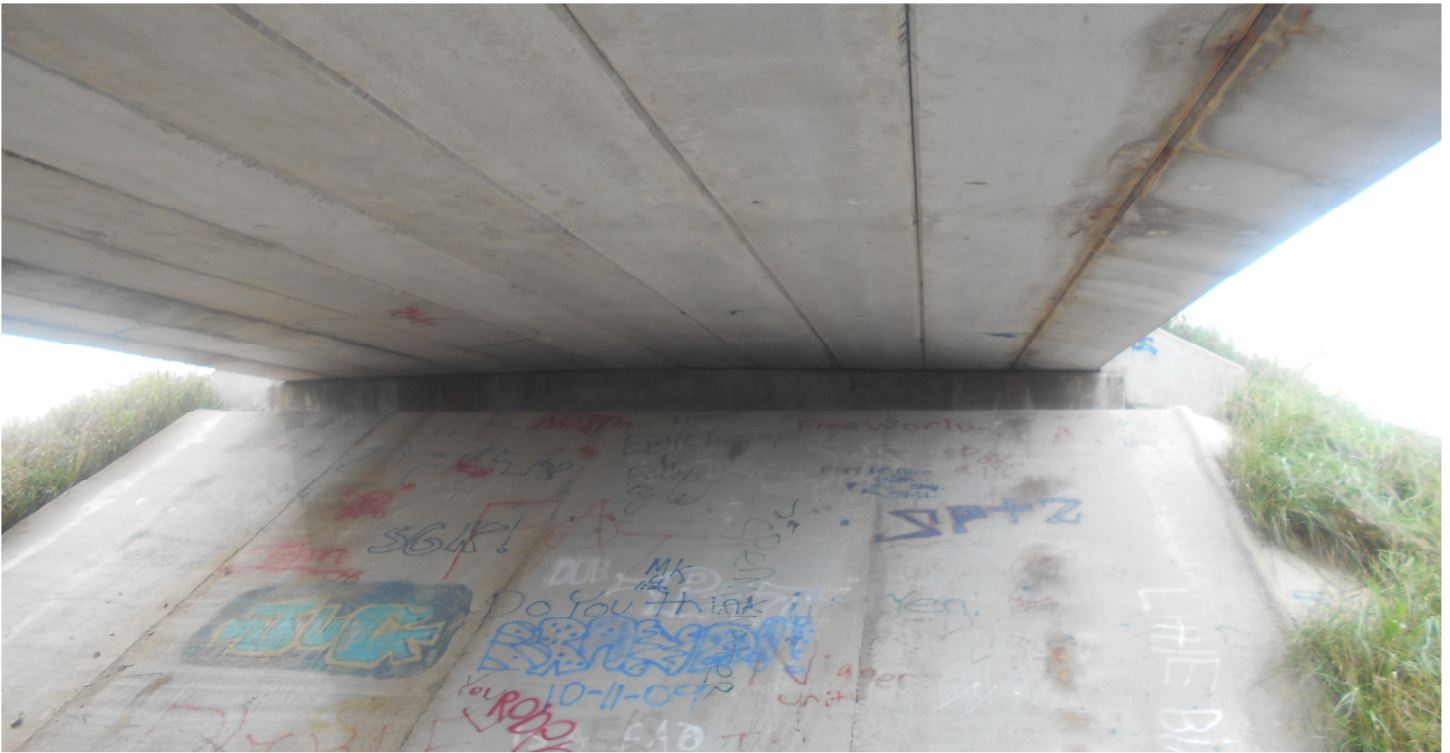
Photo 3 - South Span and Abutment
