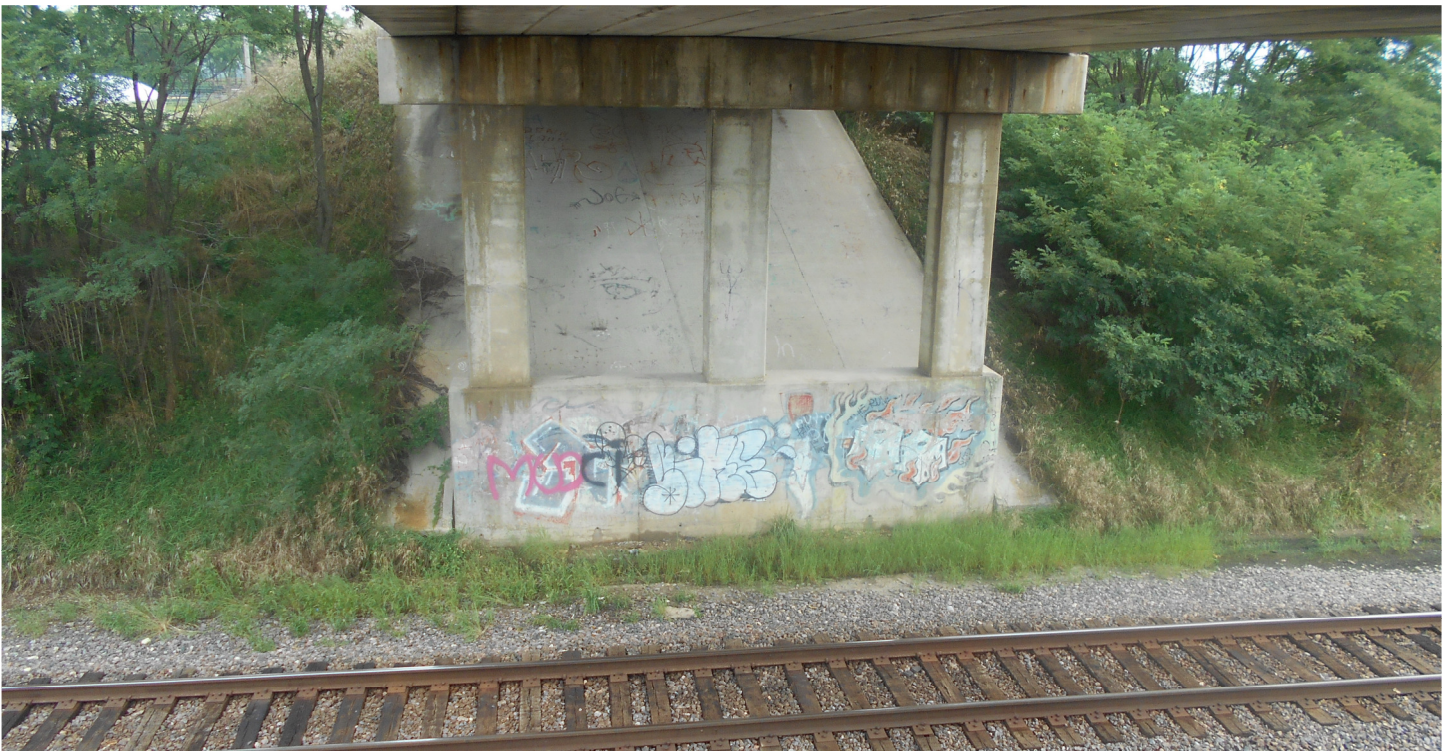
Photo 4 - South Face of the North Pier
