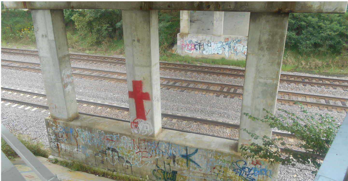
Photo 7 - South Face of the South Pier
