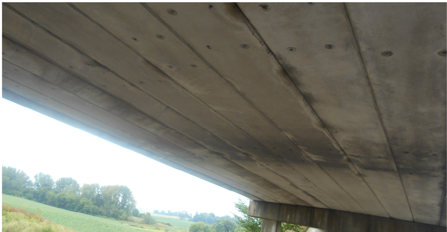
Photo 10 - Underside of Beams Looking Southeast - Span 2
