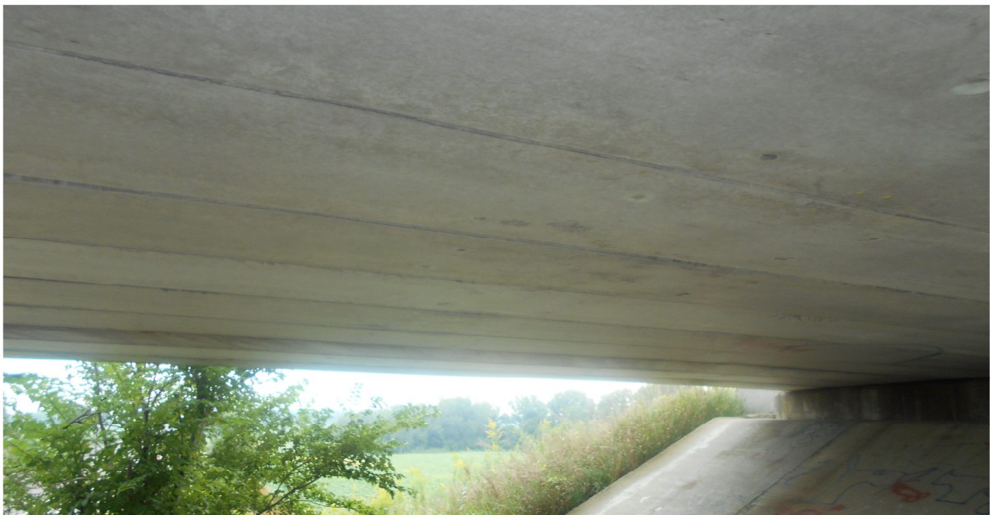
Photo 2 - Underside of Beams Looking Southeast - Span 1
