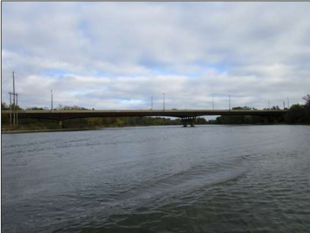
Photo No. 2 South Elevation, looking North
