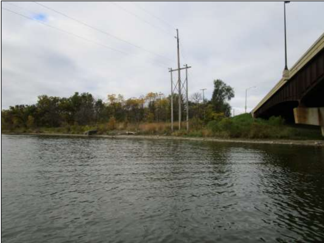
Photo No. 6 West Shoreline Downstream of Bridge, looking Southwest
