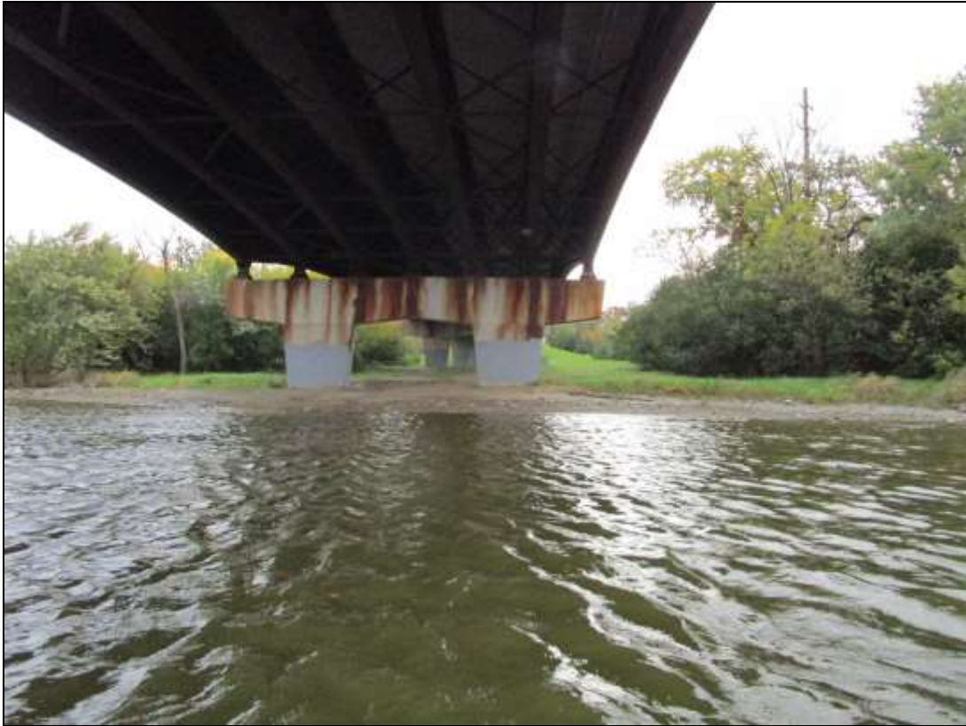
Photo No. 9 Pier 4 Elevation (West Face Shown), looking East
