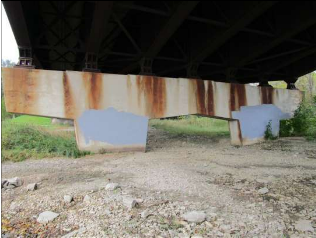
Photo No. 7 Pier 1 Elevation (East Elevation Shown), looking West
