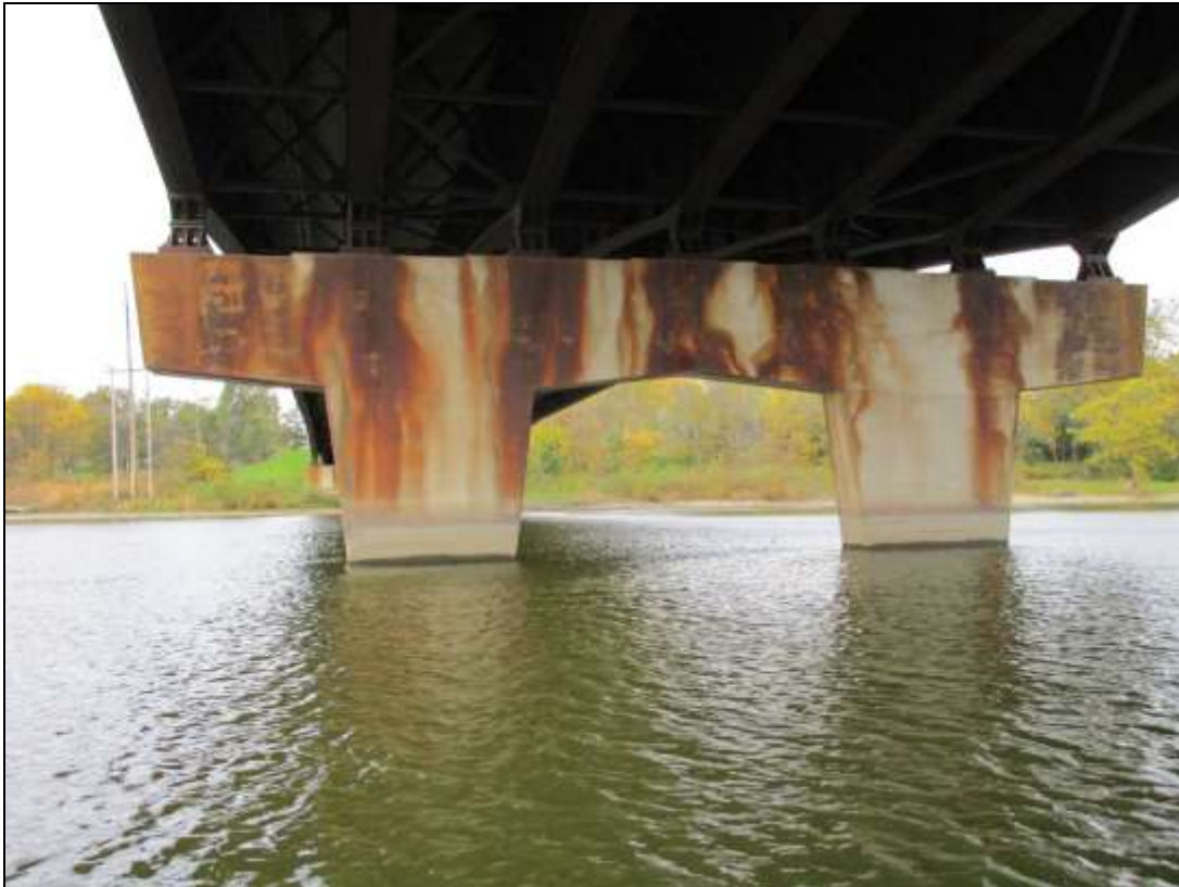
Photo No. 8 Pier 2 Elevation (East Face Shown), looking West
