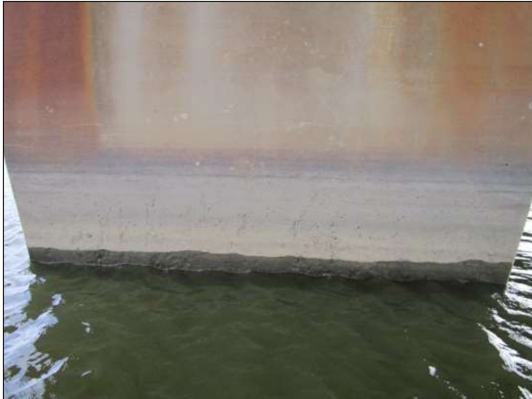
Photo No. 10 South Pier Shaft of Pier 2 Scaling (West Face Shown), looking East
