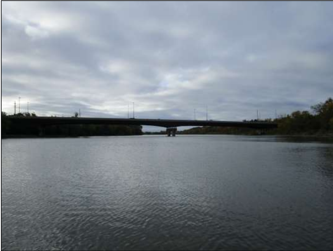
Photo No. 1 North Elevation, looking South
