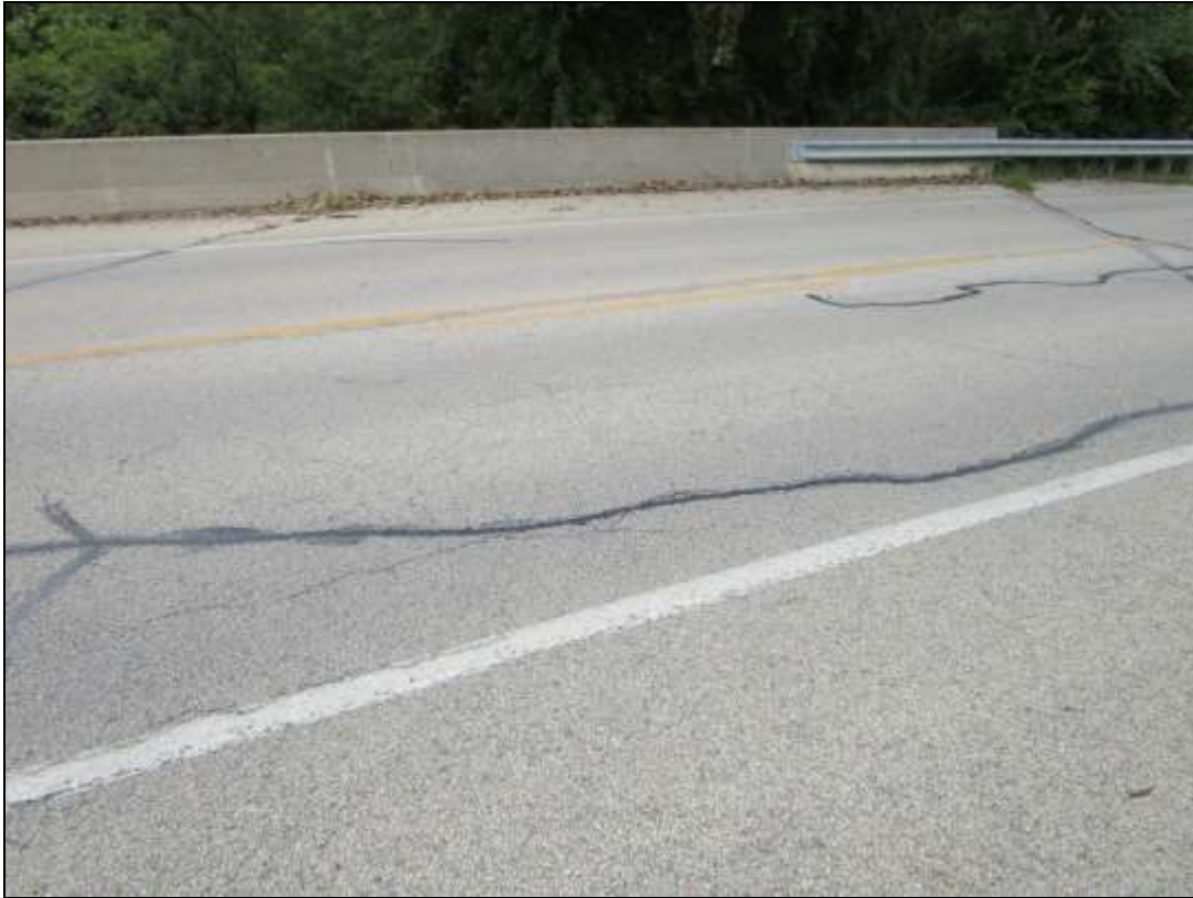
Photo No. 11 Top of Deck (North Span), looking West
