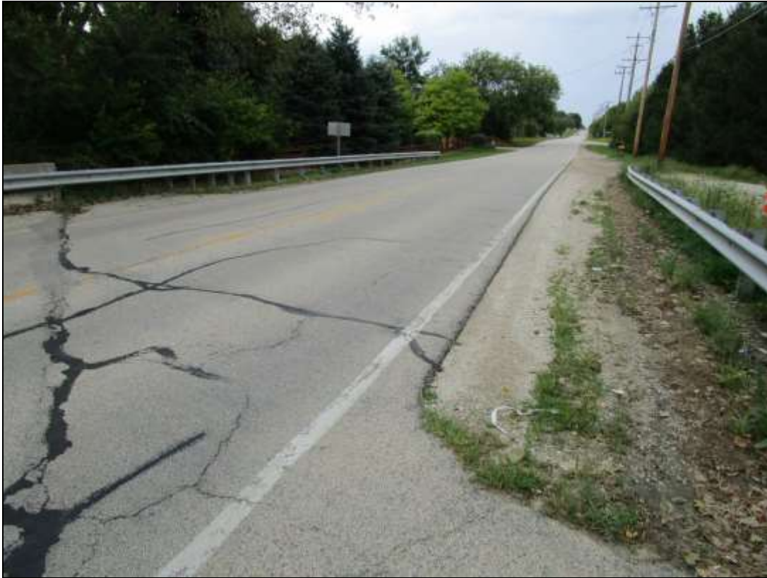
Photo No. 5 North Approach Roadway, looking Northwest
