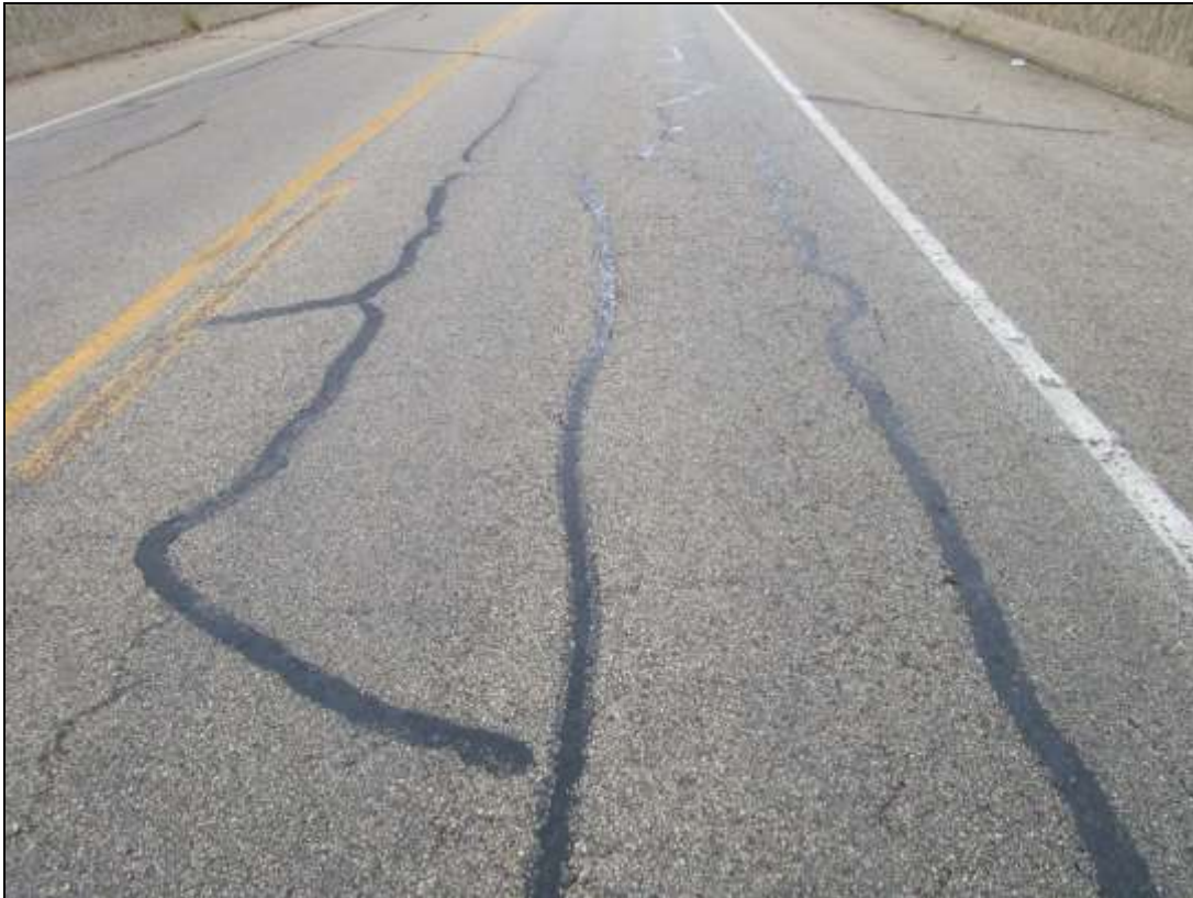
Photo No. 12 Typical Condition of Deck Overlay, looking North
