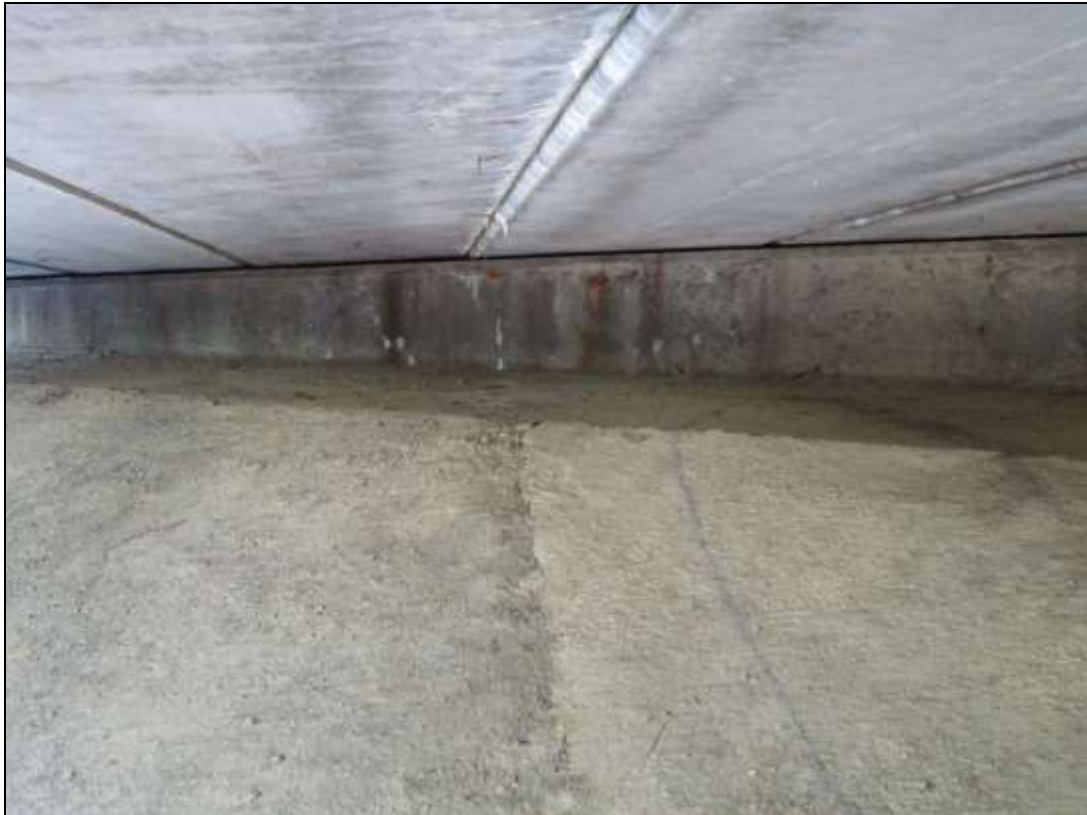
Photo No. 22 Rust Staining and Efflorescence on South Abutment, looking South
