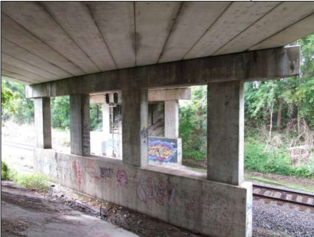
Photo No. 25 Pier 3, looking South
