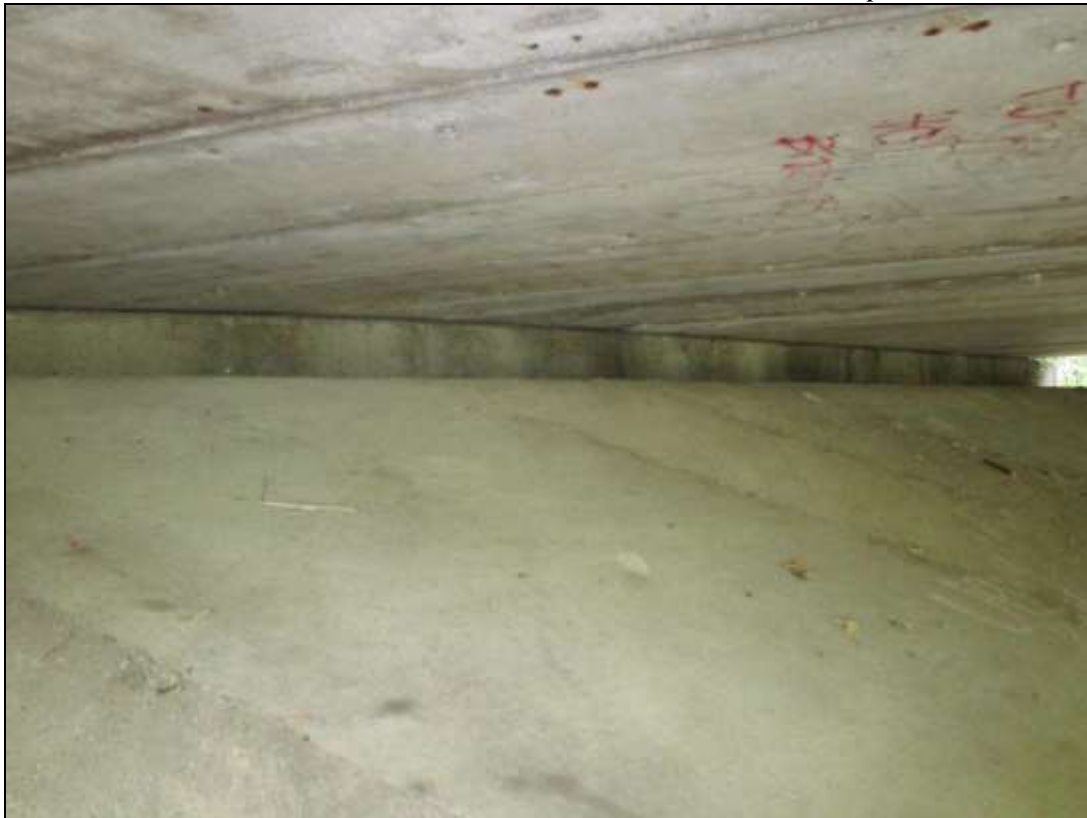
Photo No. 21 North Abutment, looking Northwest
