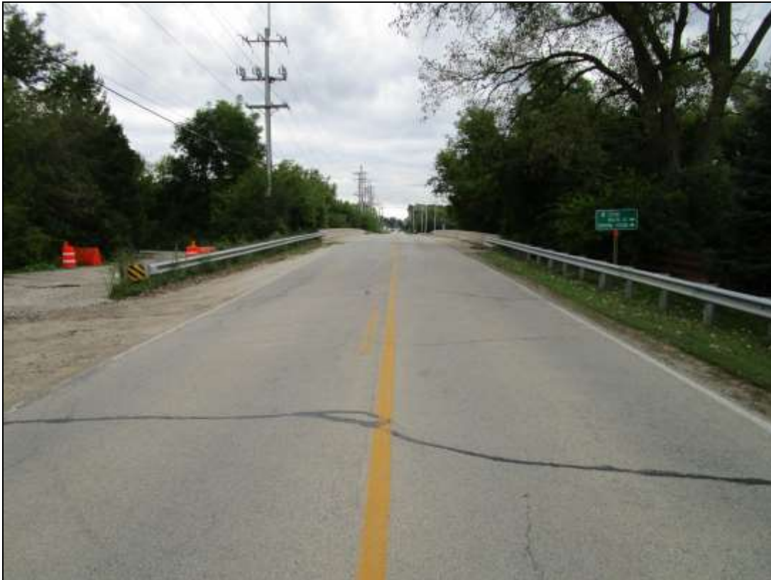
Photo No. 4 Topside of Structure, looking South
