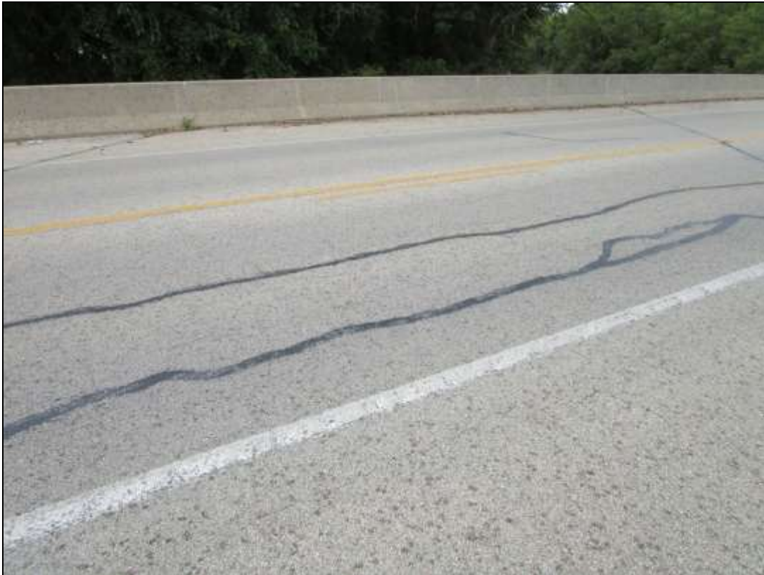
Photo No. 10 Typical Top of Deck Center Span Condition (Span 2 Shown), looking West
