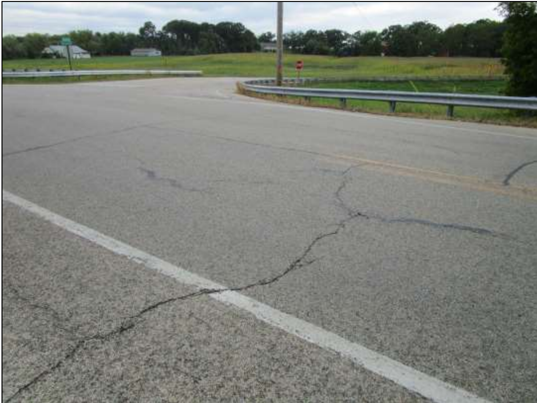
Photo No. 6 South Approach Roadway, looking Southwest
