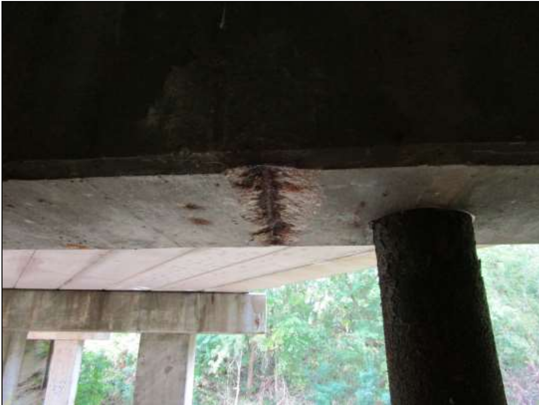
Photo No. 30 Spall at Pier 4, 3 rd Pile from East, looking South
