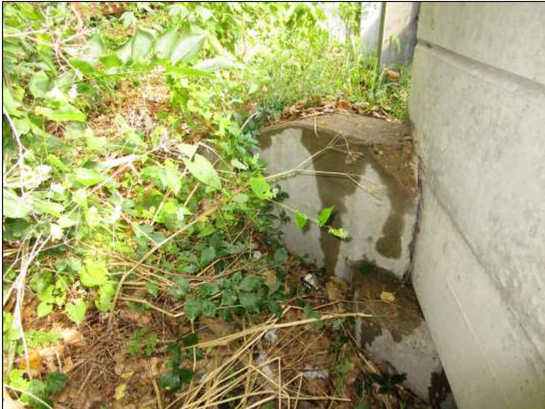
Photo No. 32 Spall at Northwest Wing Wall, looking North
