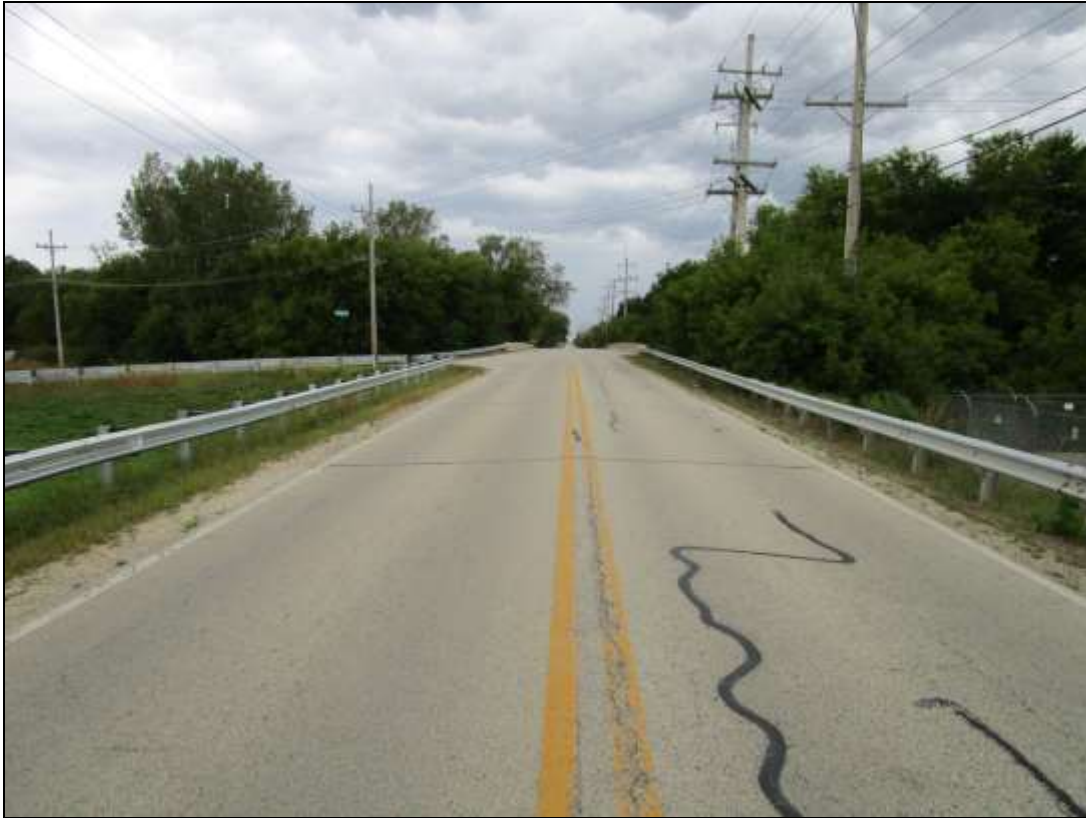
Photo No. 3 Topside of Structure, looking North
