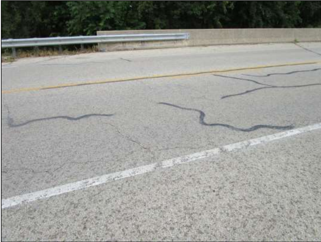
Photo No. 9 Top of Deck (South Span), looking West
