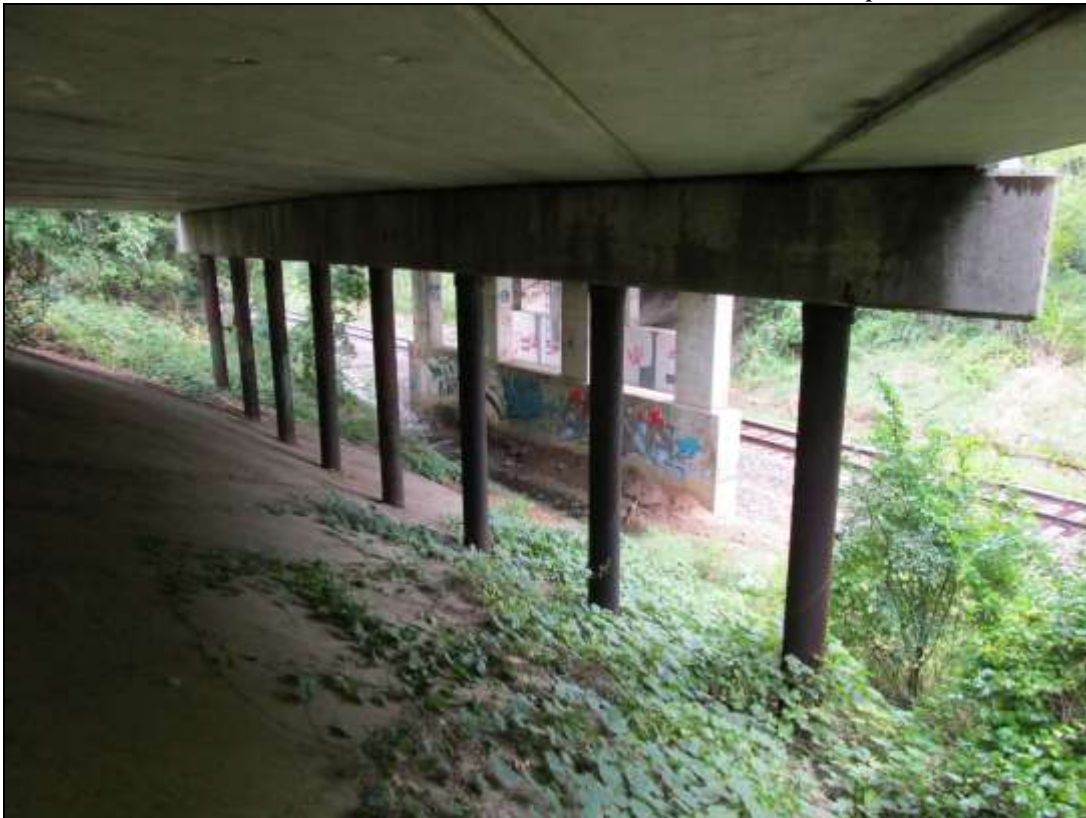
Photo No. 23 Pier 1, looking Northwest
