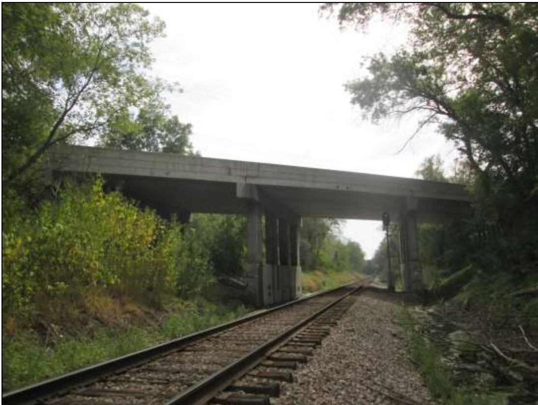
Photo No. 2 West Elevation, looking East
