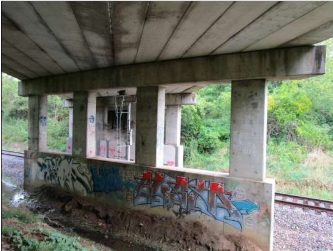
Photo No. 24 Pier 2, looking North
