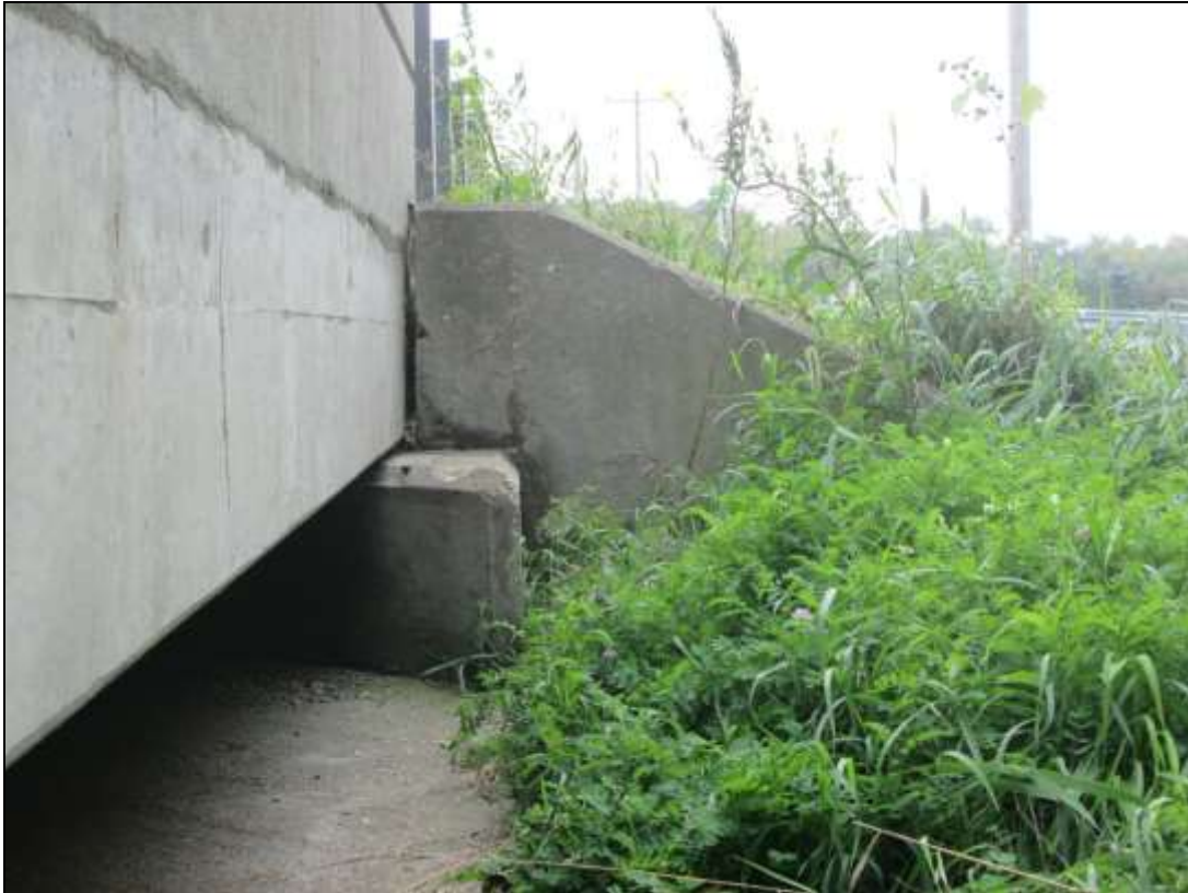
Photo No. 31 Typical Wingwall (Southwest shown), looking South
