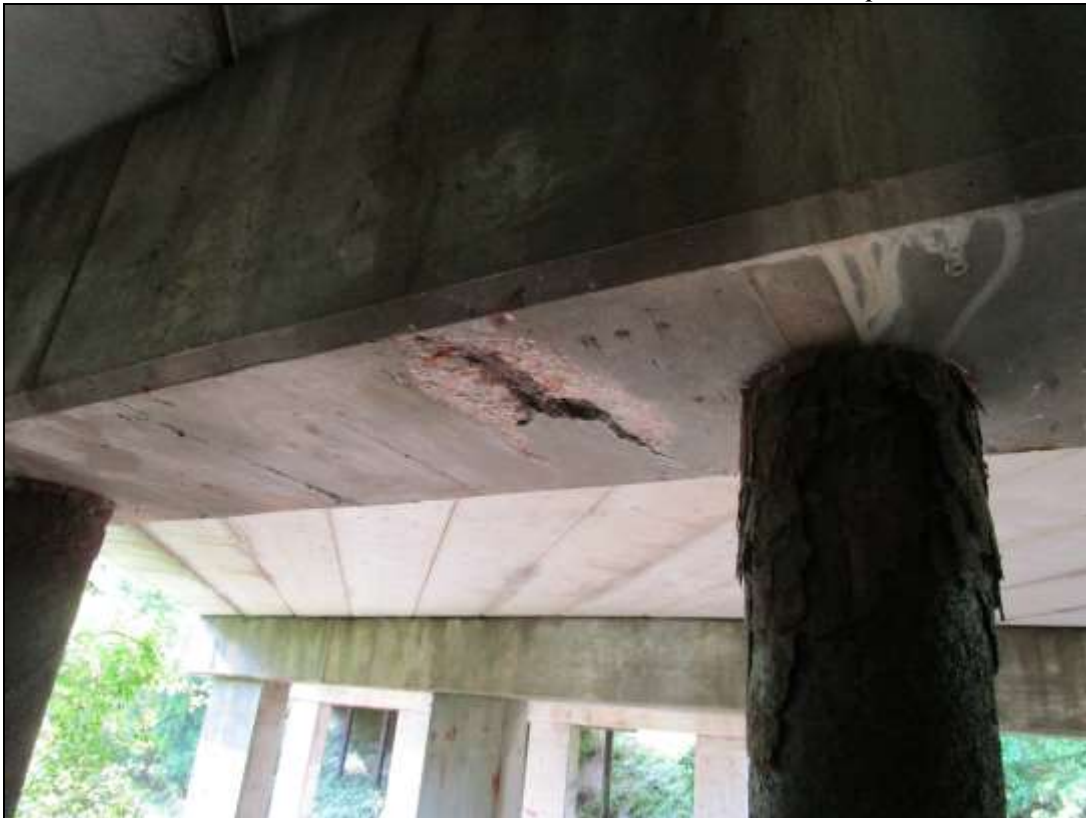
Photo No. 29 Spall at Pier 4, 6 th Pile from East, looking South
