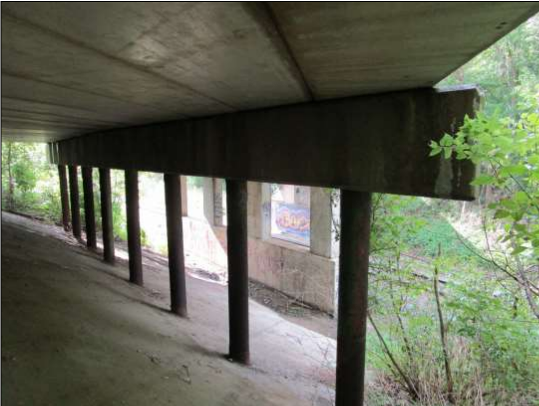
Photo No. 26 Pier 4, looking Southeast
